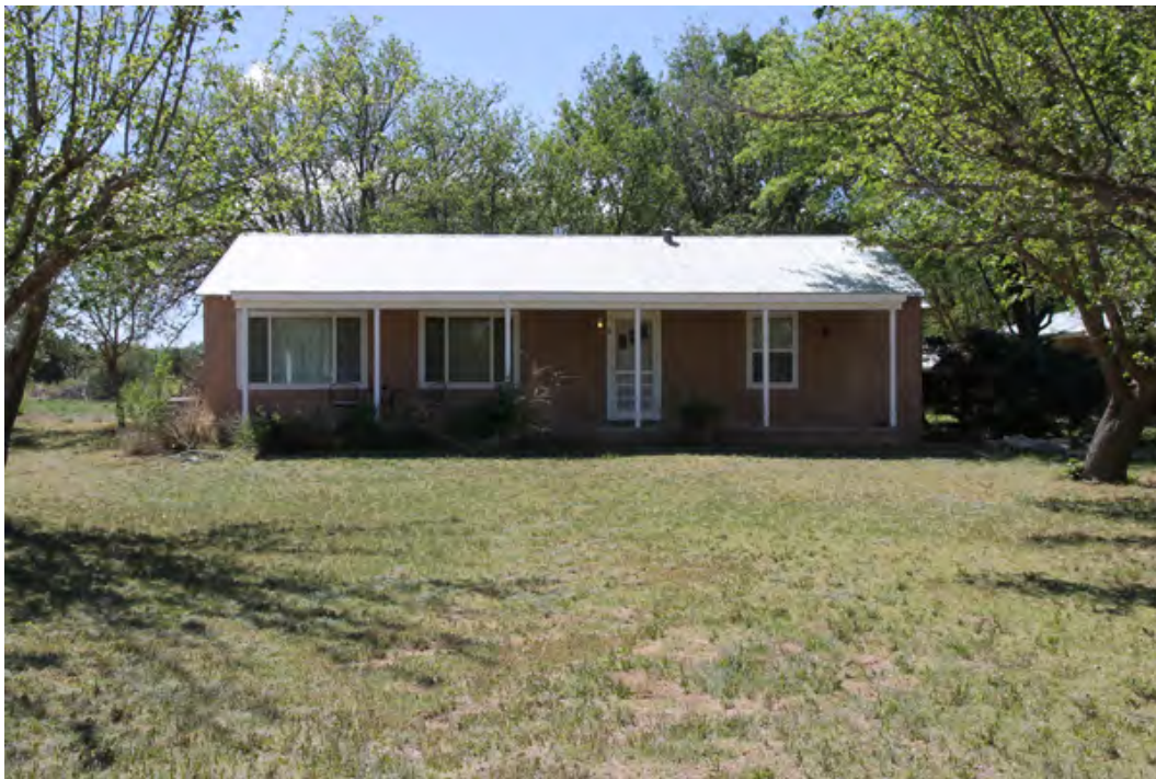
22 of 26. House A, photographer facing north.
