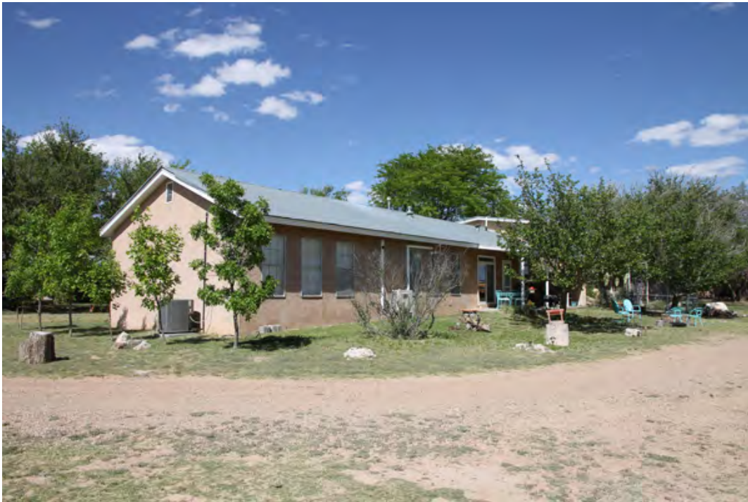
17 of 26. Studio E, photographer facing northeast.
