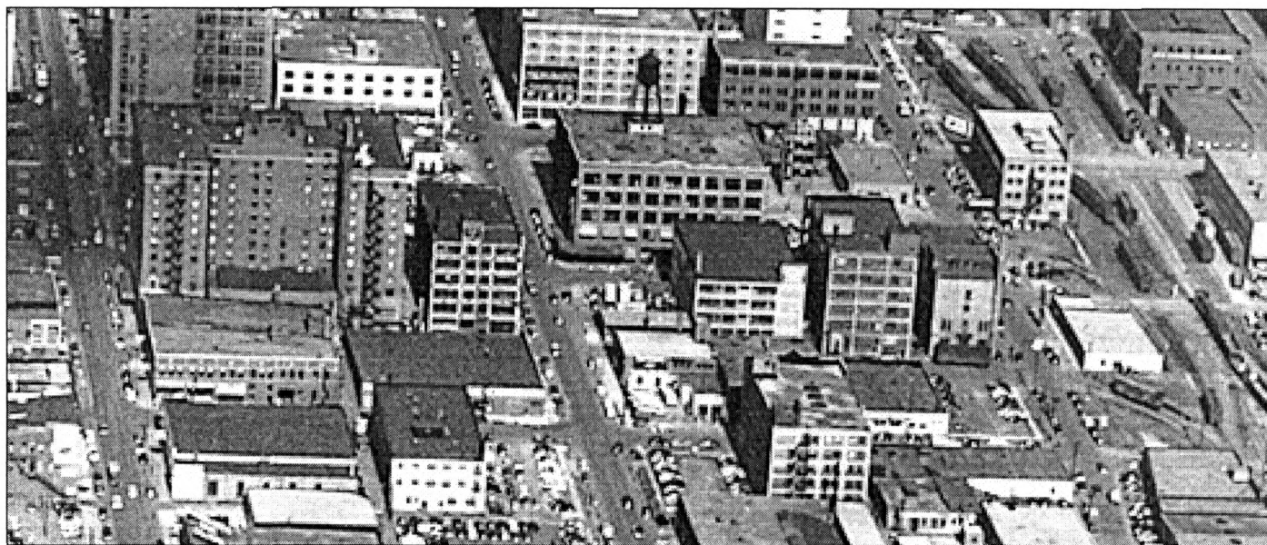
Figure 39: 1941 aerial view of the west edge of the main downtown The Clemens Building is immediately left of center, to the right of the Hotel Fort Des Moines, the massive tall building at the left side (Plan and Zoning Department, City of Des Moines)
