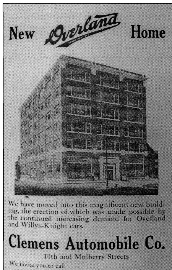
Figure 35: The newly occupied building, view northwest ( Des Moines Magazine , September 1916, p. 29)
