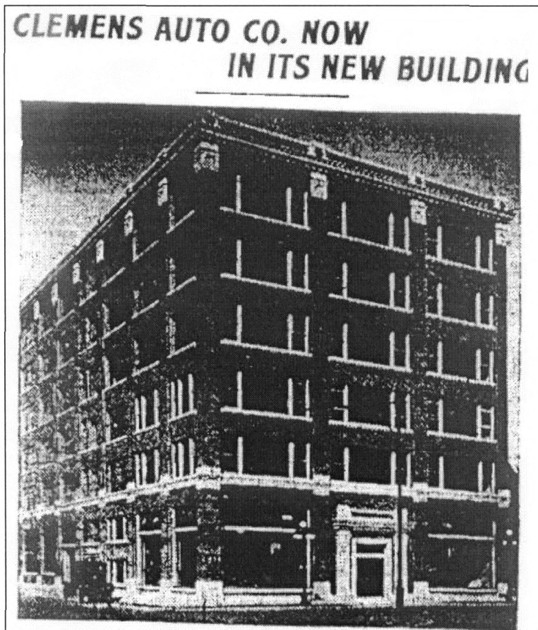
Figure 34: Completion photo, view northwest (Des Moines Capital , September 1, 1916)
