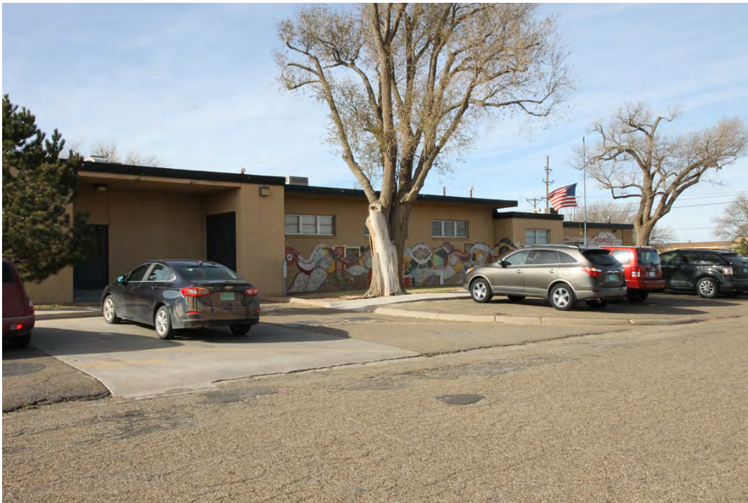
5 of 21. 1965 addition, photographer facing northwest.
