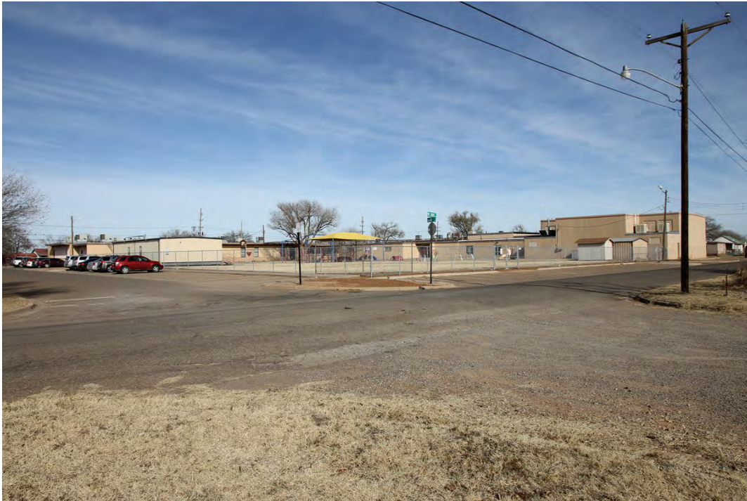
7 of 21. School complex, photographer facing northeast.
