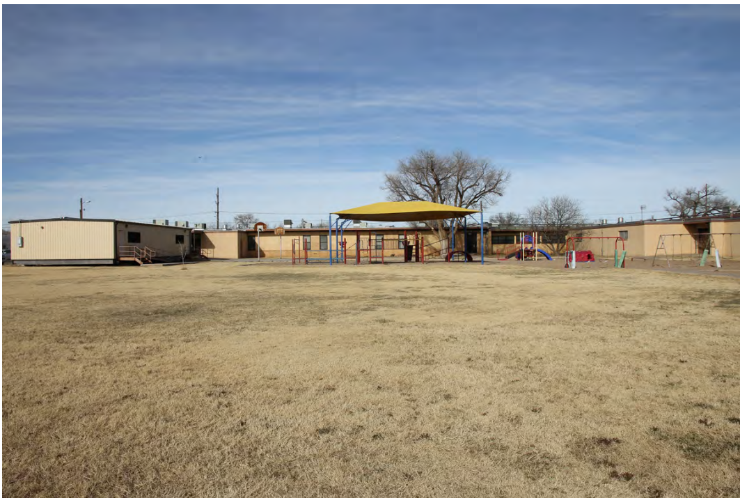
8 of 21. School complex photographer facing north.
