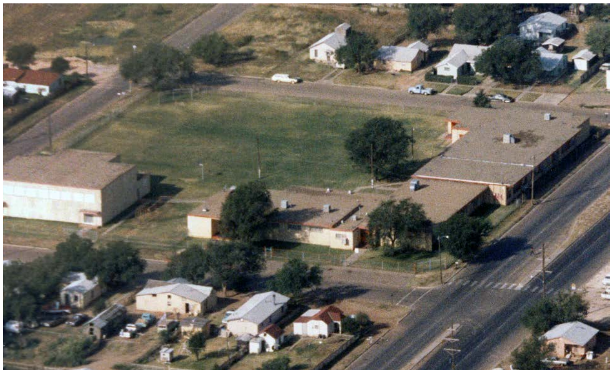
Figure 2. Lincoln Jackson School, c.1965. View toward southwest.
