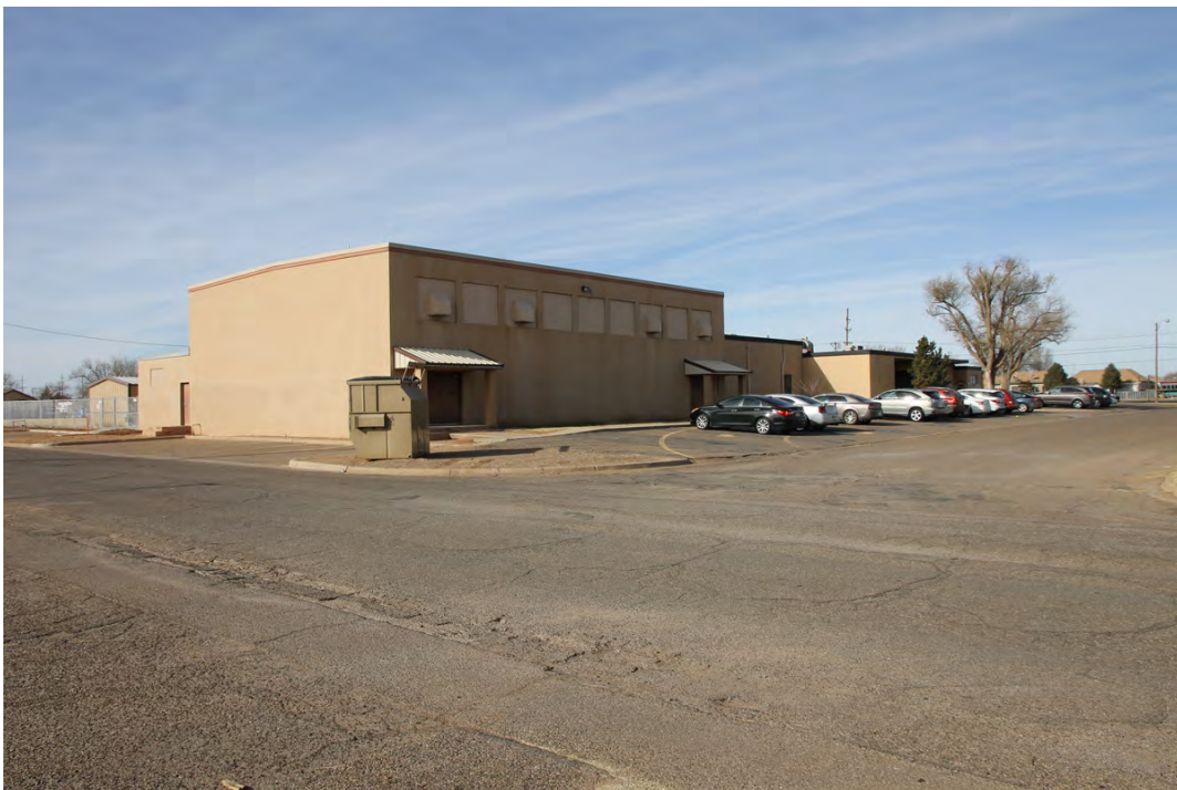
6 of 21. Gymnasium, photographer facing northwest.
