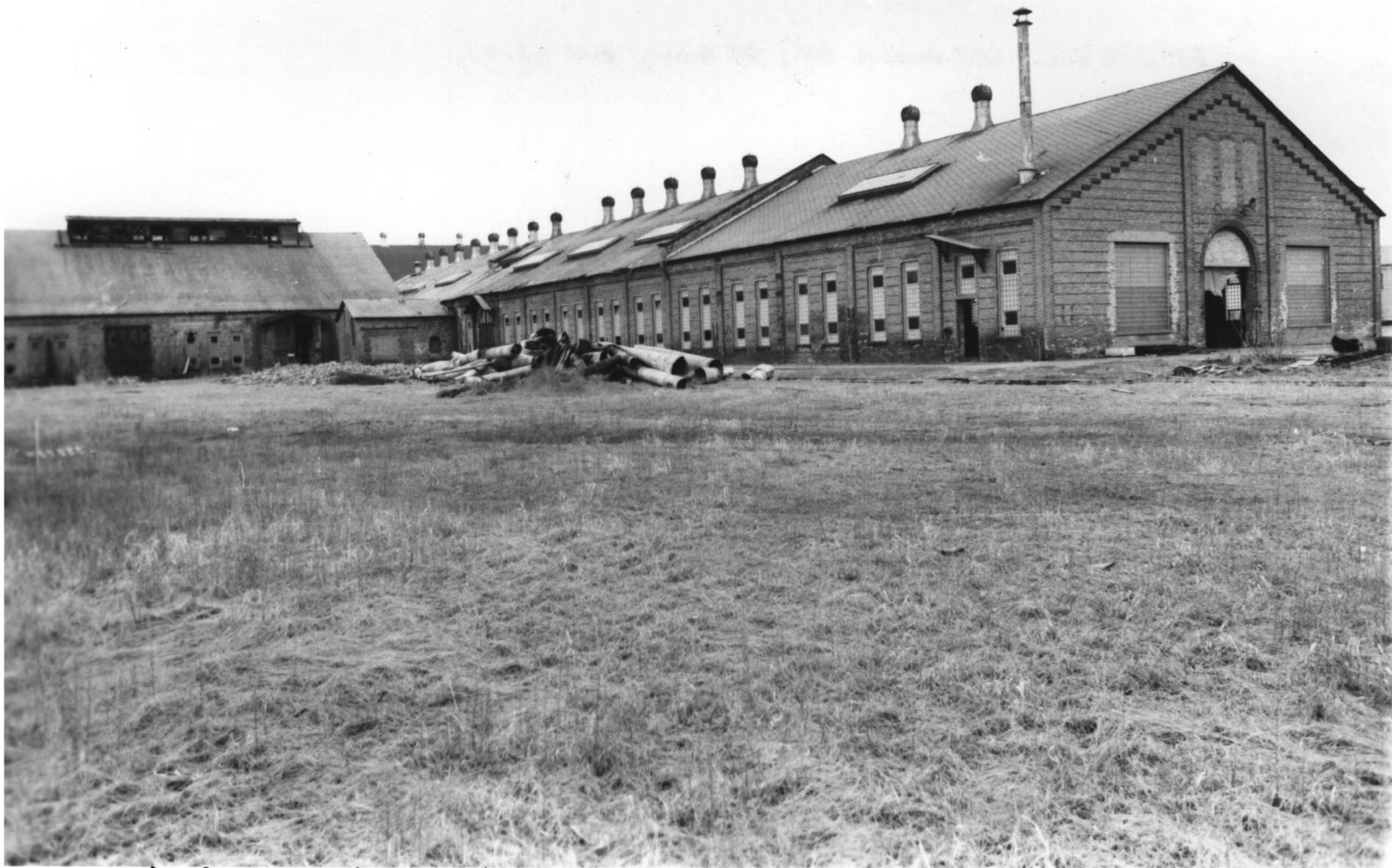
Northern Pacific Railroad Shops Historic District Blacksmith Shop #3 Crow Wing Co., MN 09979-15
