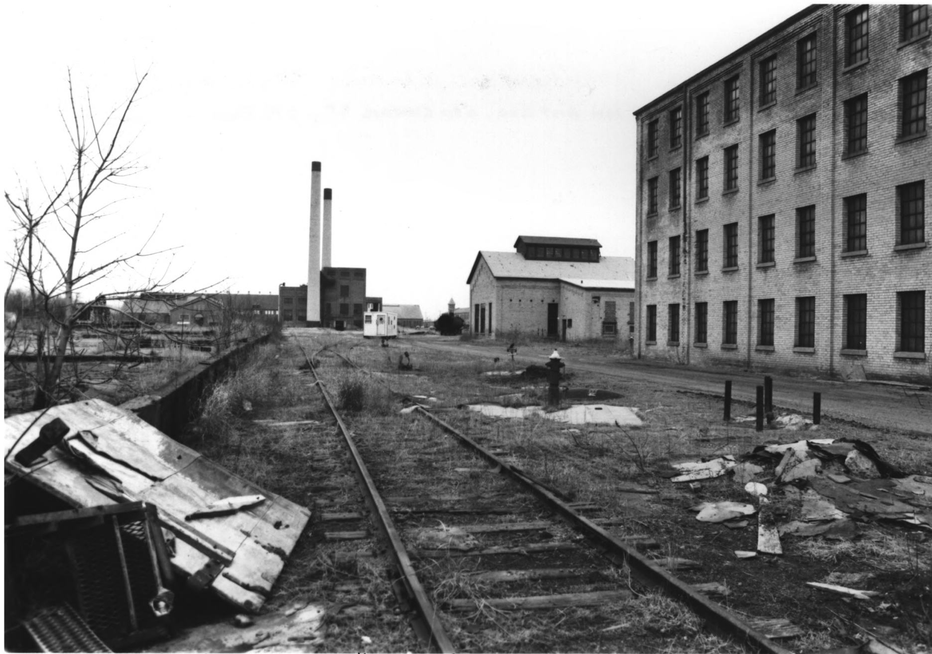
NORTHERN PACIFIC RAILROAD SHOPS HISTORIC DISTRICT GENERAL VIEW FROM BLDG 8 LOOKING WEST CROW WING CO, MN 09979-12
