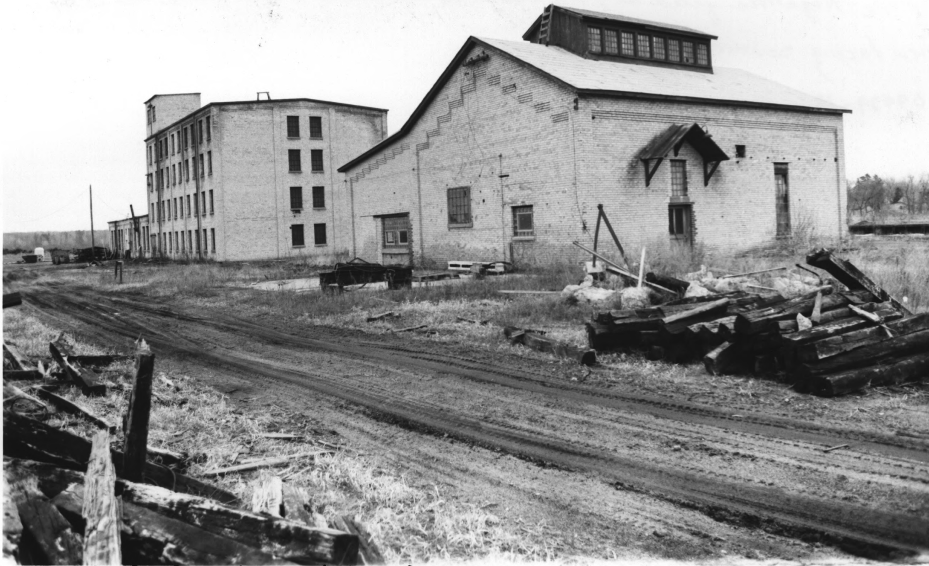
Northern Pacific Railroad Shops Historic District L: Pattern Shop - # 8; R: Foundry Boiler House - # 7 CROW WING CO., MN 09979-10
