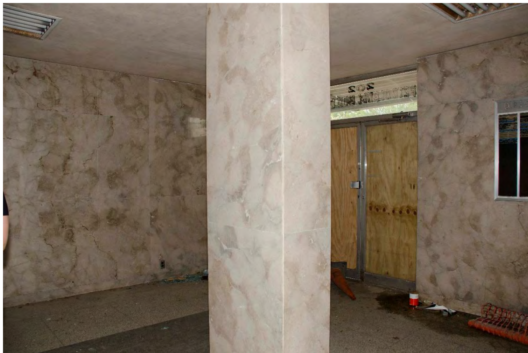
Photo 11: First floor interior. View northwest.
