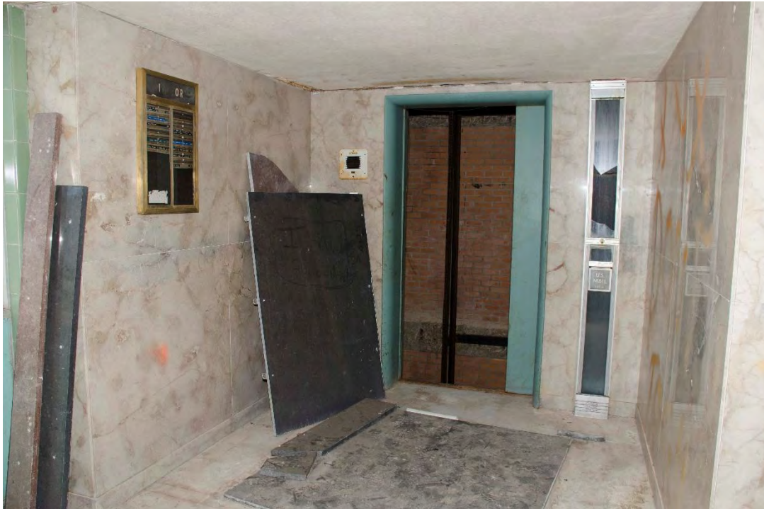
Photo 12: Third floor interior. View north.
