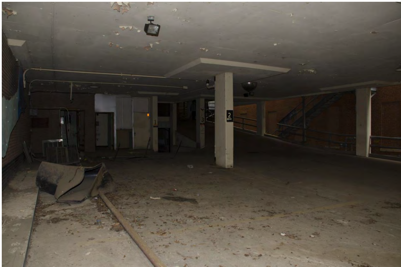
Photo 9: Parking garage ramp, first floor. View southeast.
