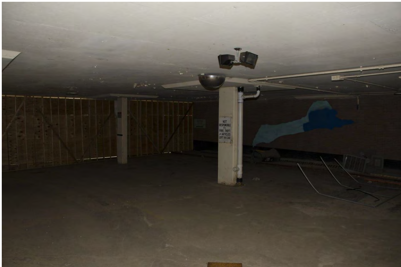
Photo 10: Parking garage interior, facing west automobile entrance. View northwest.
