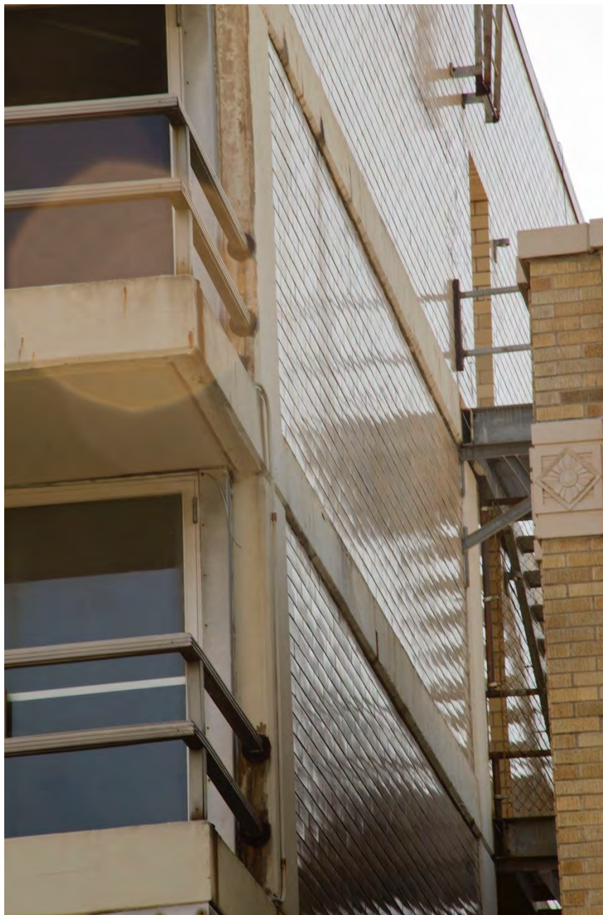
Photo 6: South Elevation. View east.
