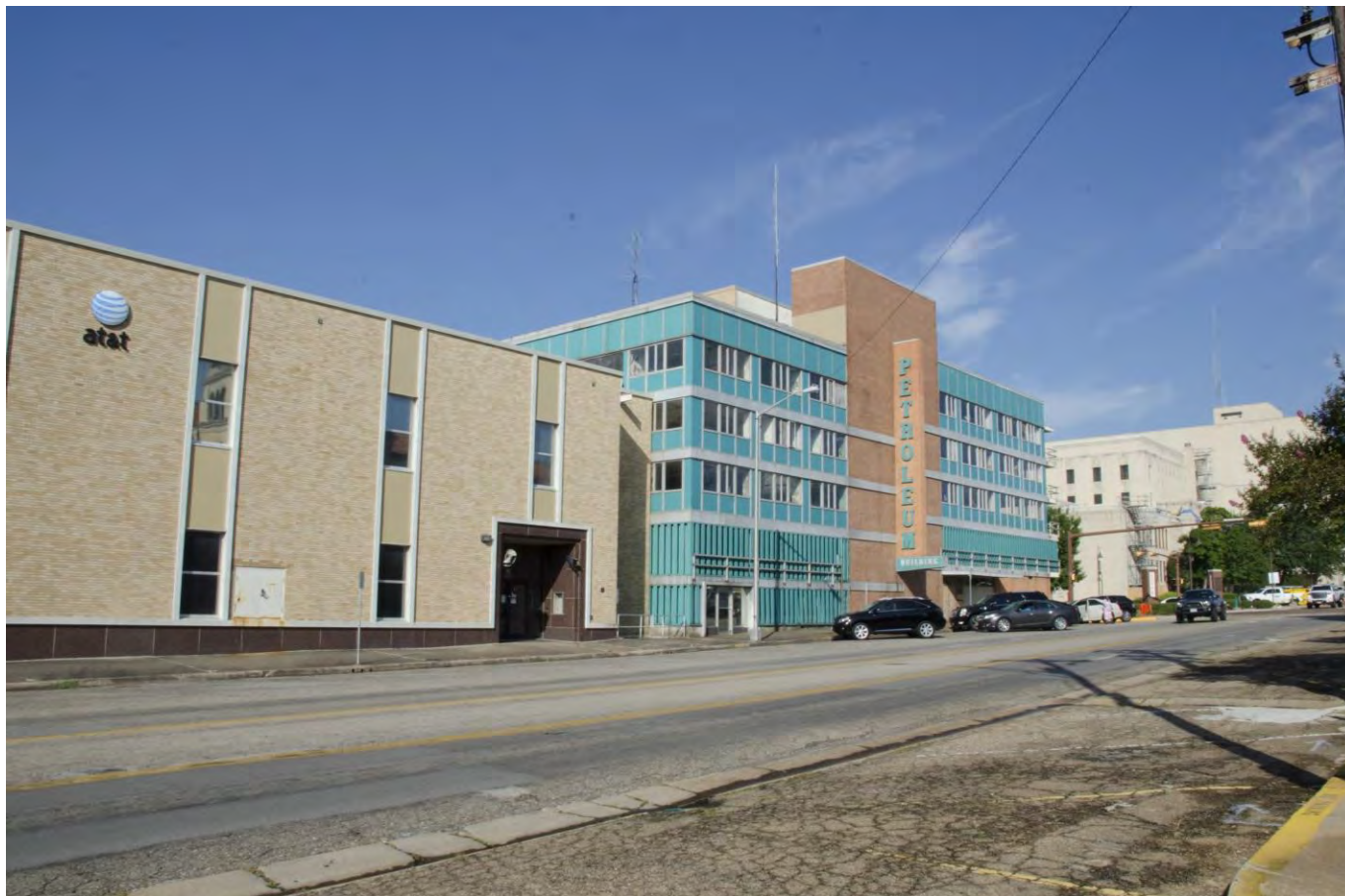
Photo 5: East and North (Primary) Elevations. View west.
