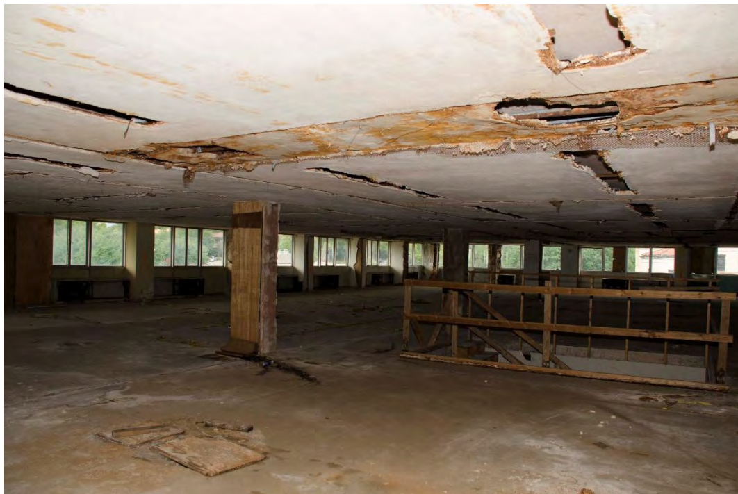
Photo 14: Fourth floor interior. View west.
