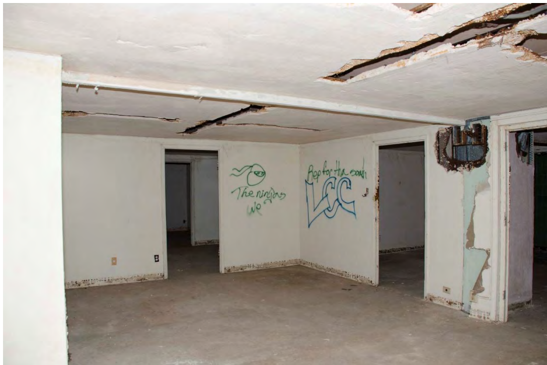
Photo 16: Fourth floor interior. Typical office. View south.
