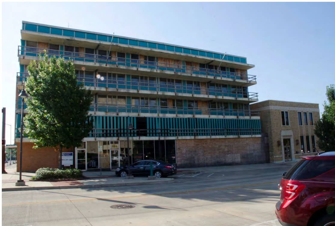
Photo 2: West (Secondary) Elevation. View southeast.
