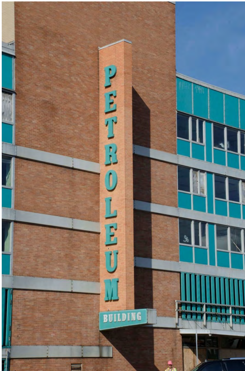
Photo 7: Signage Detail, North (Primary) Elevation. View southwest.
