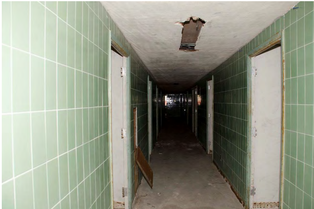
Photo 15: Fourth floor interior. View north.
