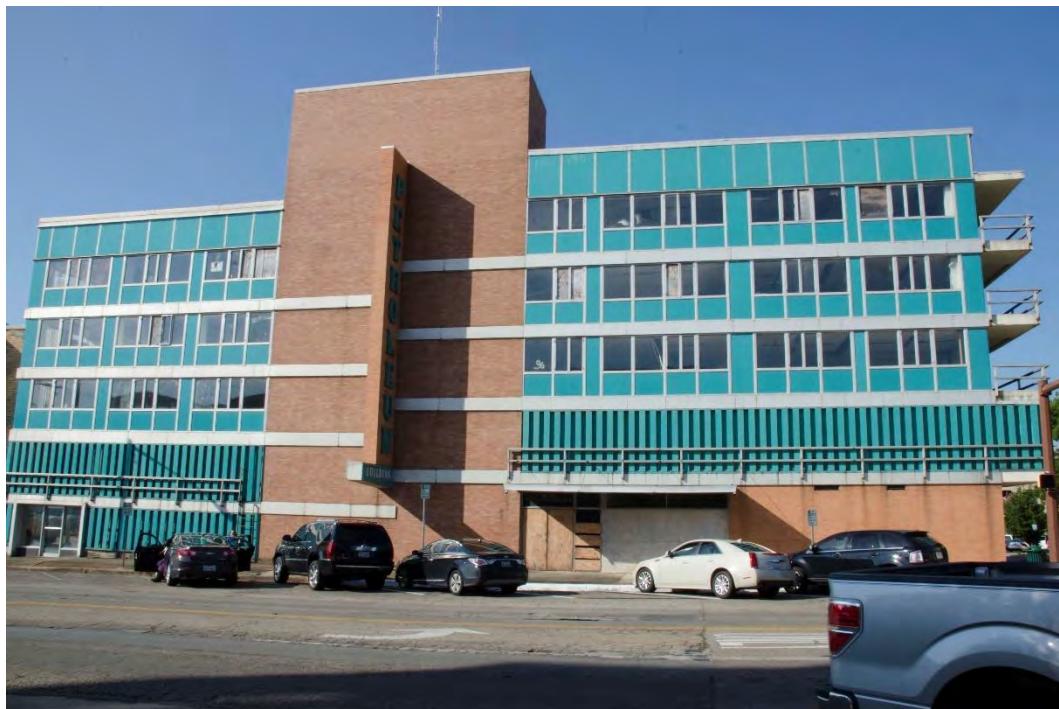
Photo 4: North (Primary) Elevation. View south.
