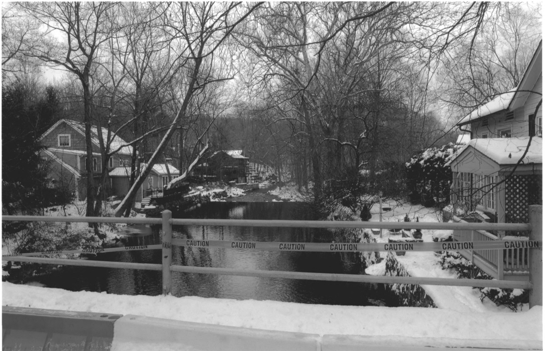
Perry Avenue Bridge Norwalk, Fairfield County, Connecticut Photograph 4 view south towards Timber Pond Dam December 11, 2005 Tod Bryant
