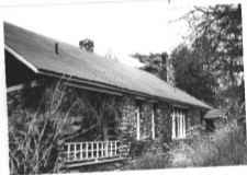
View looking NW. Neg. file # 19844-9
