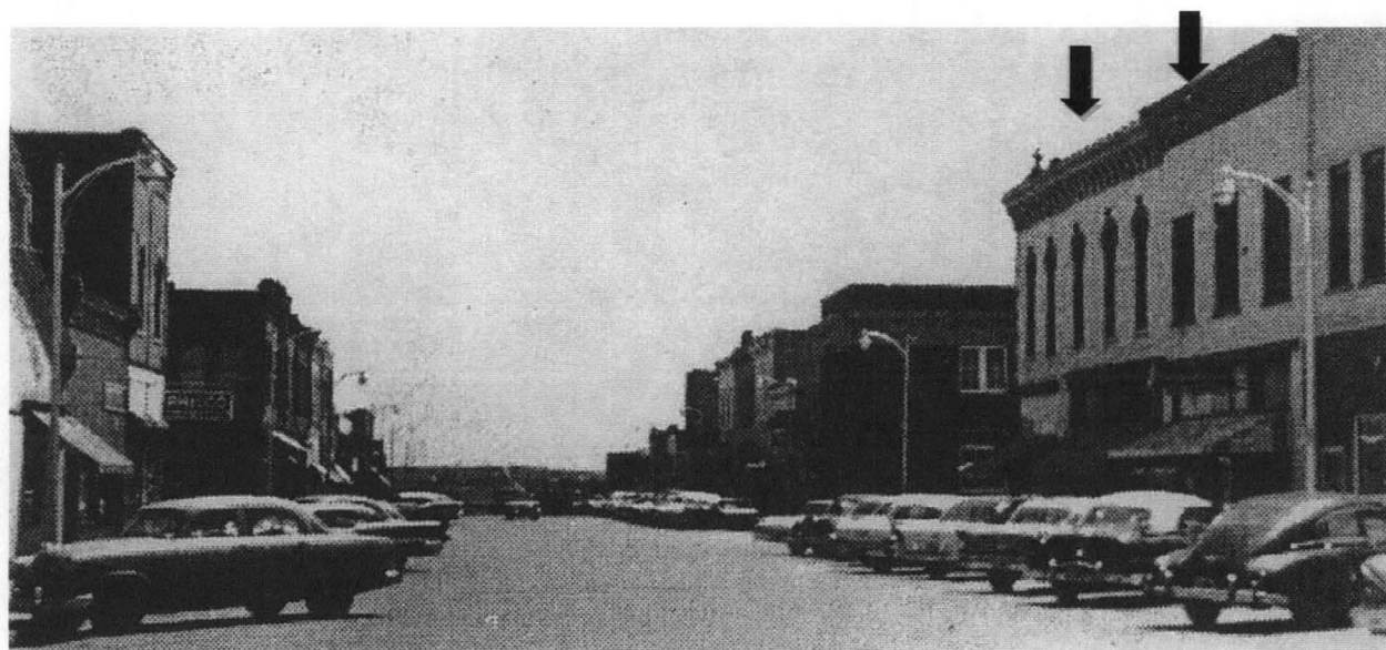
Figure 21: Photo of east façades, dated 1965. From Stephany, Dean, Woodbine Centennial 1866-1966, p. 47. Arrows indicate buildings being nominated – highlighting by APMA.
