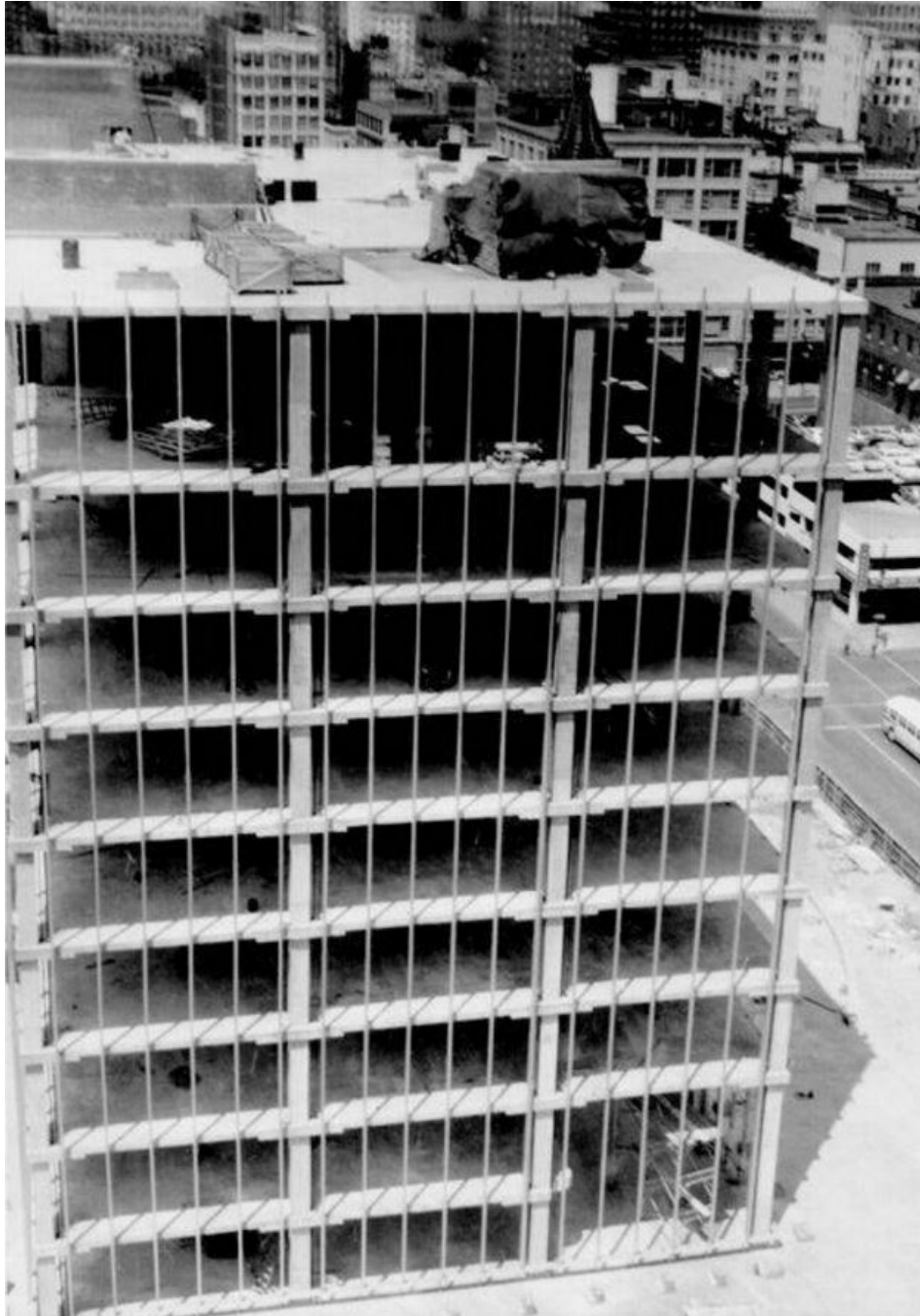
Figure 20. Historic Photograph, Construction, July 1959. Source: Missouri Valley Special Collections.
