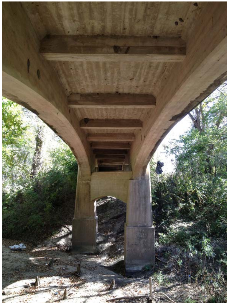
5. Substructure, looking east
