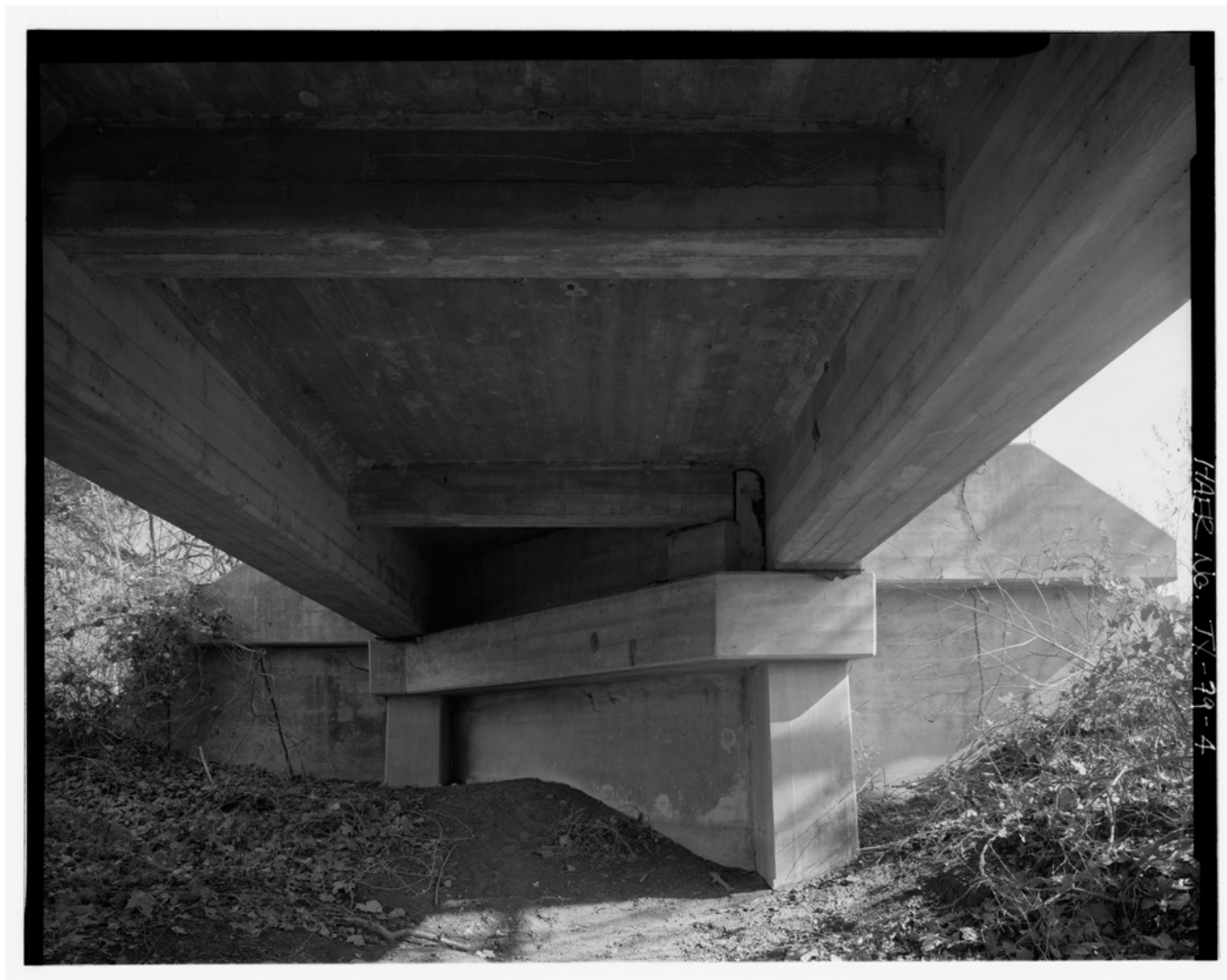
HAER Photograph by Bruce A. Harms (2001) East abutment, looking east
