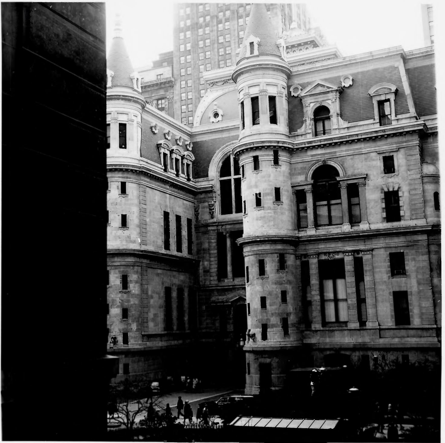
Philadelphia City Hall Inner courtyard
