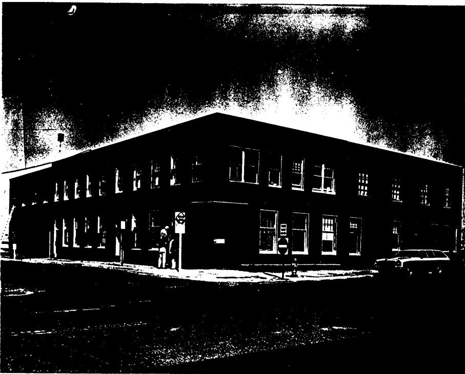
From 8th & Court 'A' (looking northeast)
