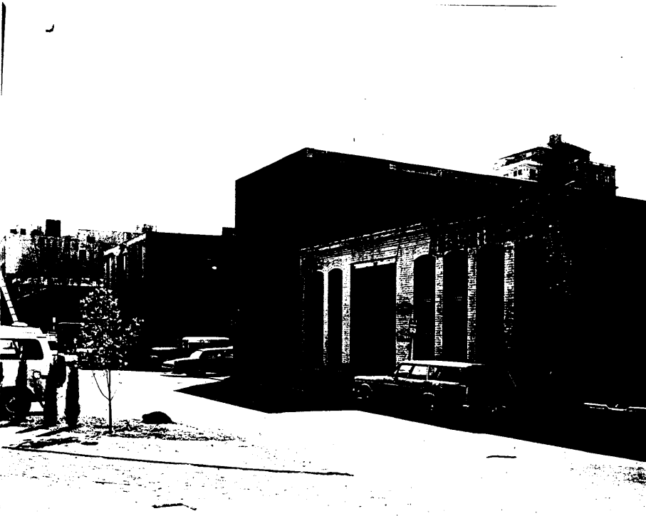
701 Pacific (garage in foreground, from Court 'A' looking southwest)
