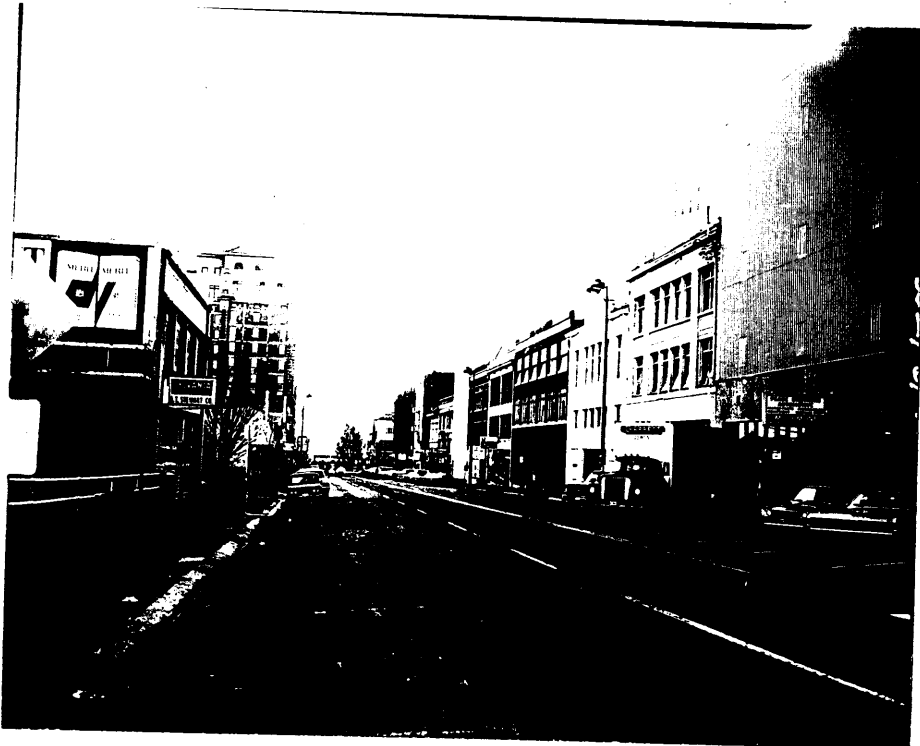
Looking south on Broadway from near the Spanish Stairs
