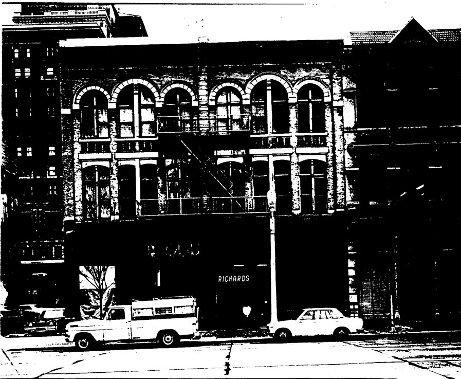
734 -36 Pacific, WEEKS BLDG. (Primary) (looking west from Pacific)
