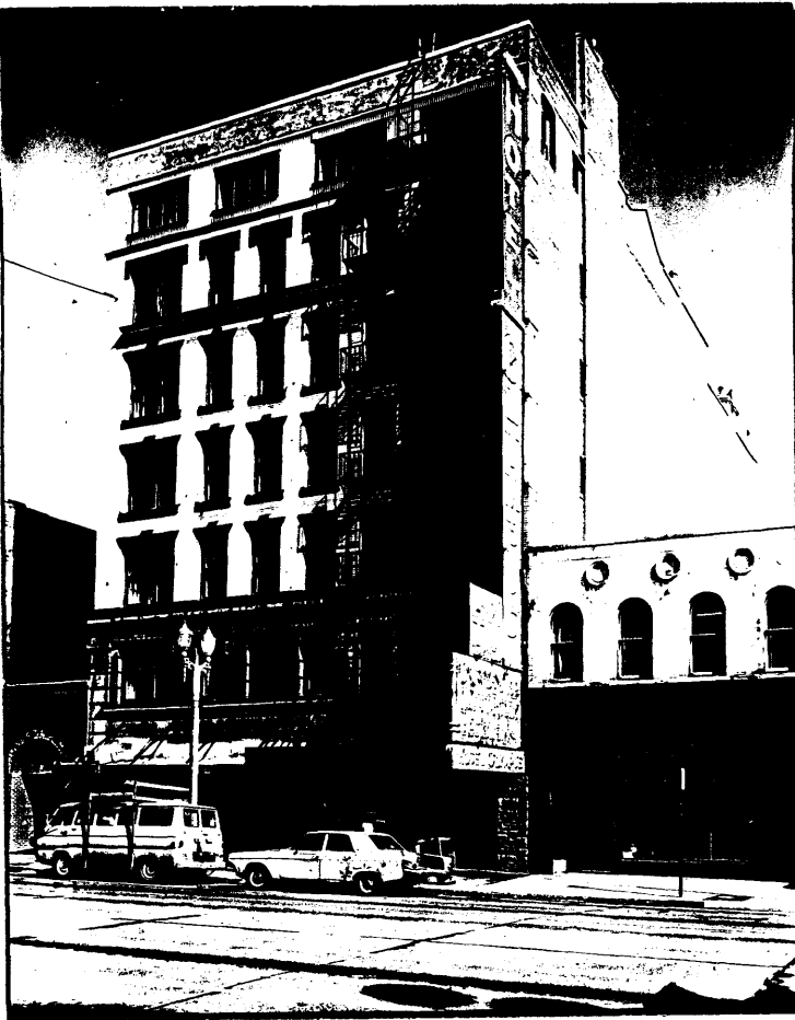
815 Pacific, OLYMPUS HOTEL (Primary) ( looking east from Pacific )
