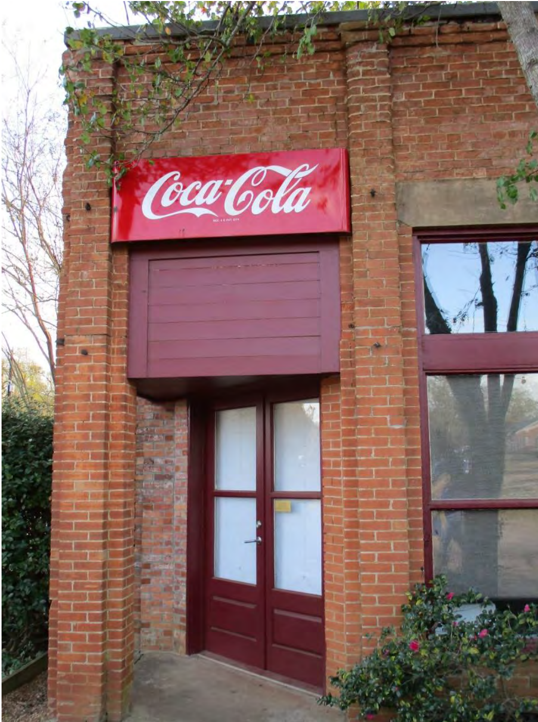
Photo 5: North façade of Mangham-McIlwain Building, detail of historic northeast corner double entrance and advertising. Camera facing south.
