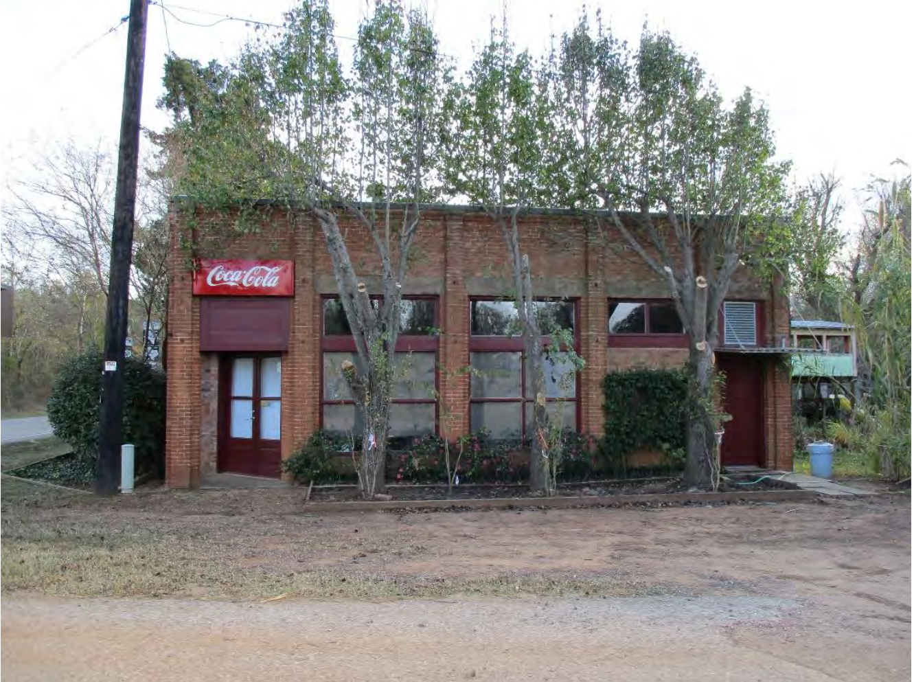
Photo 2: North façade of Mangham-McIlwain Building. Camera facing south
