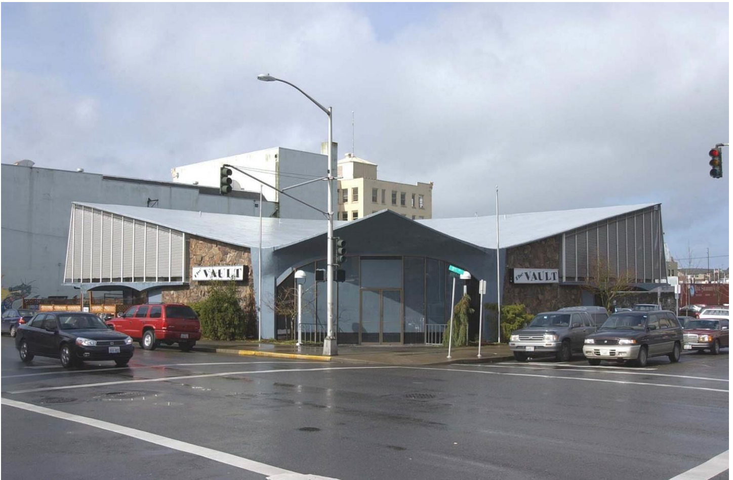
1 of 13 - SW corner of 5 th and Franklin looking northwest.
