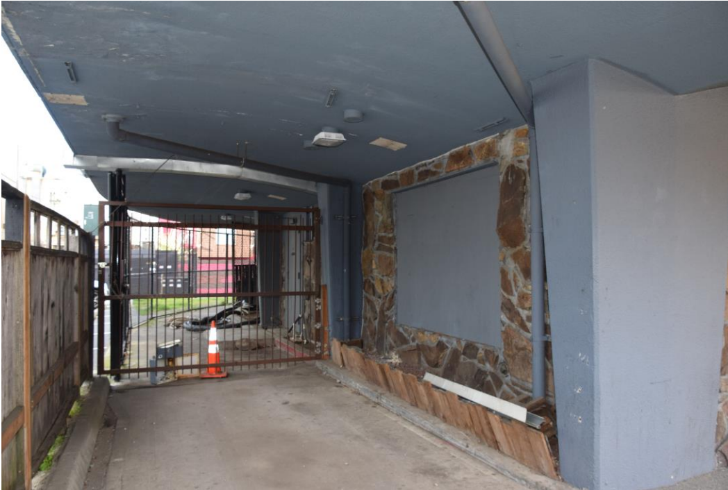
6 of 13 - Detail of former bank teller drive through window.
