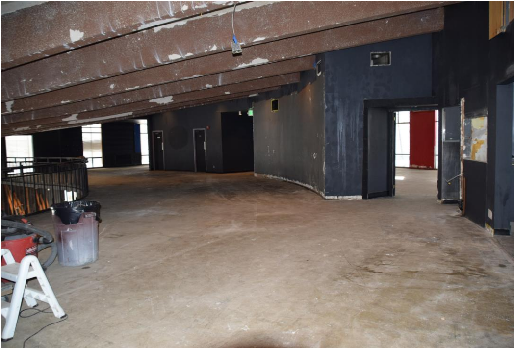
12 of 13 - View mezzanine area.
