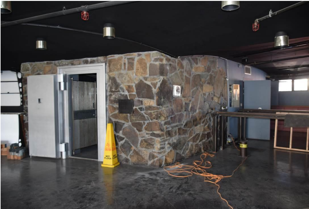
8 of 13 - Detail of main banking vault.
