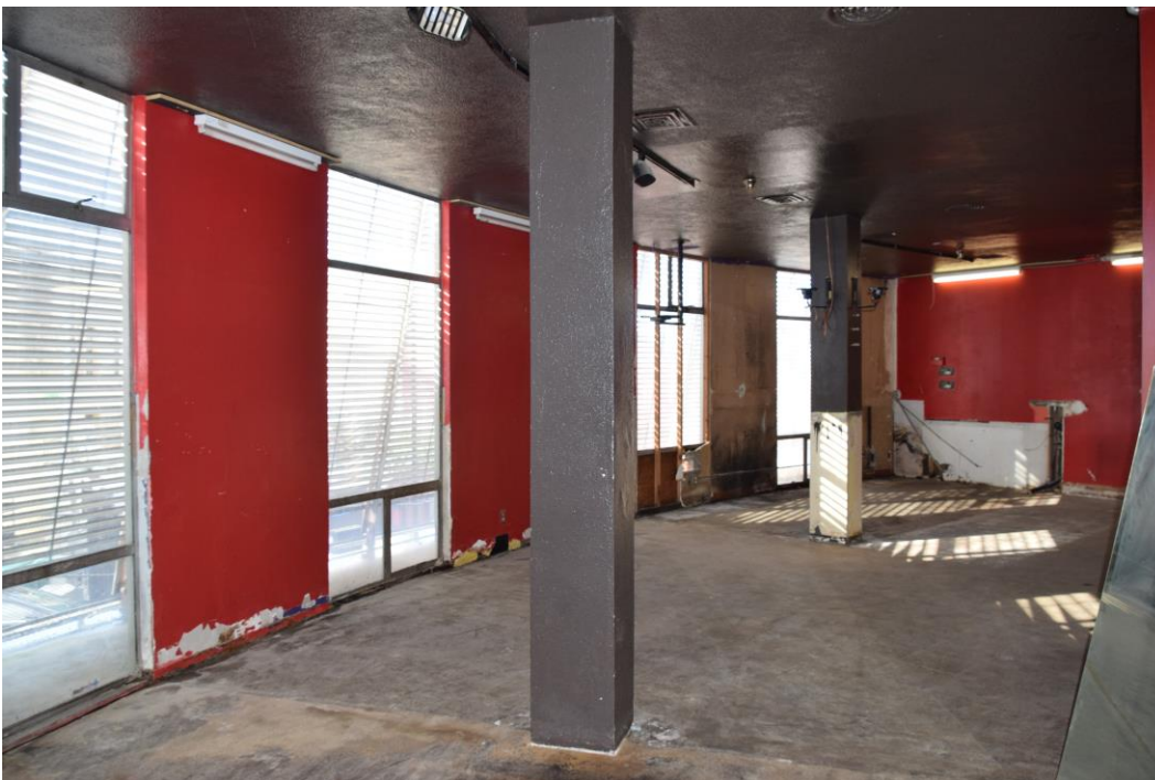
13 of 13 - View mezzanine/ second floor office area.
