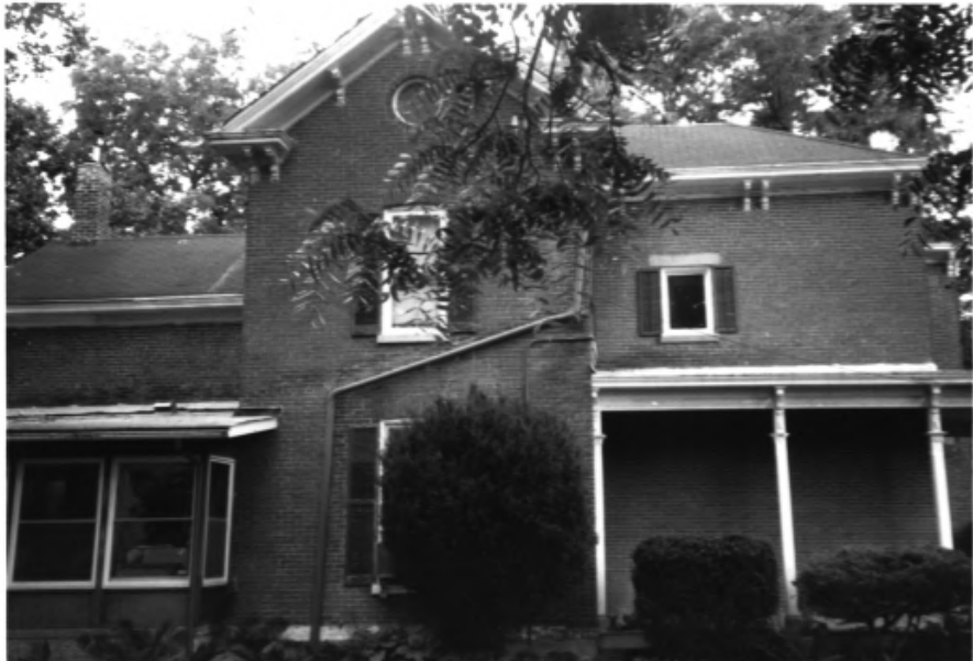
EUKEL HOUSE, JOHNSON COUNTY, IOWA 9
