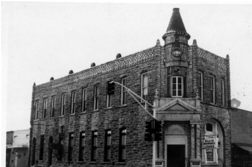
Figure 7 - Exterior view of First National Bank Building. Note replacement of metal cladding at 2nd floor turret is underway and large arched window at the front facade has been modified to accommodate new door; ca. 1930s. Camera facing northwest
