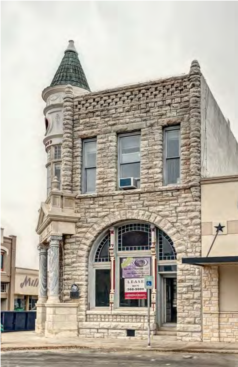
Photo 5 - North and East Elevation Oblique. Camera facing: Southwest
