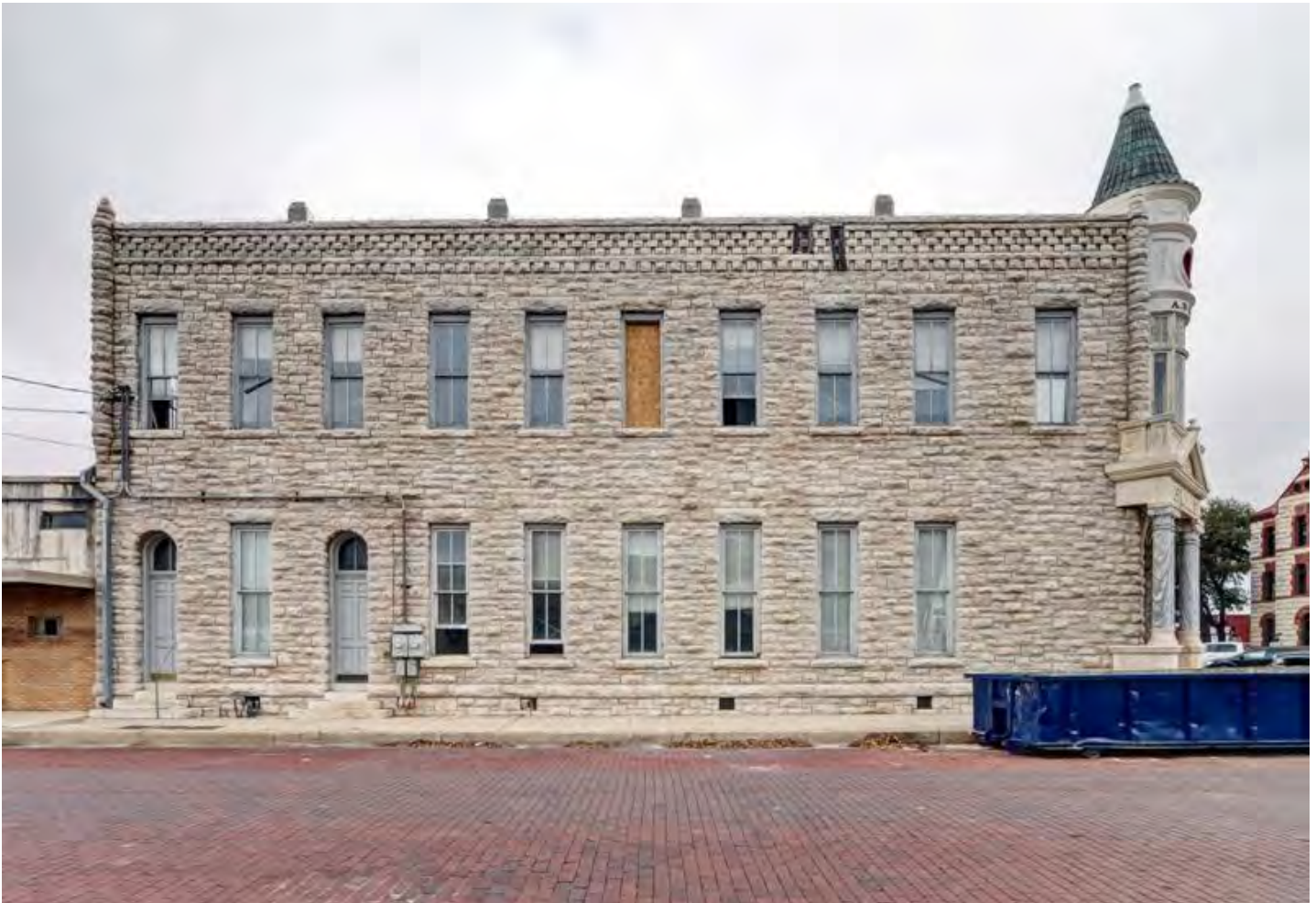
Photo 1 - South Elevation. Camera facing: North
