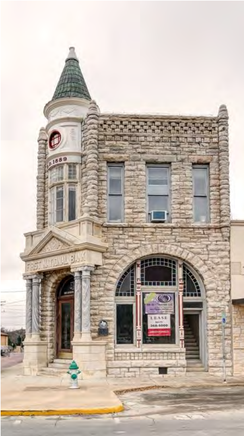
Photo 3 - East Elevation. Camera facing: West
