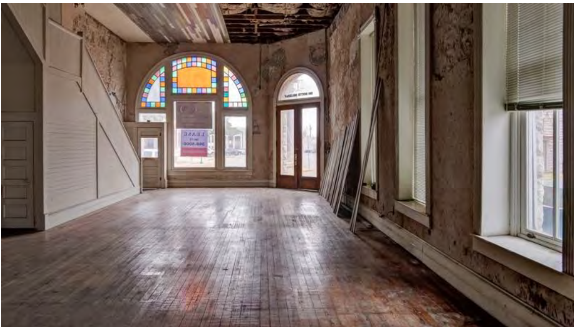
Photo 8 - Interior of First Floor Banking Space. Camera facing: East
