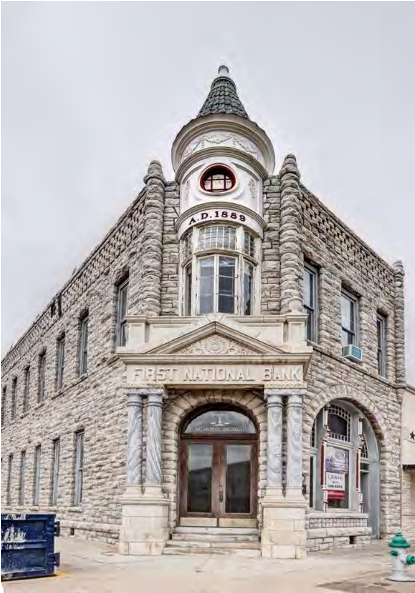
Photo 6 - Close-up of South and East Elevation Oblique with Corner Entrance. Camera facing: Northwest
