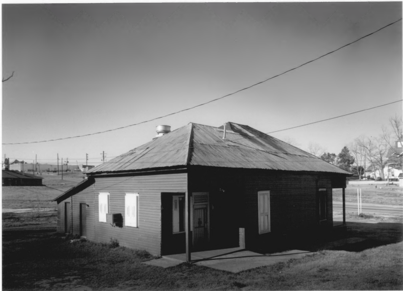
Dismuke Storehouse, Sumter County, GA 3 of 5
