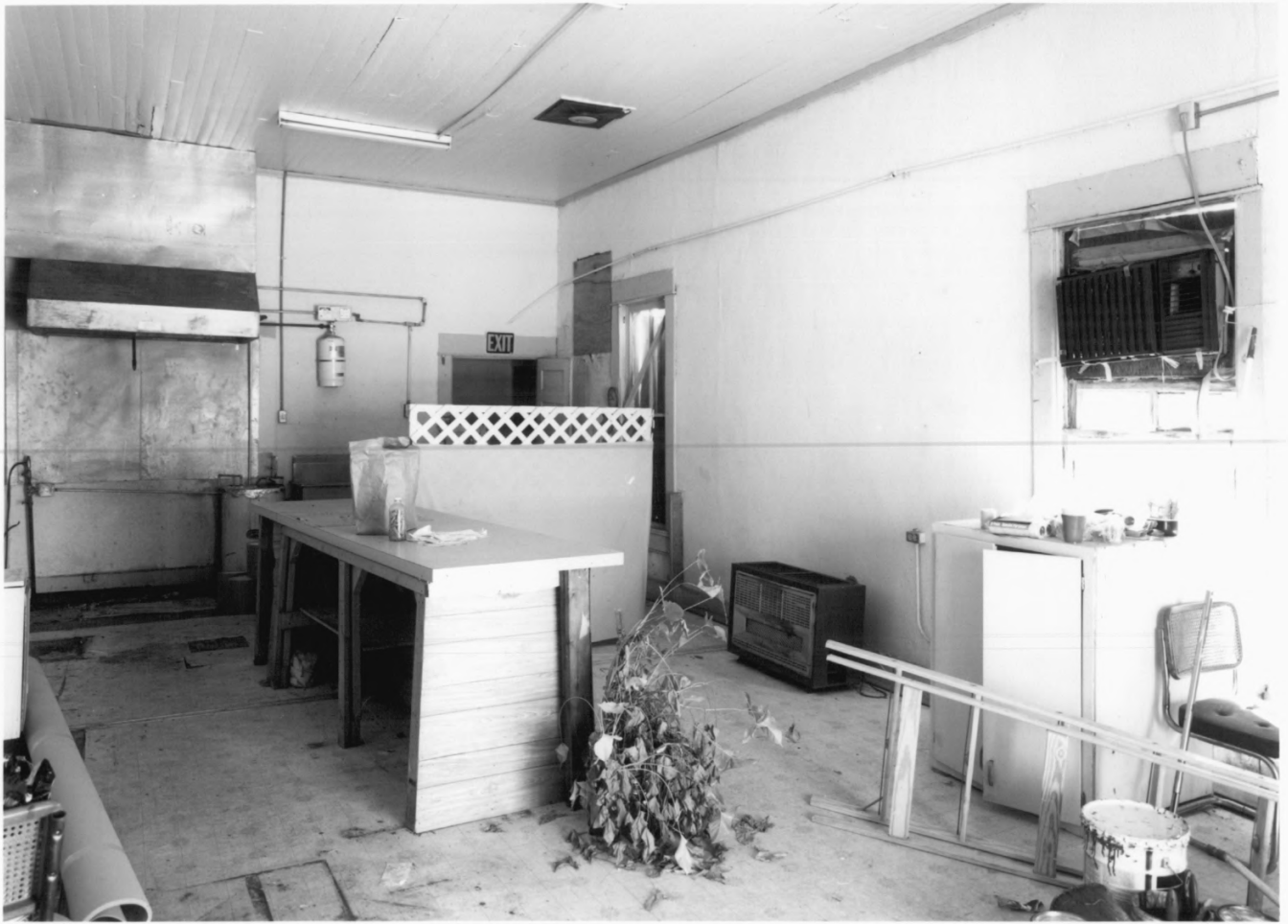
Dismuke Storehouse, Sumter County, GA 4 of 5
