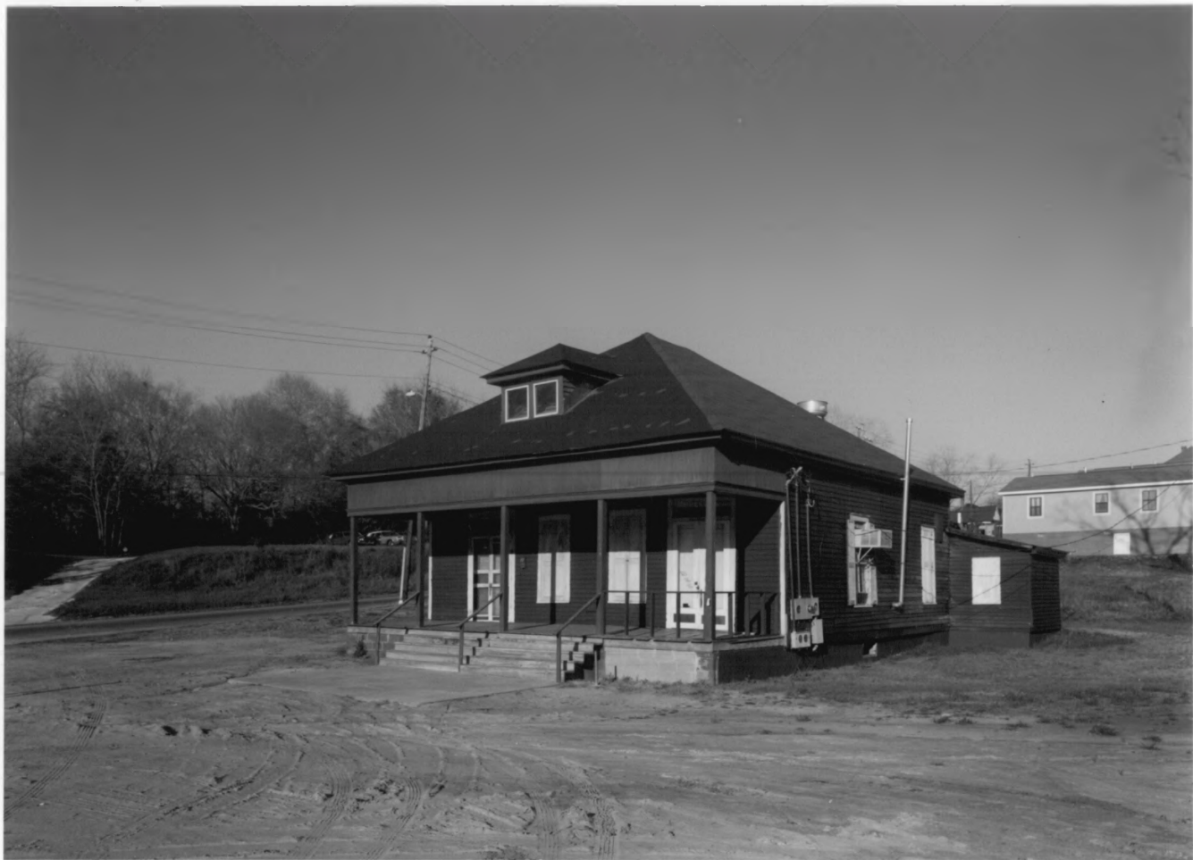
Dismuke Storehouse, Sumter County, GA
