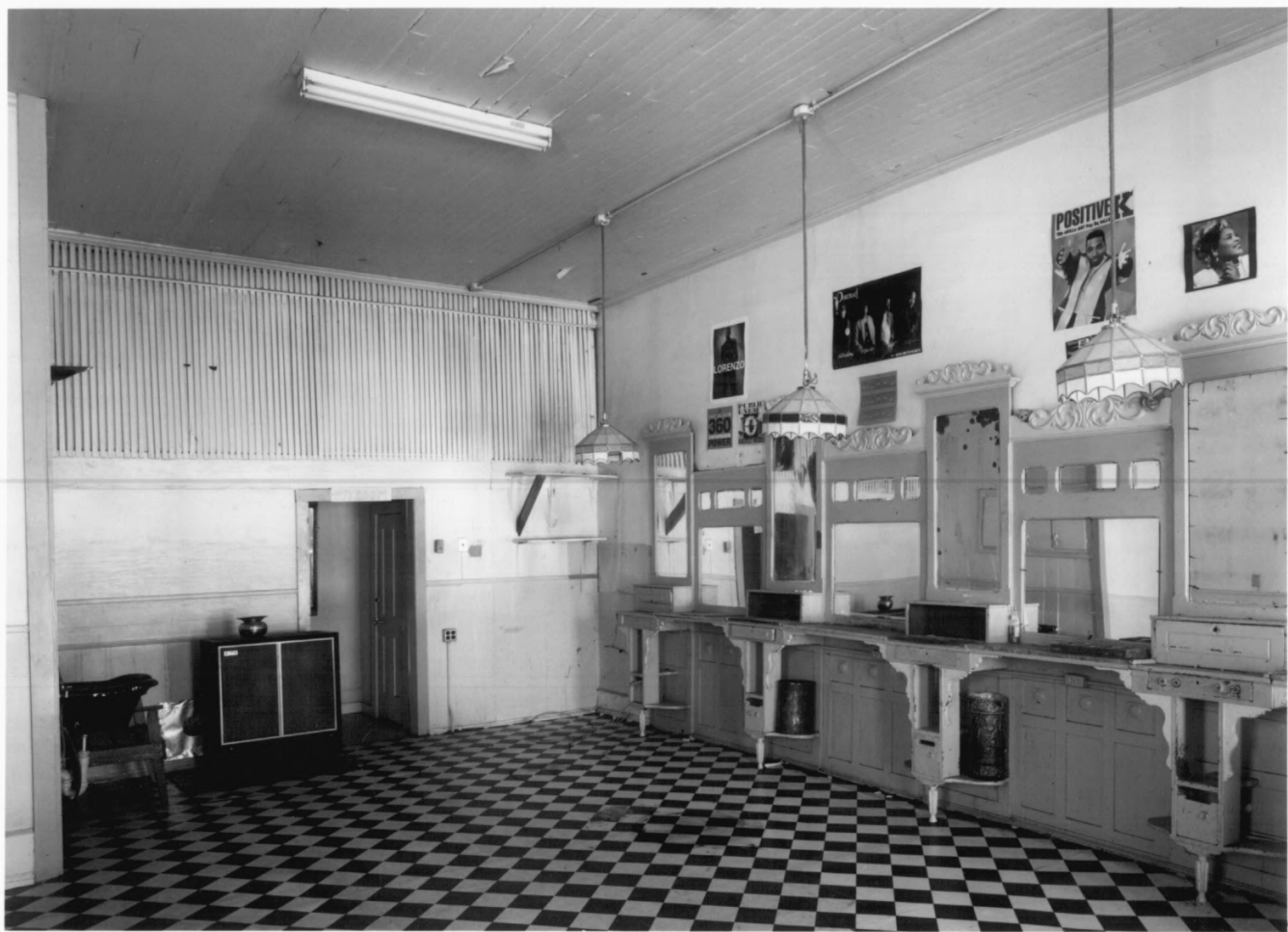
Dismuke storehouse, Sumter County, GA 5 of 5
