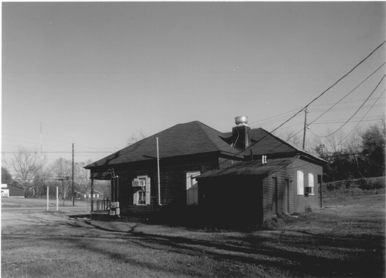
Dismuke Storehouse, Sumter County, GA 2 of 5
