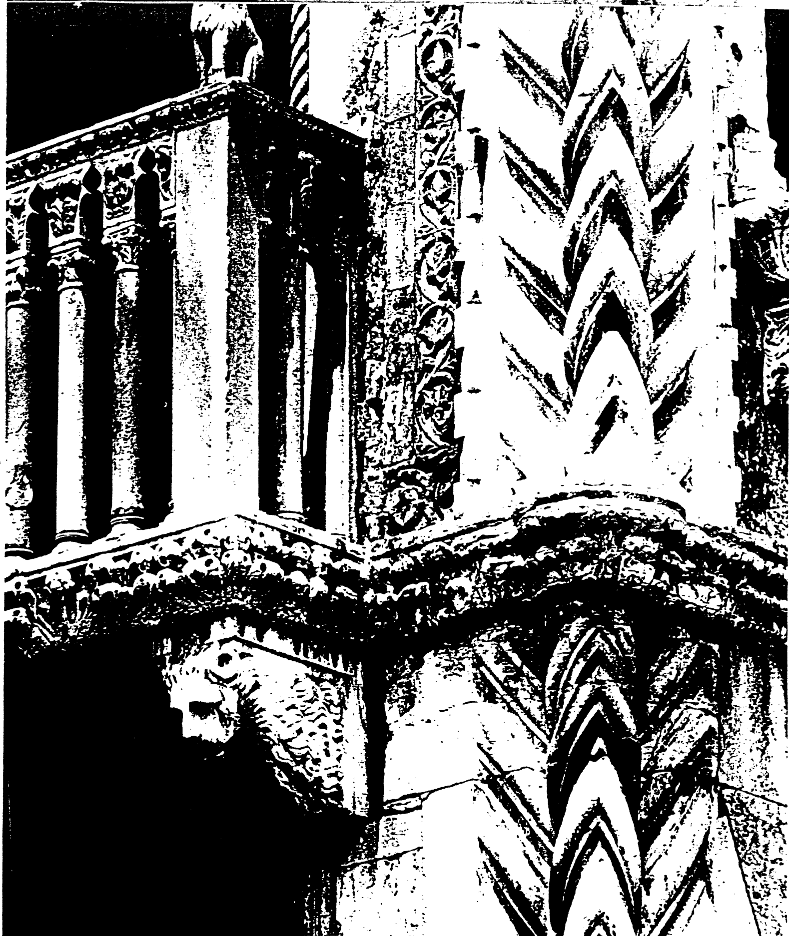
FIGURE 9 Lion's head bracket supporting balcony at Ca. D'Oro in Venice.
