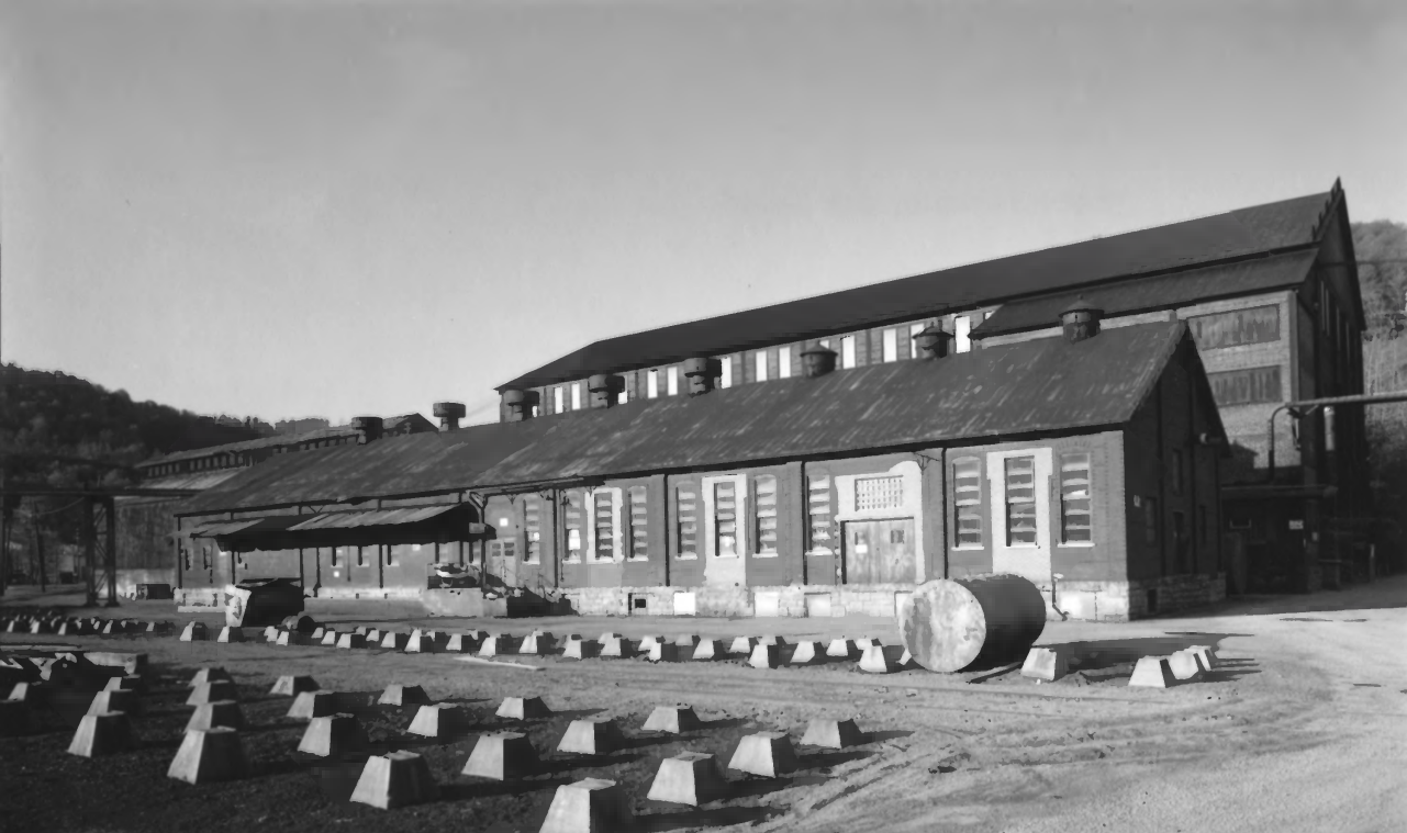
Cambria Iron Company Compressor Engine House Lower Works Johnstown, Pennsylvania
