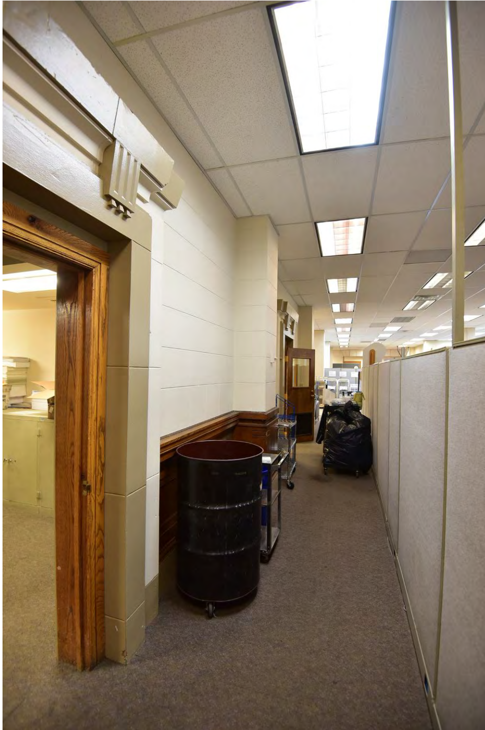
Figure 26. Historic door surround and scored plaster walls, 1 st floor of west wing. Brad Finch, 2017.
