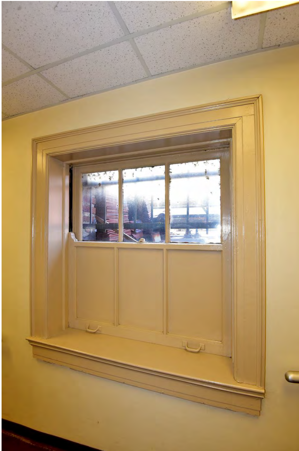
Figure 25. Partially infilled window with solid lights and historic surround. Brad Finch, 2017.
