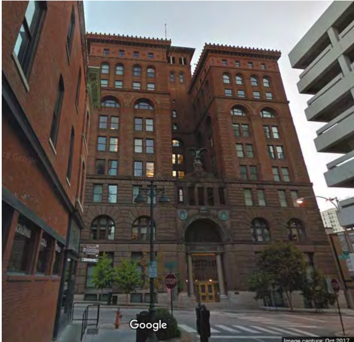
Figure 30. New York Life Building, 20 West Ninth Street, 2018. Source: Google Street View.
