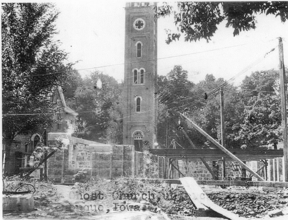
Figure 17. Church under construction in summer/fall 1916 (Holy Ghost parish files).
