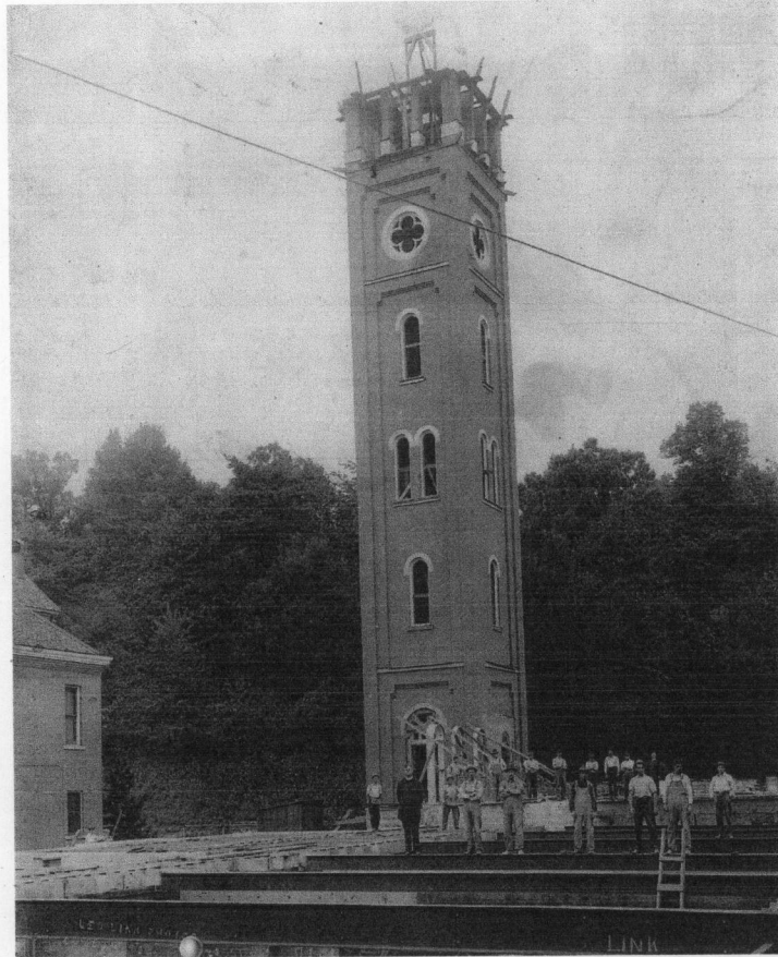
Figure 16. Church under construction in summer/fall 1916 (Holy Ghost parish files).
