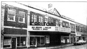
The Carlton Theatre, 1975 photo. The sign has been changed, but otherwise the façade remains unaltered two years after it closed. (Randy Gabrielian, Images of America: Red Bank Vol. 3 , 1998, page 88. Courtesy Special Collections and University Archives, Rutgers University Libraries.)
