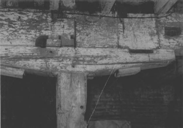
SEP 1 3 1978 11 423 OWINGS UPPER MILL Owings Mill, Baltimore County, Md. Photo by John McGrain Sept. 1974 Groff's Mill - post, bolster & girt construction, 1st story
