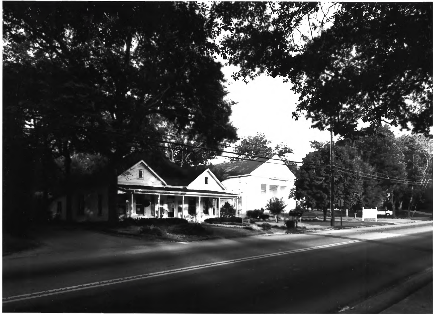
JEFFERSON HISTORIC DISTRICT JEFFERSON, JACKSON COUNTY, GEORGIA PHOTOGRAPH F20 OF 86
