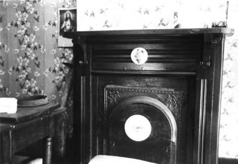
PHOTO **8**Cast iron mantel in upstairs of Section B.
