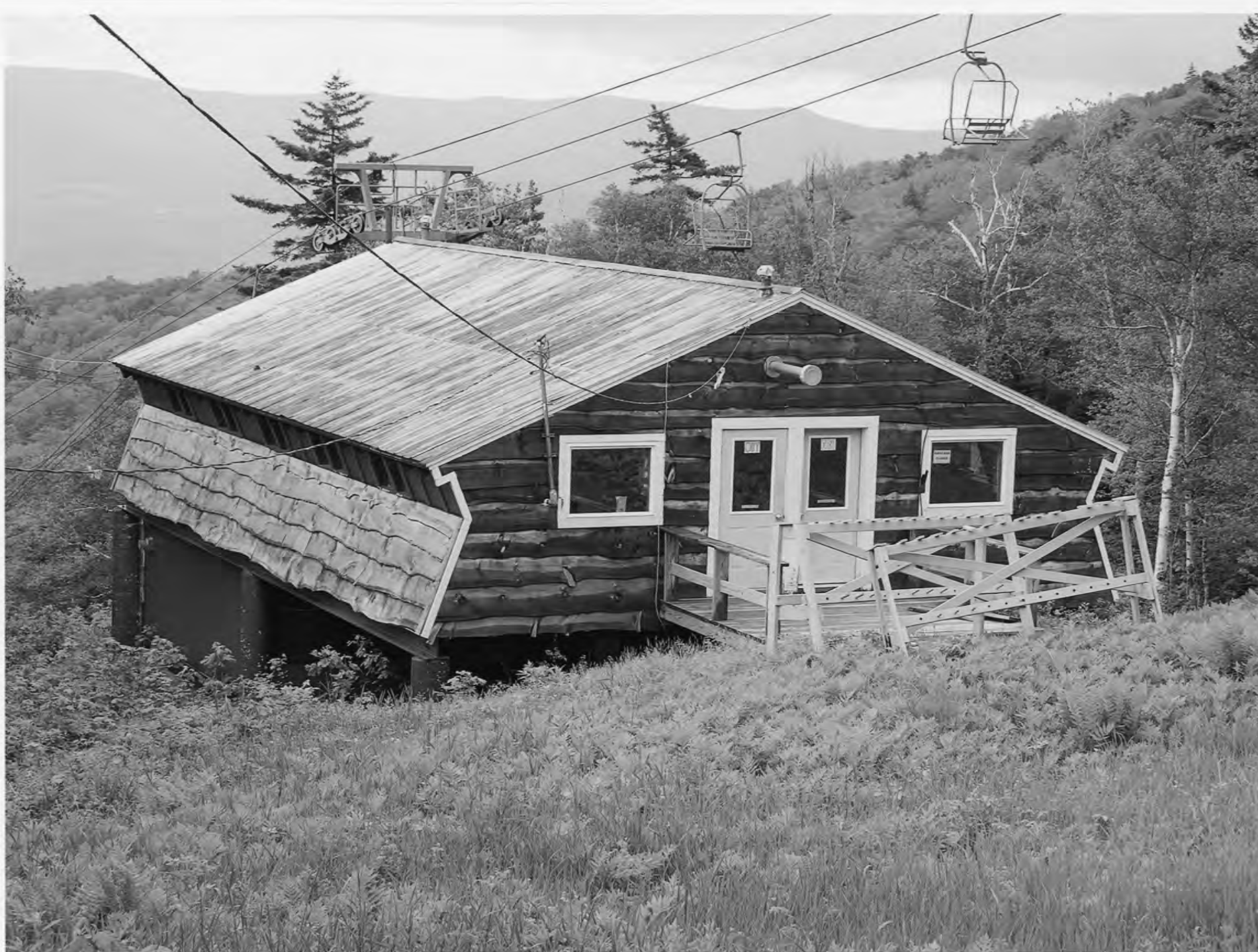
Mad River Glen Ski Area Historic District, Fayston, Washington Co. & Buel's Gore, Chittenden Co., Vermont Photograph # 46 of 56 Birdcage (60) & Sunnyside Double Chair Lift (49), view looking southeast
