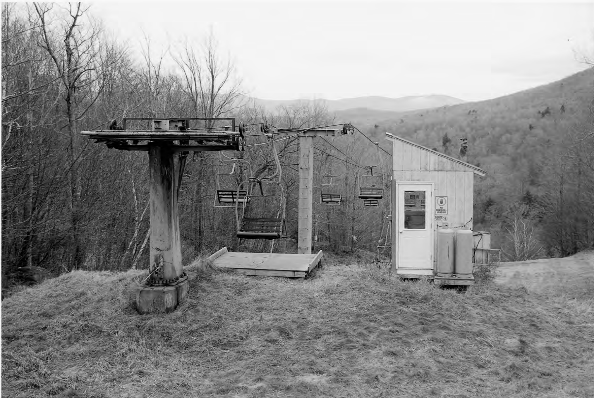
Mad River Glen Ski Area Historic District, Fayston, Washington Co. & Buel's Gore, Chittenden Co., Vermont Photograph # 31 of 56
