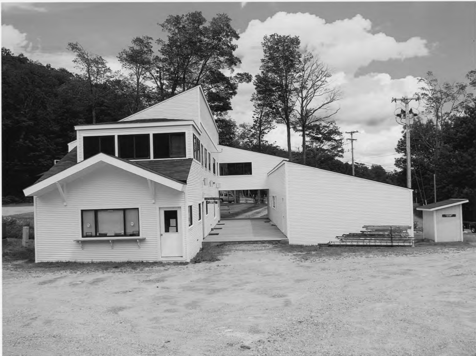
Mad River Glen Ski Area Historic District, Fayston, Washington Co. & Buel's Gore, Chittenden Co., Vermont Photograph # 37 of 56 Ski Shop/Entry Building (52) rear (west) facade & Vehicle Fueling Shed (58), view looking east
