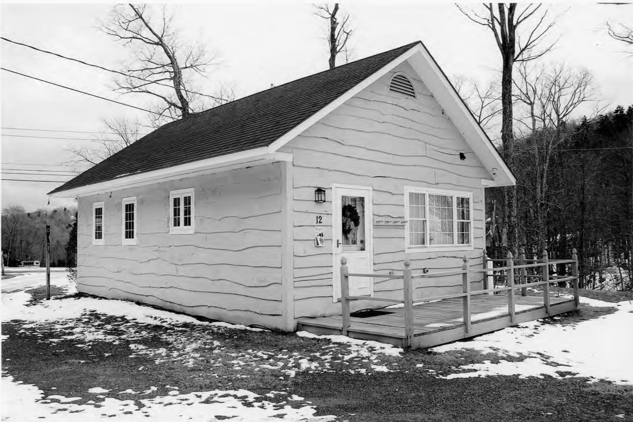
Mad River Glen Ski Area Historic District, Fayston, Washington Co. & Buel's Gore, Chittenden Co., Vermont Photograph # 35 of 56 Chalet X (51), front (west) and north facades, view looking southeast
