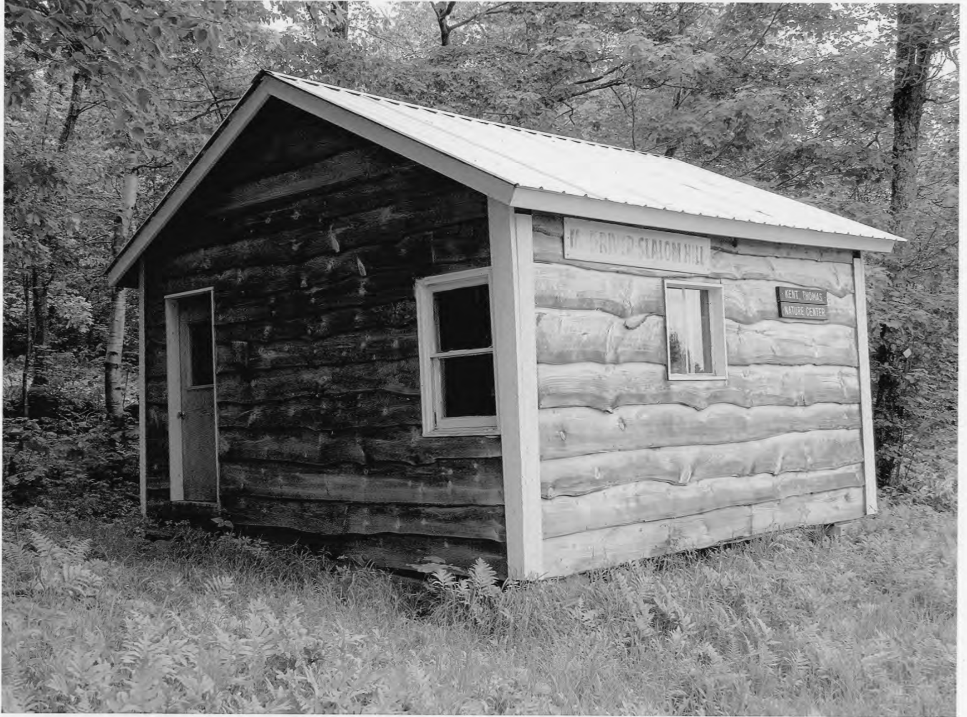
Mad River Glen Ski Area Historic District, Fayston, Washington Co. & Buel's Gore, Chittenden Co., Vermont Photograph # 45 of 56 Kent Thomas Nature Center (59), view looking northeast
