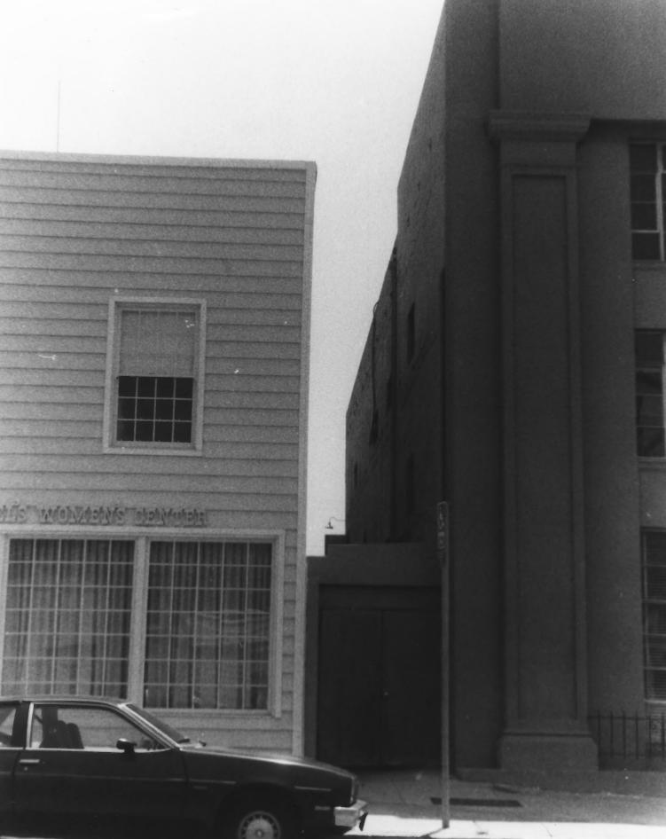
Eagles Hall, 733 8th Avenue, San Diego Photograph taken June 15, 1984 by Ray Brandes, 2725 Barnson Place, San Diego, CA 92103. Photograph shows north wall; taken from west to east. The north facade is built of brick which has been coated with a stucco finish. Photograph 6 of 10 photographs.
