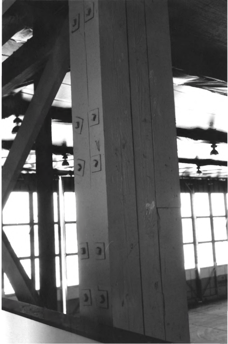
Hangar No. 1 Cape May County, NJ No. 8 of 15
