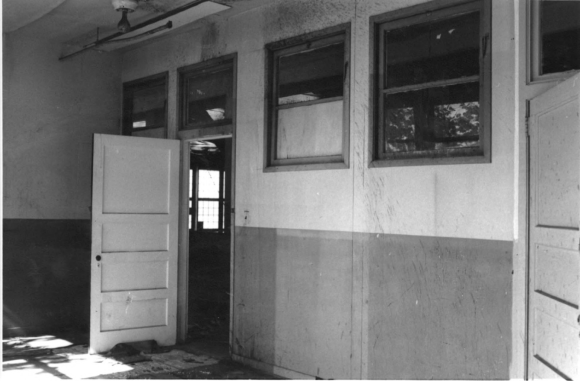
Hangar No. 1 Cape May County, NJ
