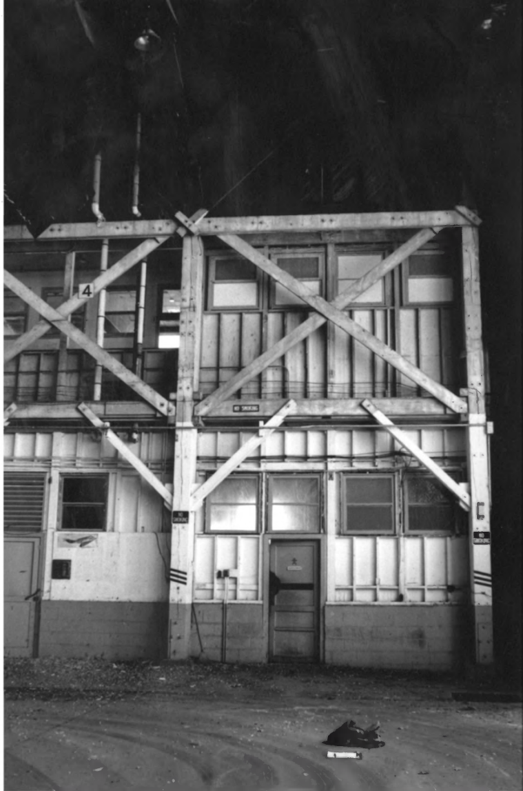
Hangar No. 2 Cape May County, NJ No. 12 of 15
