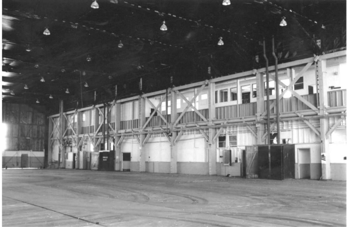
Hangar No. 1 Cape May County, NJ No. 14 of 15
