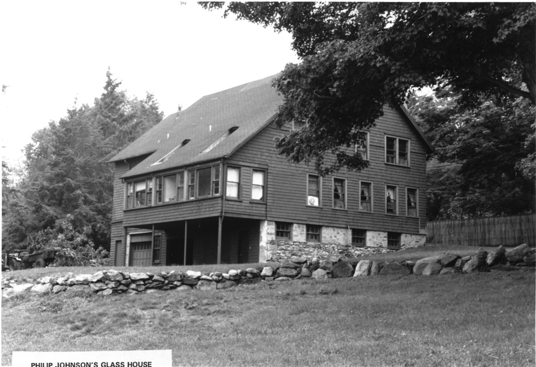
PHILIP JOHNSON'S GLASS HOUSE Fairfield County, Connecticut Caretaker's House, c. 1910 Photo: Historic Resources Consultants, Inc., July 1996
