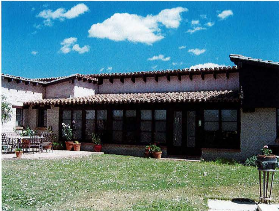
Figure 6. Glass enclosed sunroom (formerly screened porch), modified pre-1948. Looking northwest.
