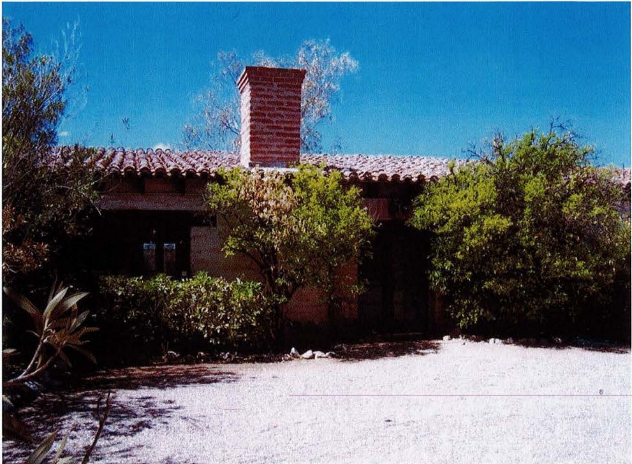
Photo #4 (AZ_PimaCounty_CFEJob#399House_0004) Front (north) façade, camera facing southwest.
