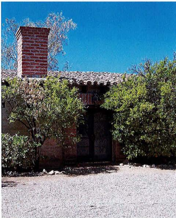
Figure 4. Entry Door Brick Surround (1948+). Looking southwest.
