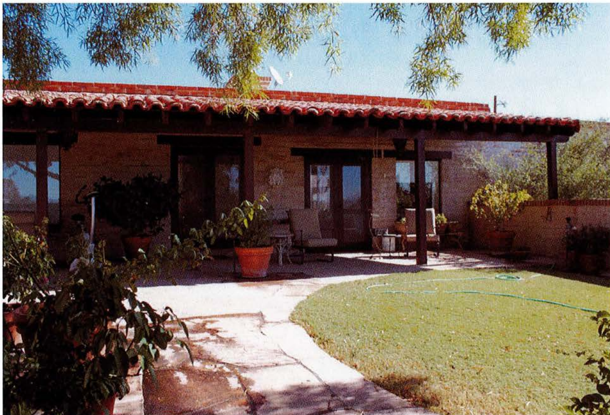
Photo #14 (AZ_PimaCounty_CFEJob#399House_0014) South façade, east wing addition (1969), camera facing northeast.
