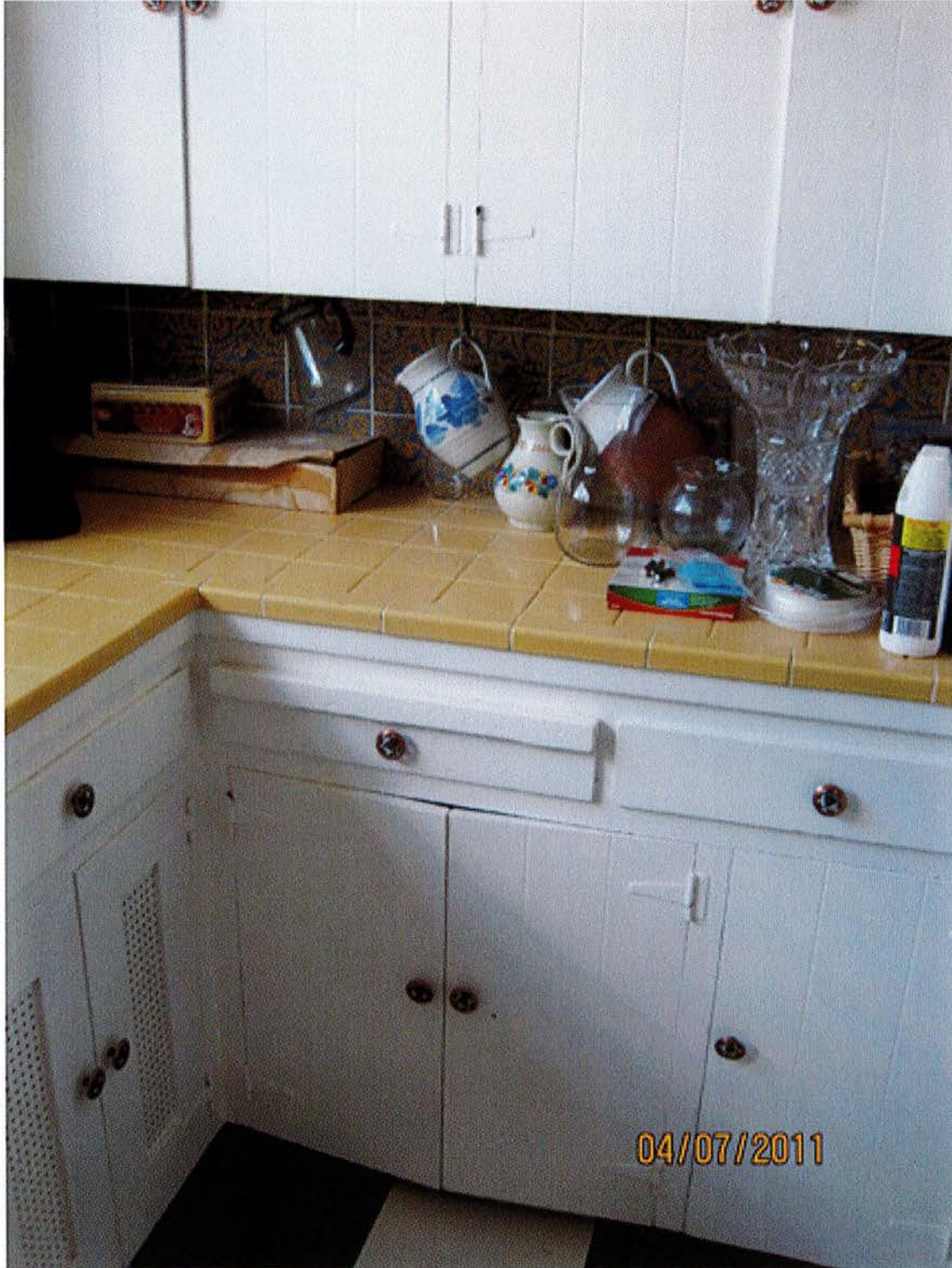
Photo #12 (AZ_PimaCounty_CFEJob#399House_0012) "Mexican Kitchen," original kitchen details, camera facing northwest.
