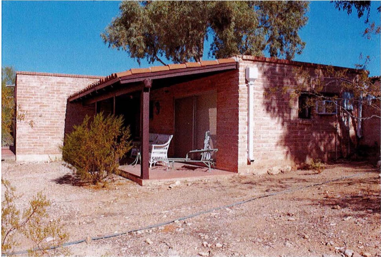
Photo #13 (AZ_PimaCounty_CFEJob#399House_0013) Guest House, Garage (1979), camera facing northwest.
