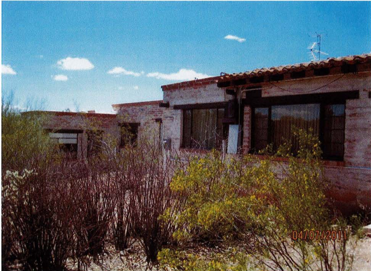
Photo #5 (AZ_PimaCounty_CFEJob#399House_0005) Compatible east addition, camera facing southeast.
