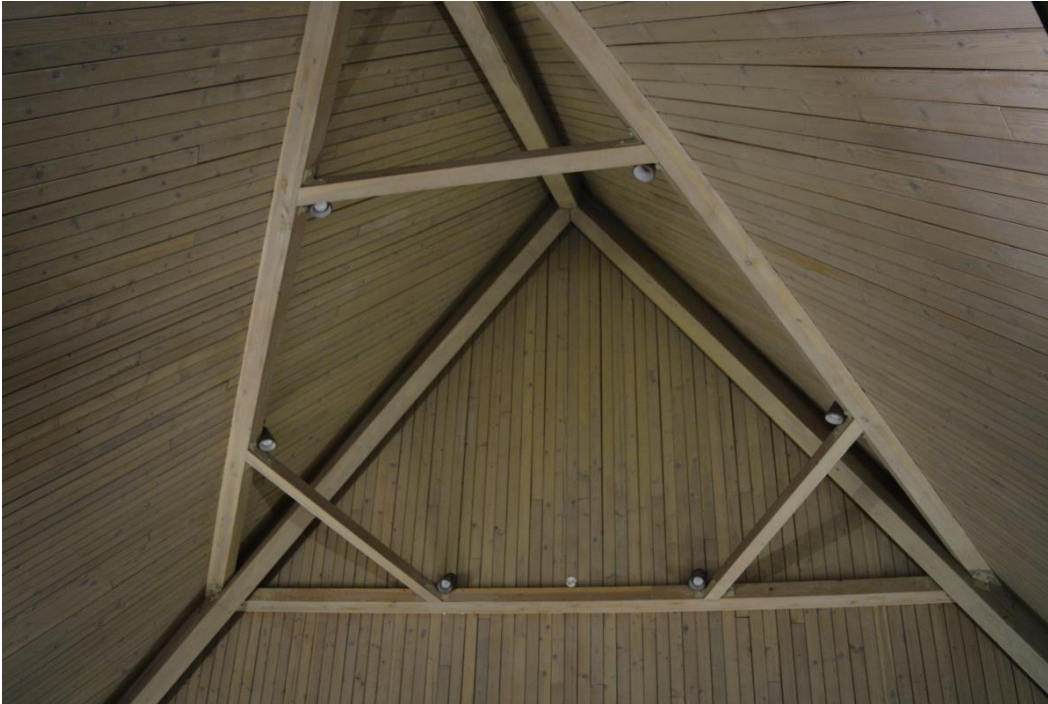
Looking up at the pyramidal roof, in the permanent gallery. 16 of 22.
