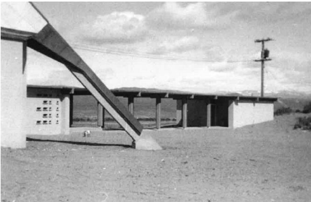
Nearly completed Interpretive Center. Finished comfort station and preezway. Main buiding on left. Looking east.
