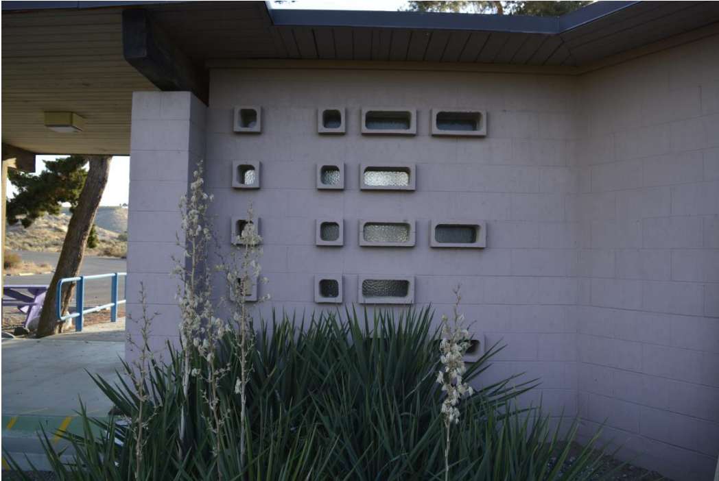
Looking northeast at the square and rectangular window cutout in the cinderblock walls of the entrance vestibule. 10 of 22.
