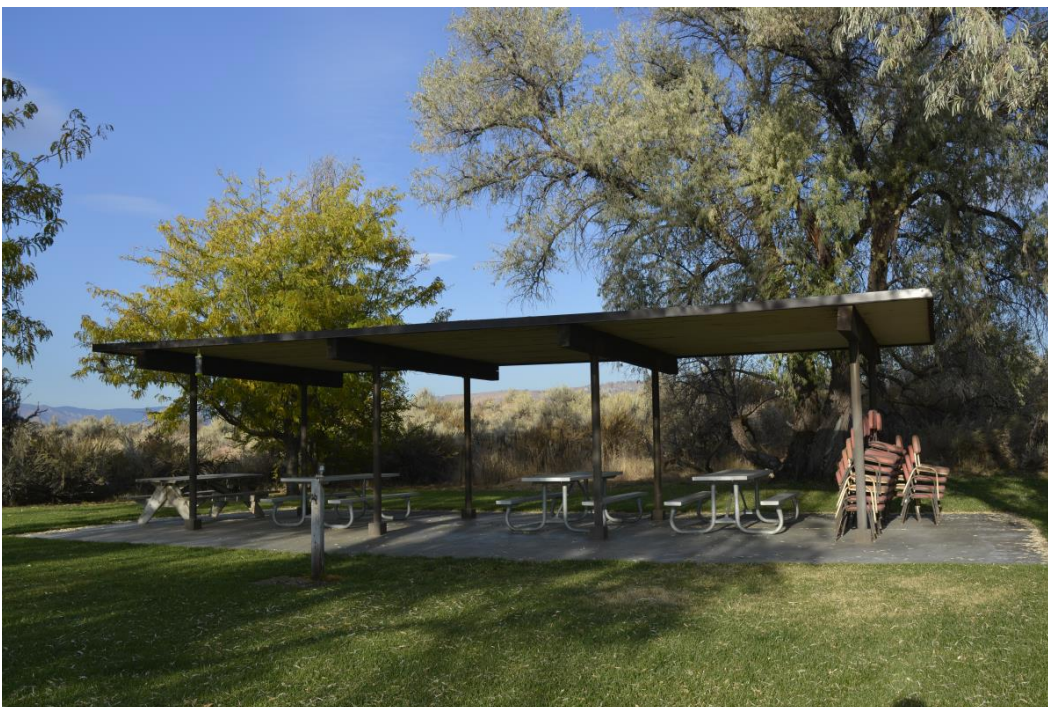
The flat roofed picnic shelter. 11 of 22.
