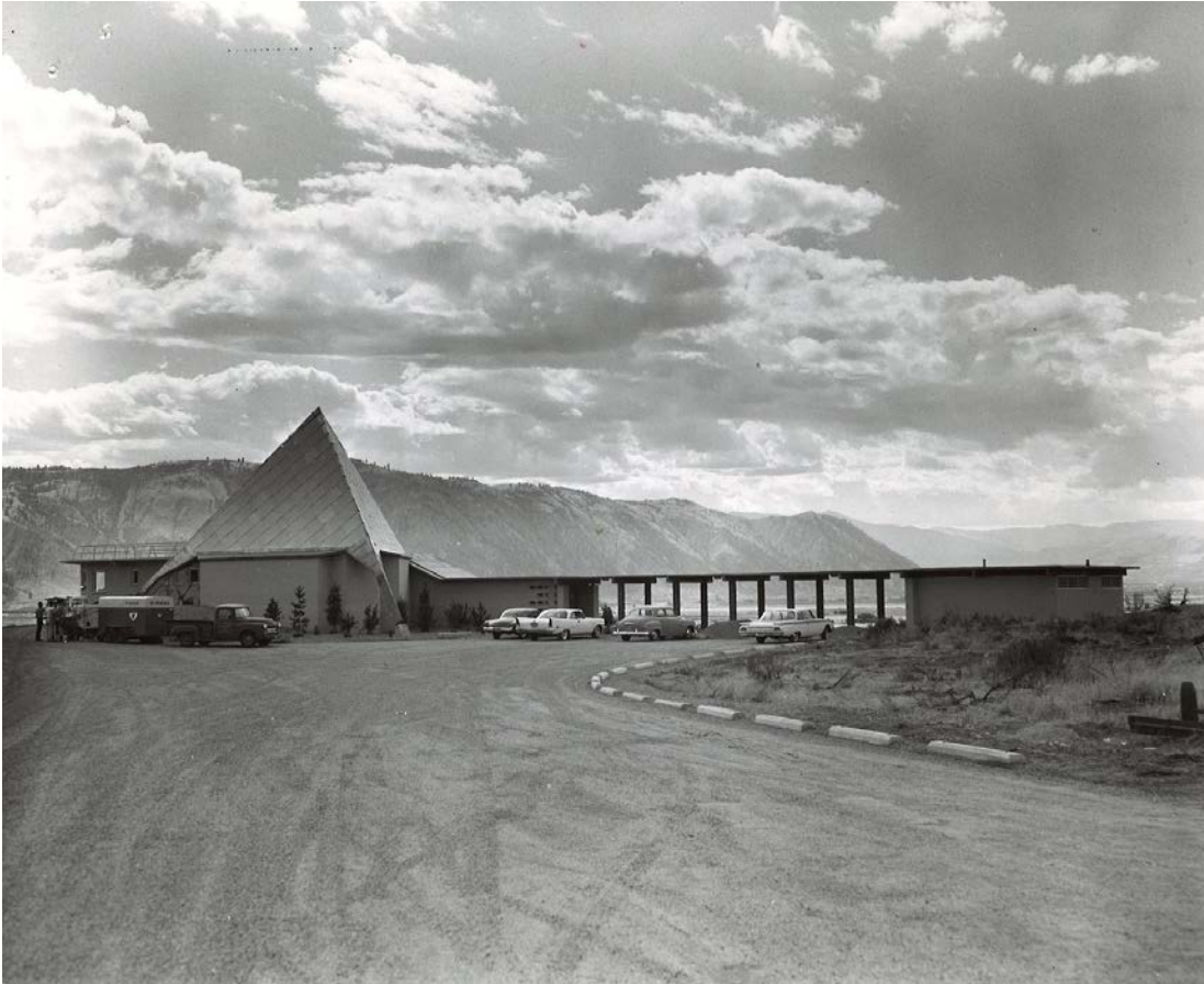
Completed Fort Okanogan Interpretive Center. Photographer: Parker McAllister, 1960
