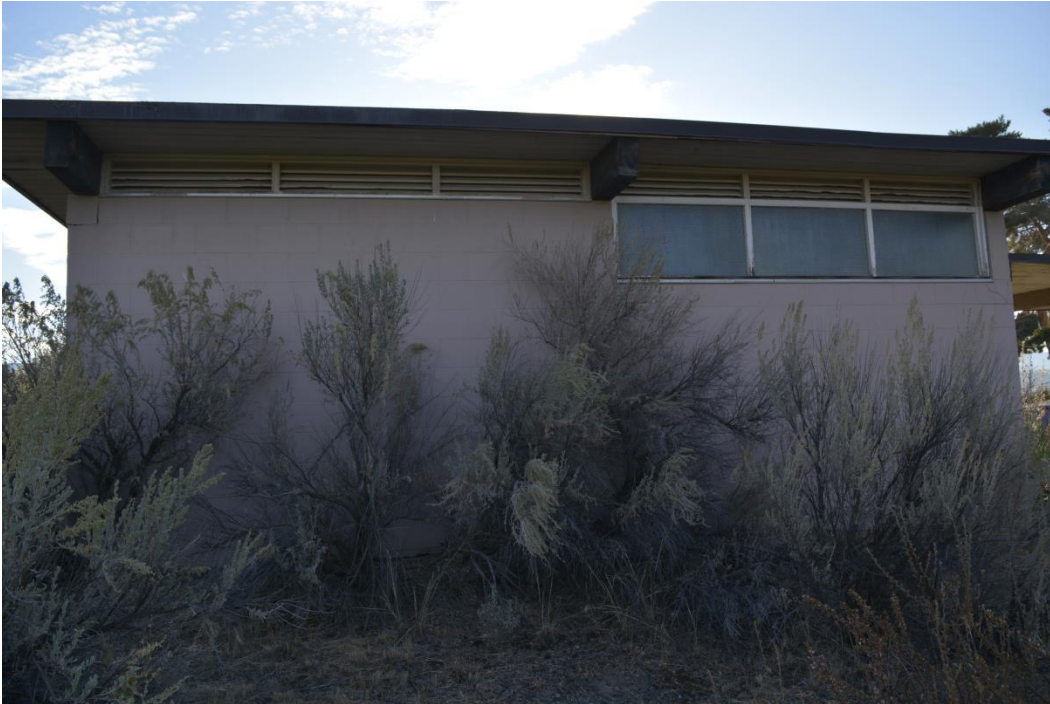
Looking at the south wall of the public restrooms. 6 of 22.
