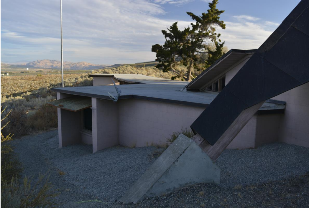
Looking northwest at the main entrance, breezeway and public restrooms. A concrete foundational block and one of the large beams creating the triangular peaked roof are in the foreground. 8 of 22.
