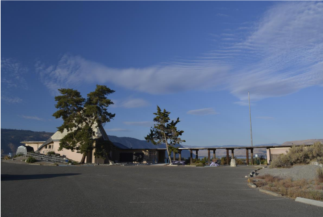
Looking south at the Fort Okanogan Interpretive Center. From Left to right, backing living quarters (flat roof), main gallery (pyramidal roof), greeting area (flat roof), breezeway connecting to the public restrooms on the left side of the photograph.
