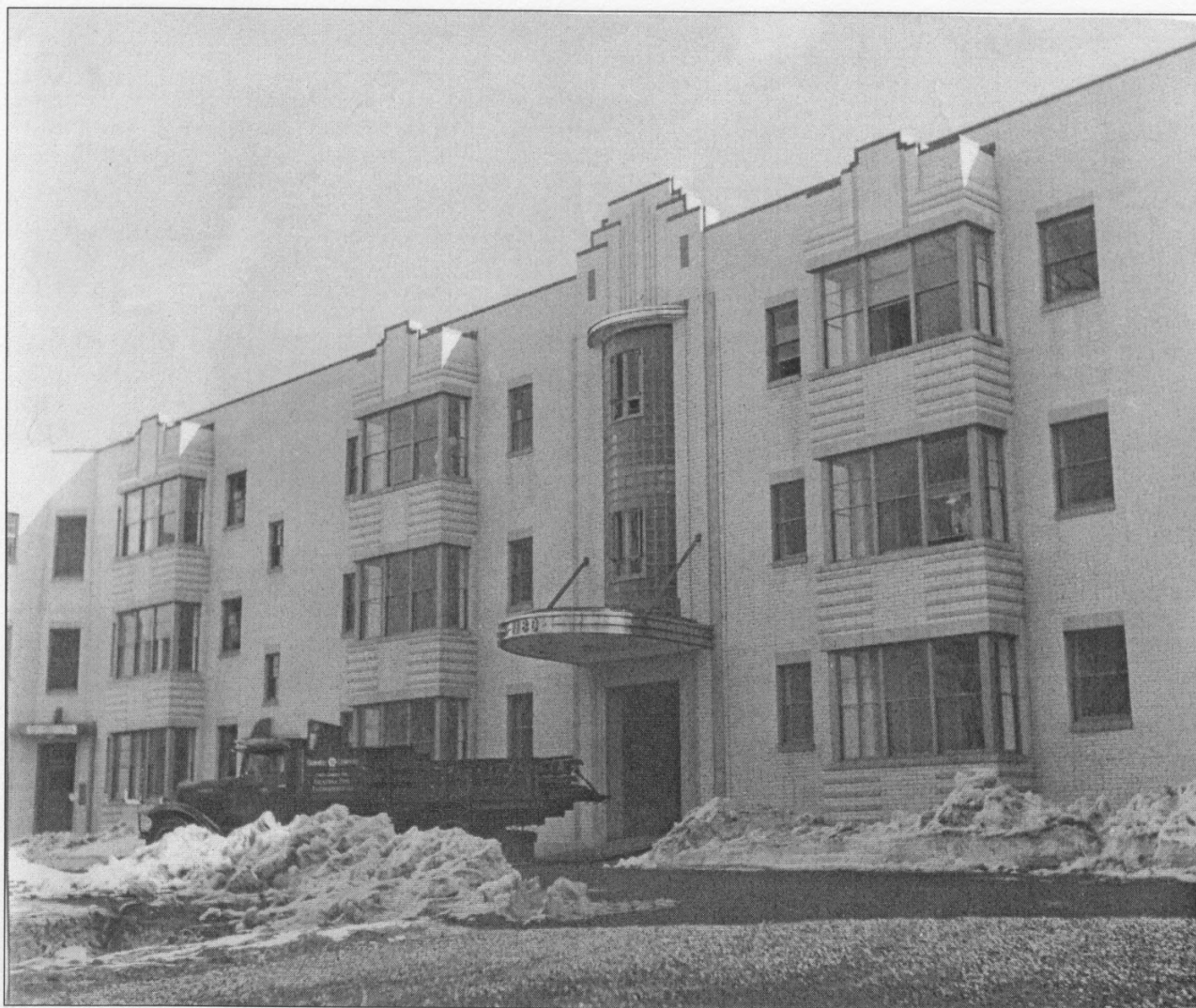
Figure 1 Historical photo of Rosedale Apartments Front elevation, ca 1940. Courtesy of Steven R. and Joanna Hunt
