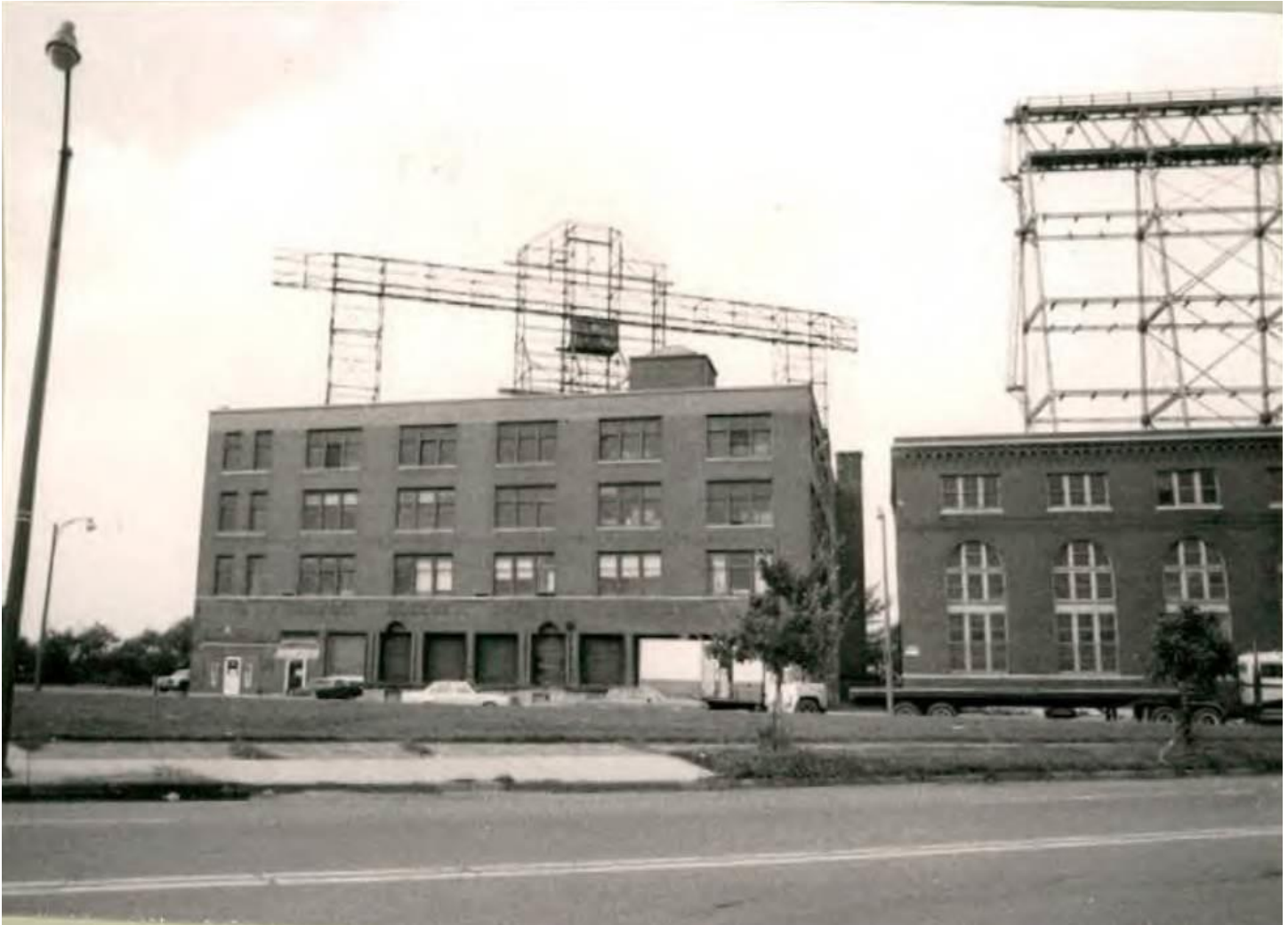
Buffalo General Electric Company Service Building (1981) From Historic Resource Inventory Form
