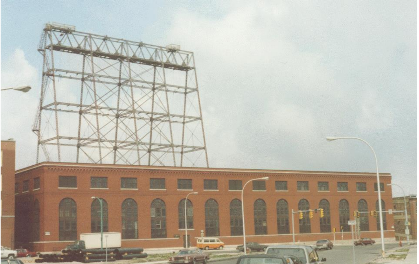
Buffalo General Electric Company Terminal Station B (2008)
