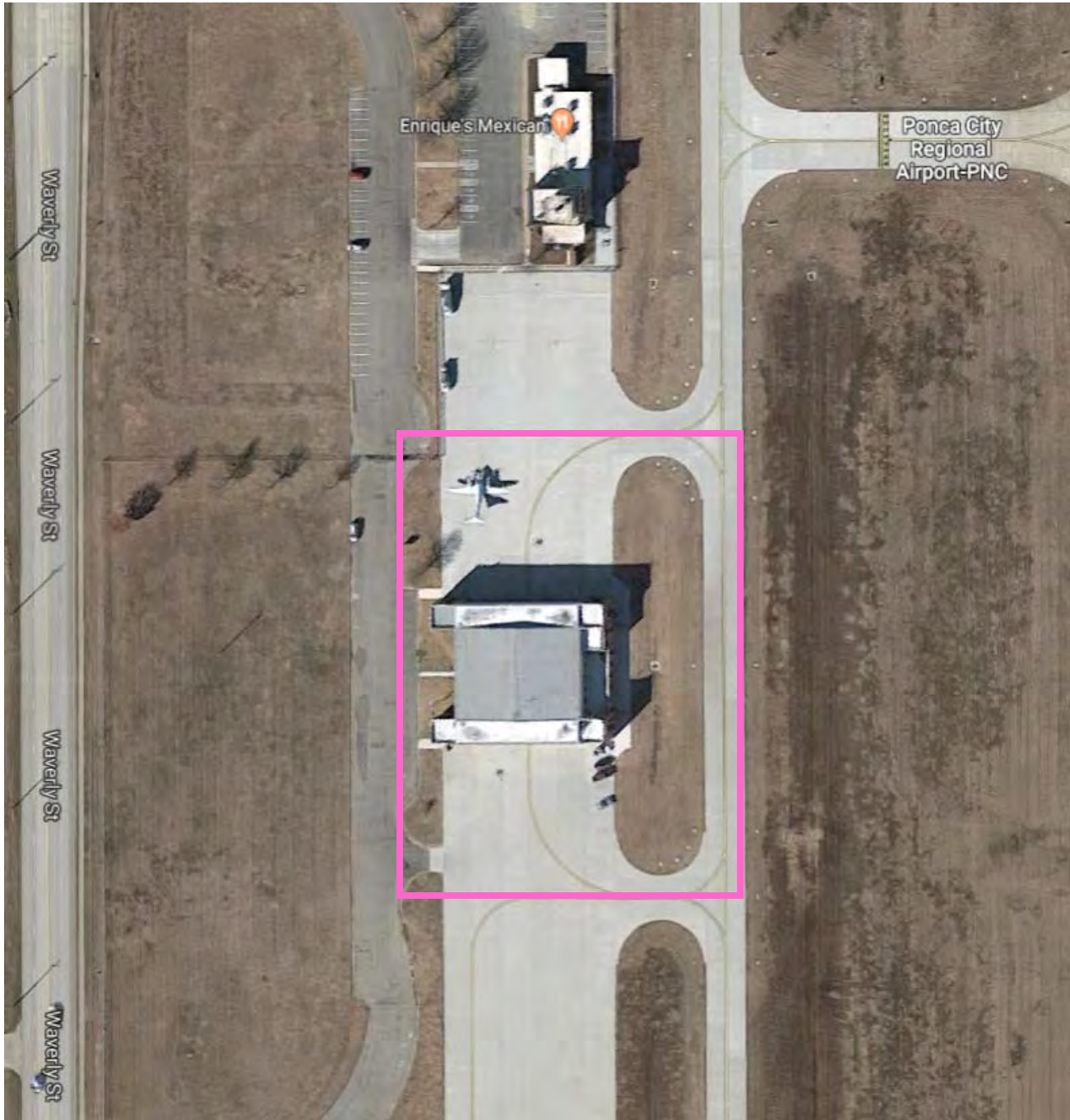
Close-Up: 2018 Ponca City Municipal Airport Aerial
