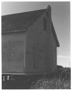
VIEW OF NORTHWEST CORNER, SHOWING CONCRETE BLOCK CHIMMEY AND BOAT HOIST ENGINE EXHAUST PORT
