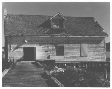
VIEW OF SOUTHSIDE, SHOWING DORMER WINDOW, DOUBLE EQUIPMENT DOOR AND WOODEN WALKWAY
