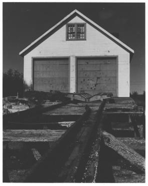
VIEW OF EASTSIDE, SHOWING BOAT LAUNCHWAY, DOUBLE RAILS DECKING, BOAT LAUNCH CRADLE AND OVERHEAD BOAT DOORS
