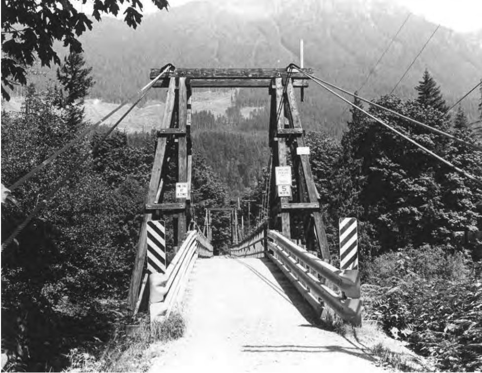
Baring Bridge South Tower 1979, King County Historic Preservation Program
