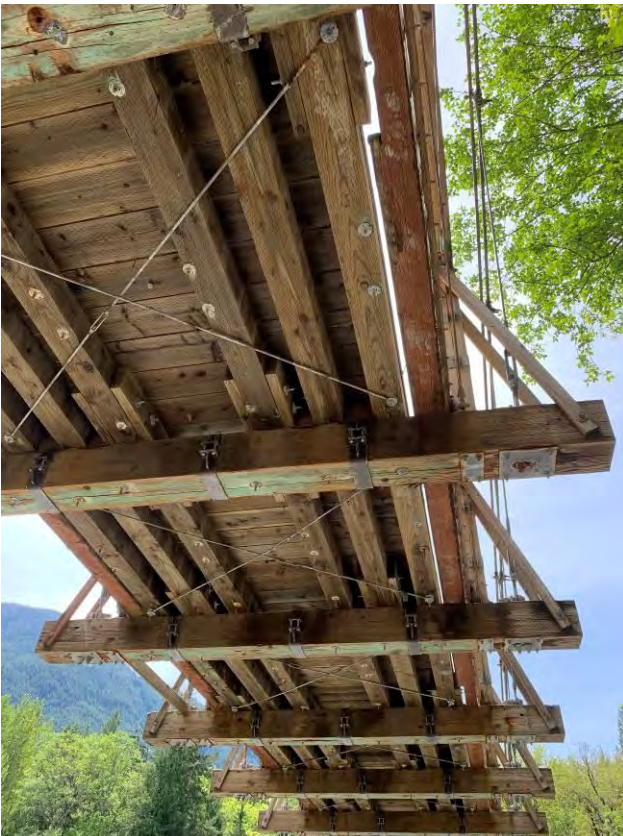
9 of 10: Baring Bridge – Underside of bridge deck
