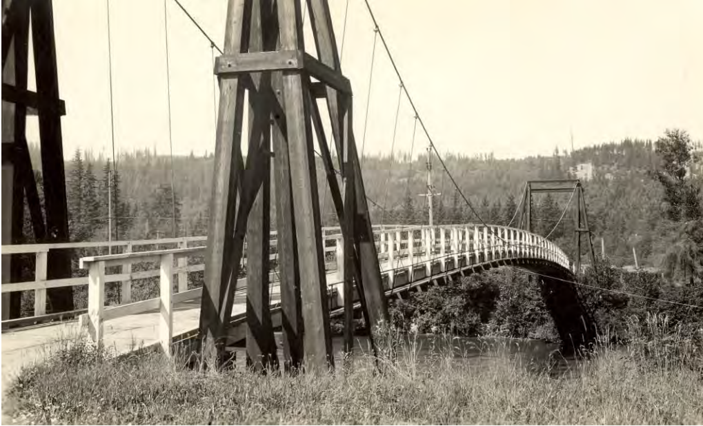
Tarr Bridge: Snoqualmie River, July 26, 1932. - demolished (Series 474, Bridge Number 61F. Section 24, Township 24N, Range 7E.)
