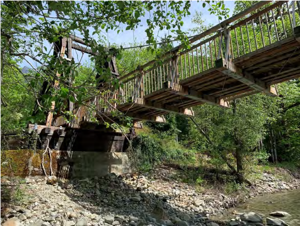
10 of 10: Baring Bridge – North tower from riverbed
