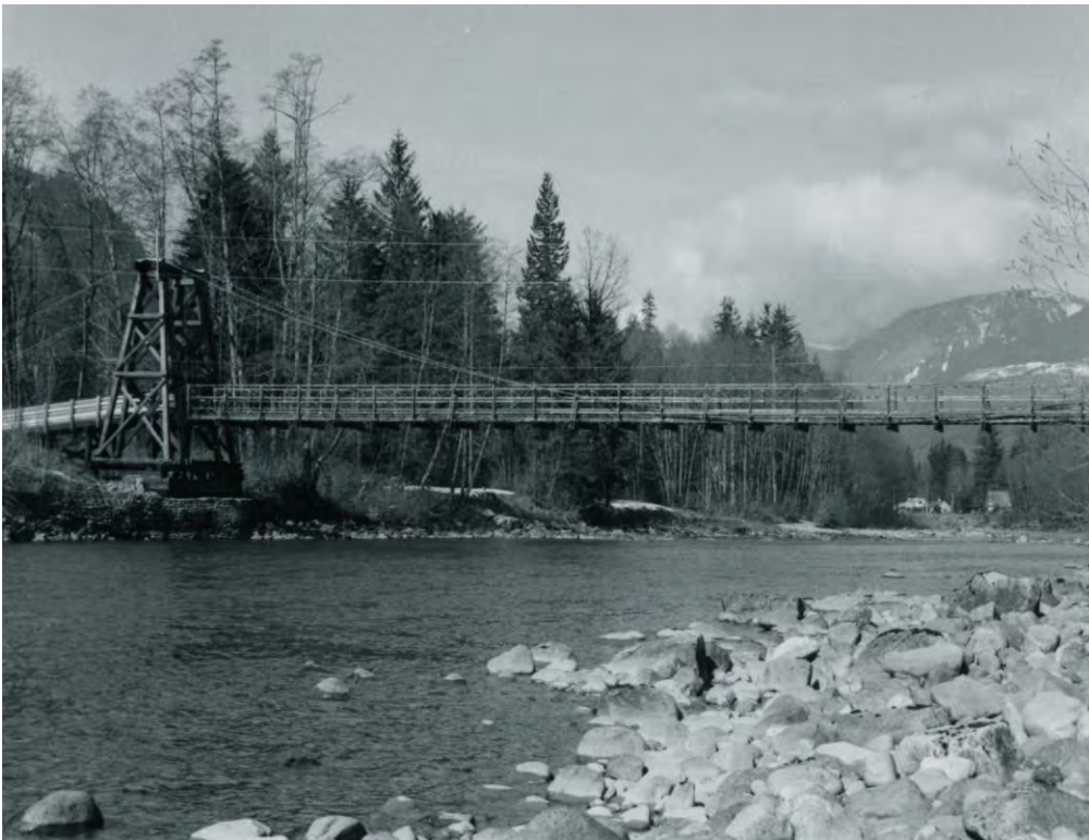
Baring Bridge 1951, King County Archives
