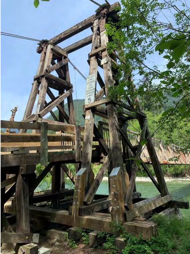
6 of 10: Baring Bridge – South tower detail
