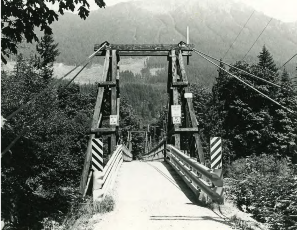
Baring Bridge, 1951, King County Archives
