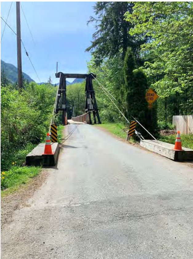
3 of 10: Baring Bridge - North approach, view to south
