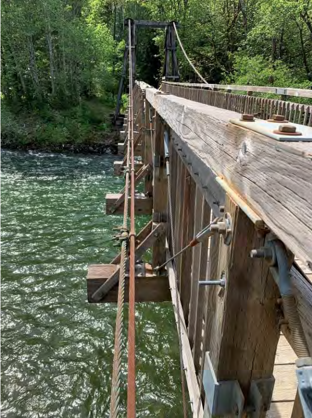
8 of 10: Baring Bridge – Bridge deck, cable and buttress detail
