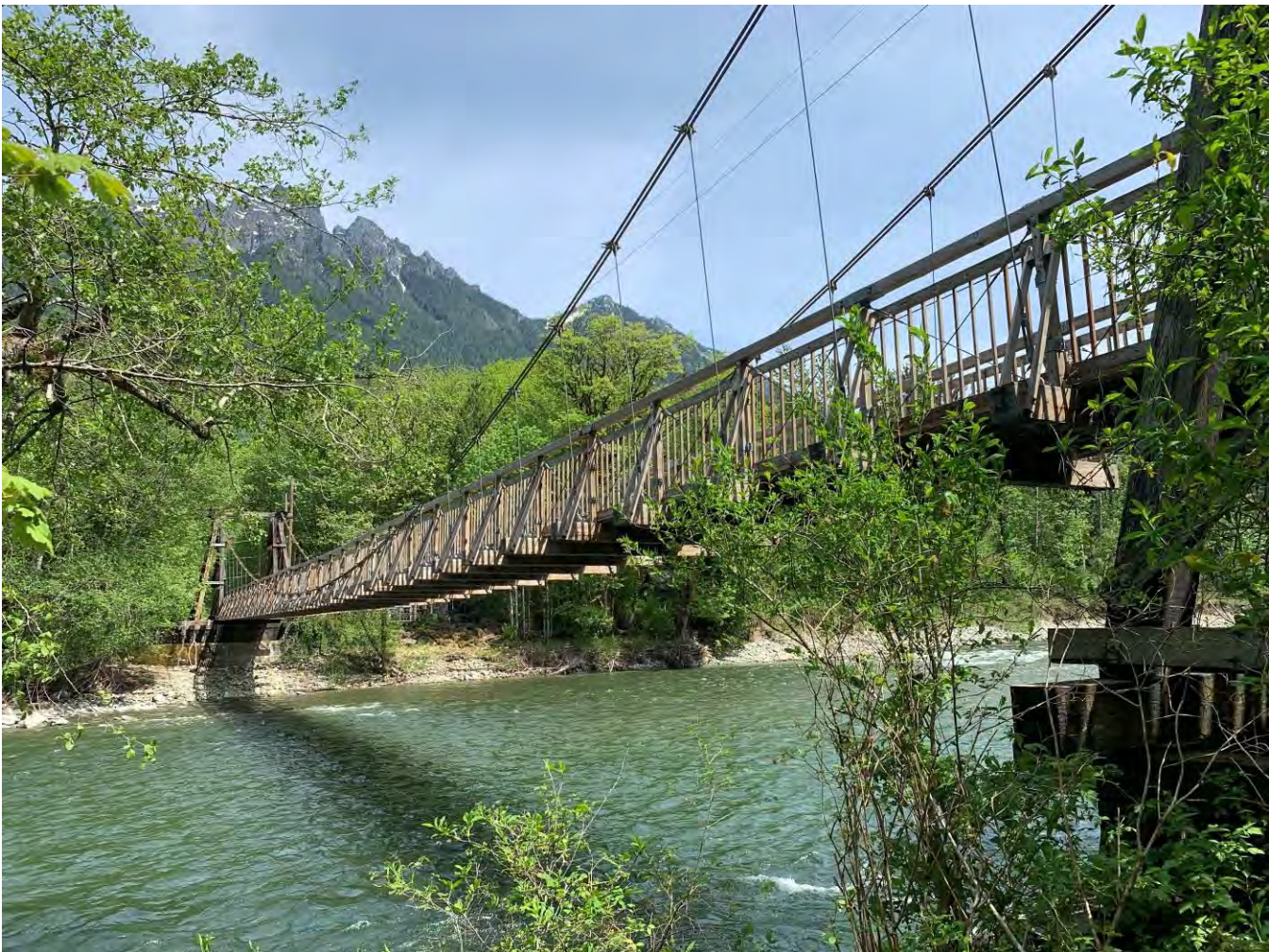
1 of 10: Baring Bridge - View to the north, west side of bridge
