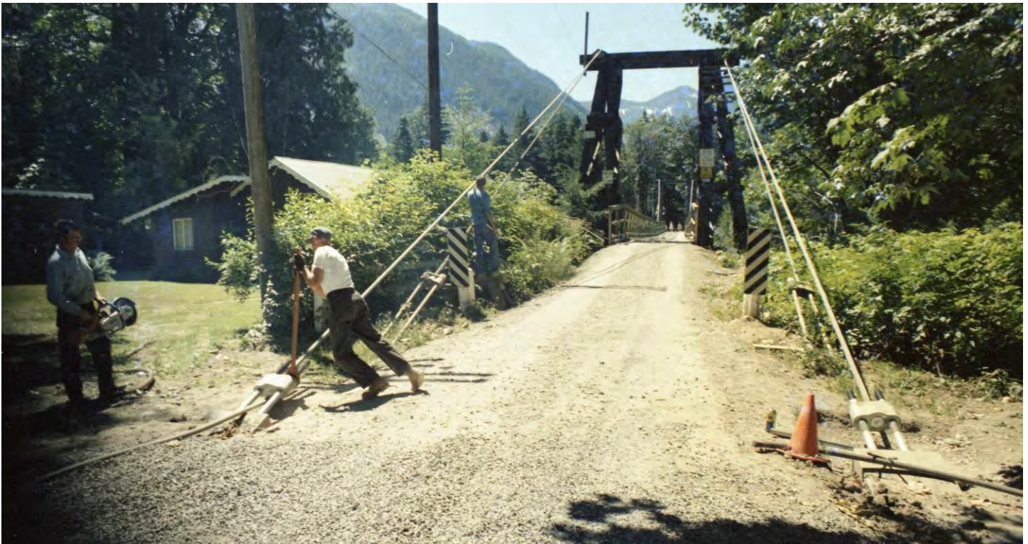
Baring Bridge 1976, Addition of new second cable and North Tower, King County Archives
