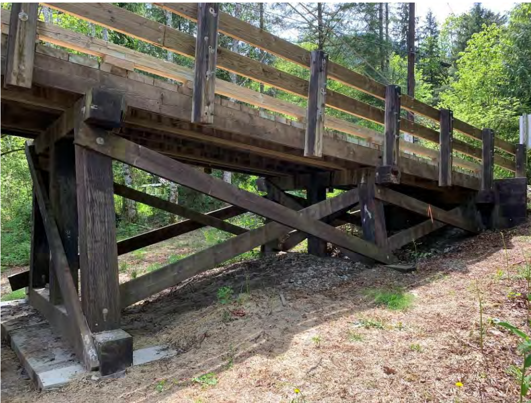
5 of 10: Baring Bridge – South approach detail
