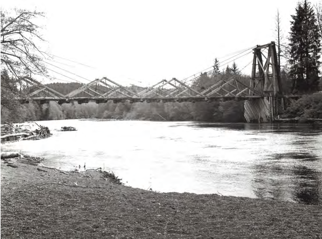
Chow Chow Bridge, Taholah (Built 1952) – demolished
