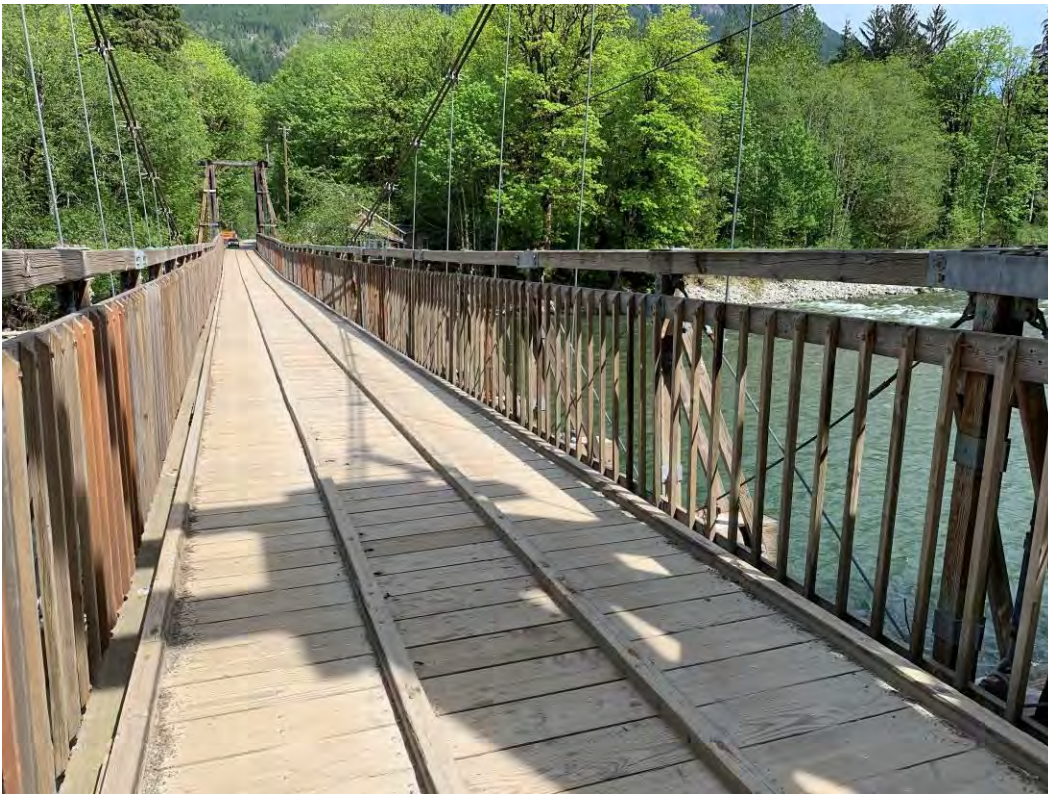
7 of 10: Baring Bridge – Bridge deck detail, view to north
