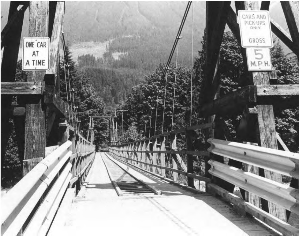
Baring Bridge looking North, 1979, King County Historic Preservation Program
