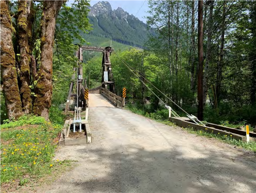
4 of 10: Baring Bridge - South approach, view to the north
