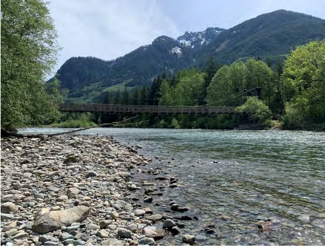
2 of 10: Baring Bridge - View to the east, west side of bridge
