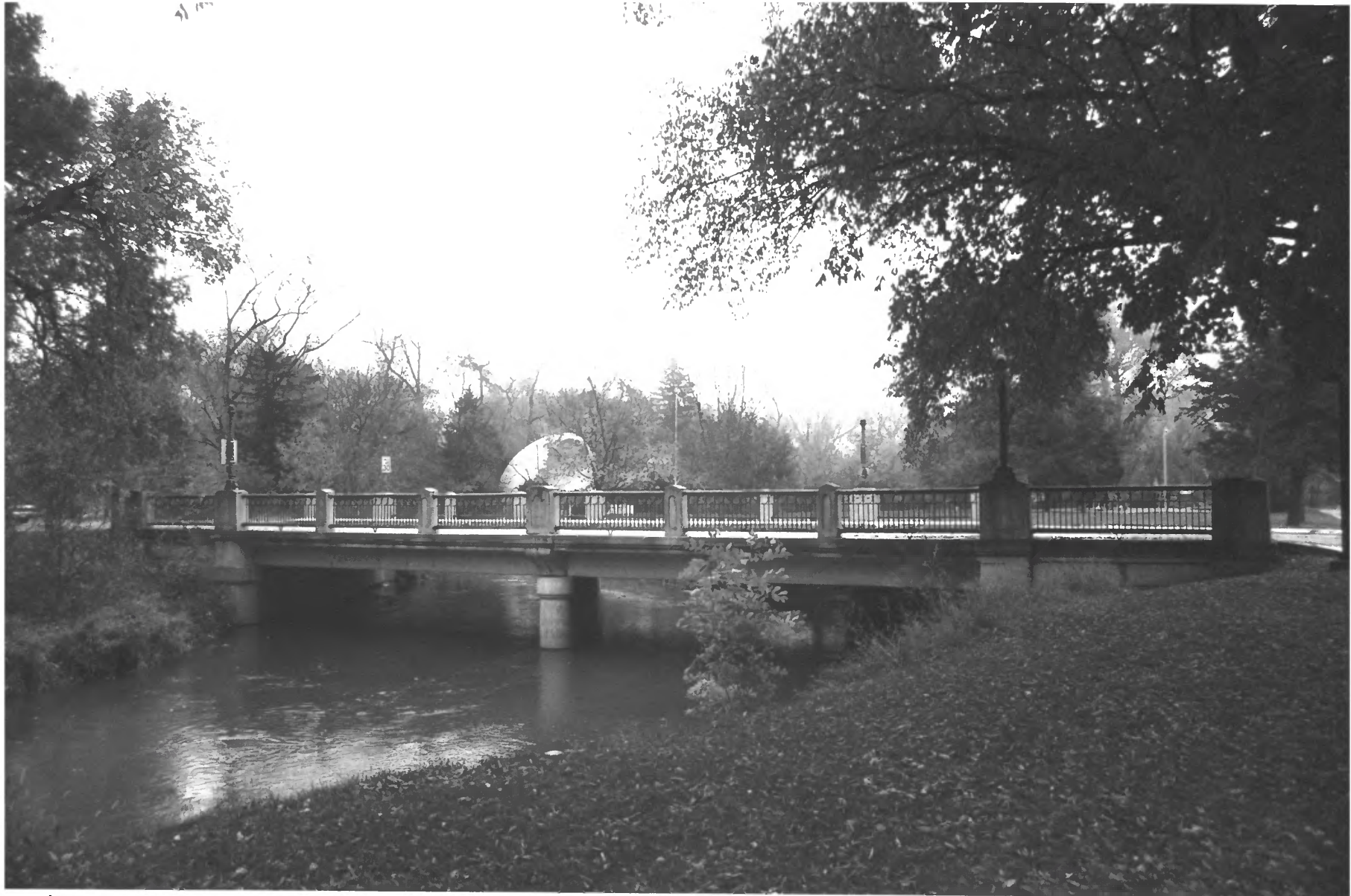
bridge no. 5083 on Highway 19 over Redwood River, Marshall Lyon Co., MN 210684-3
