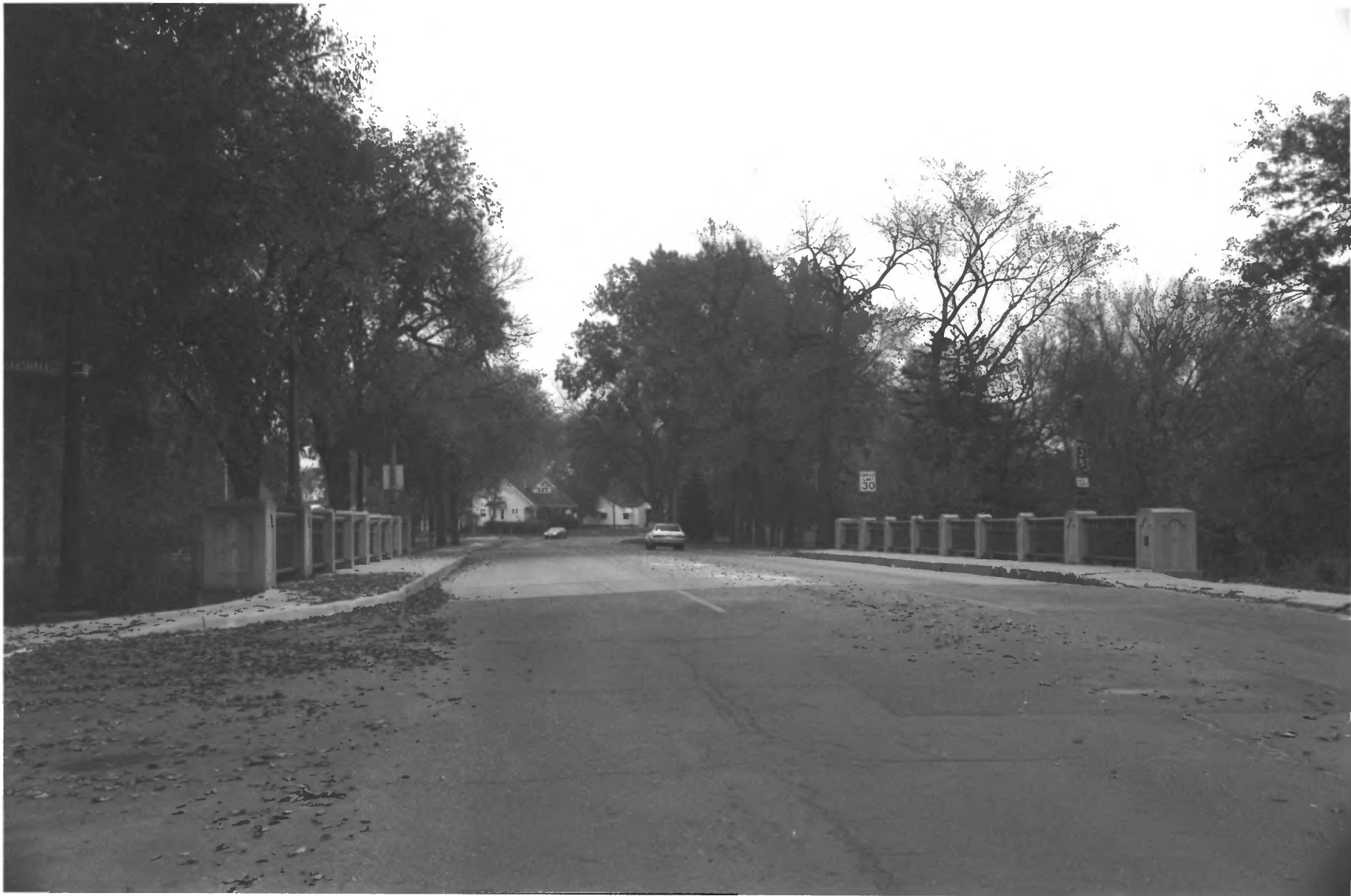
Bridge no. 5083 Mn Highway 190 over Redwood River, Marshall Lyon Co., Mn 012684-4
