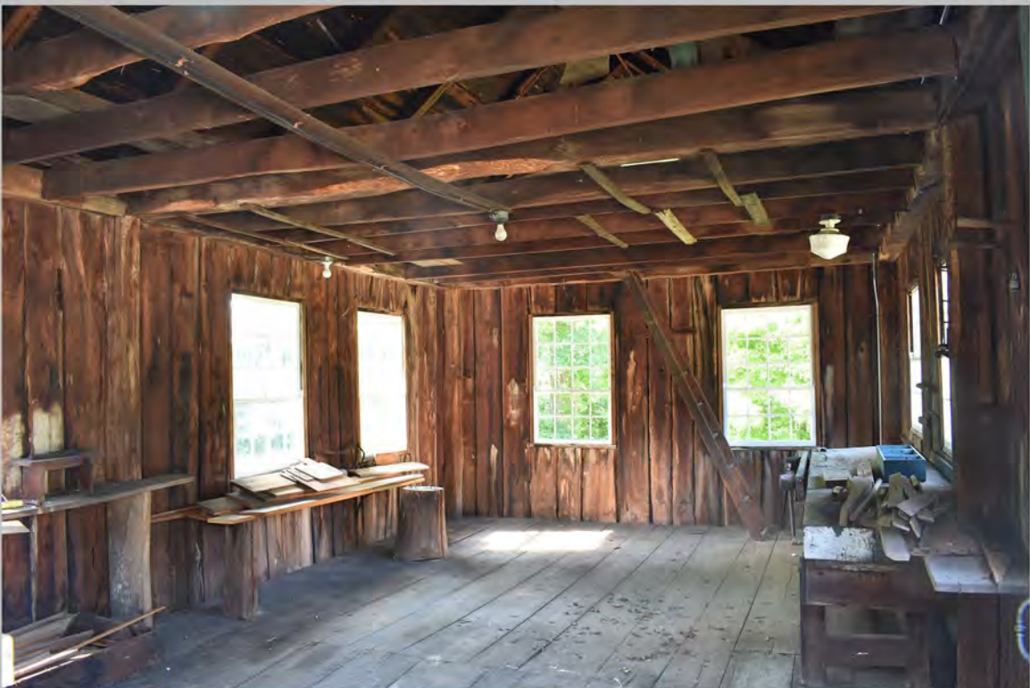
4. Interior view of the first floor of the Olney Cook Artisan Shop showing glazing workspace, looking south from north corner.
