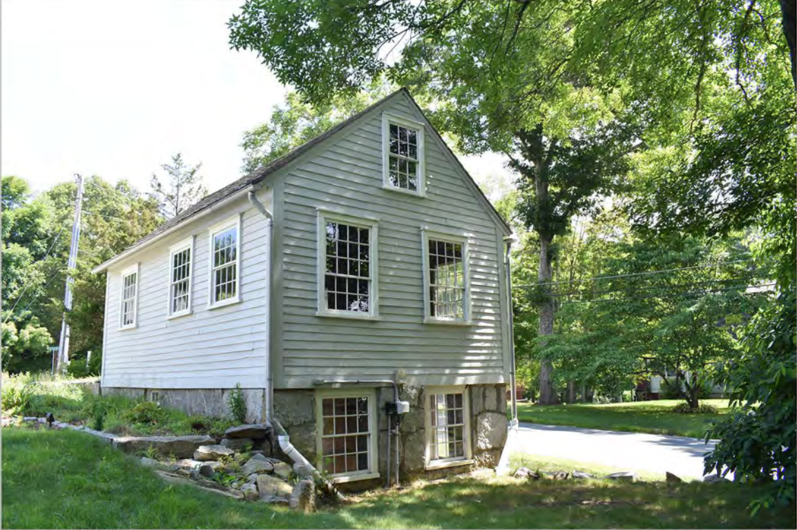
3. General view of Olney Cook Artisan Shop showing southwest and northwest elevations, looking east.
