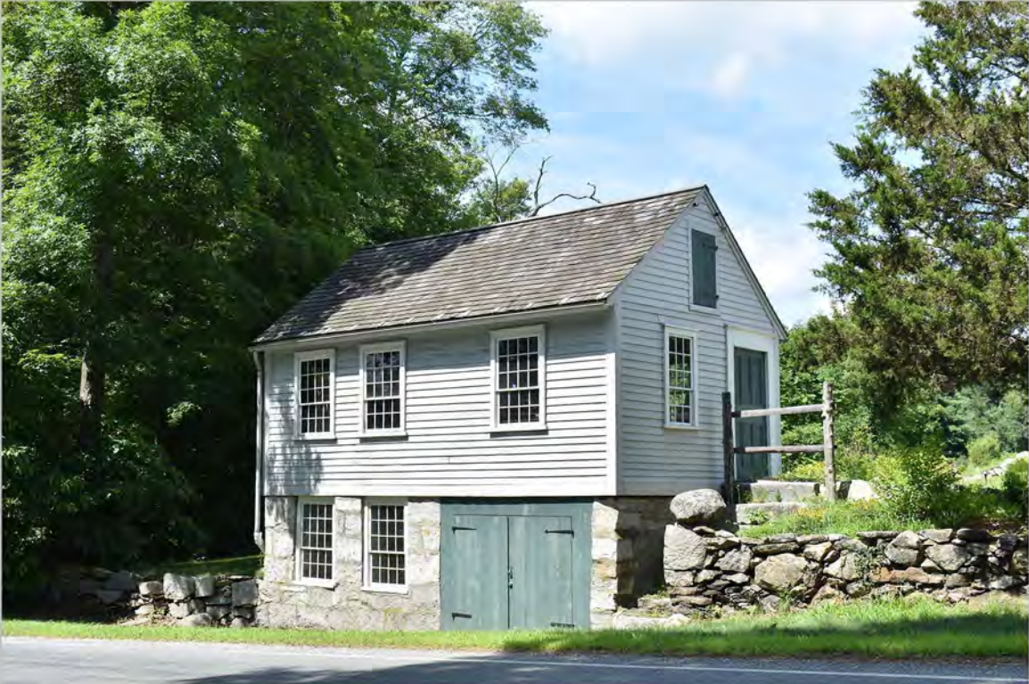
1. General view of Olney Cook Artisan Shop showing northeast and southeast elevations, looking west from Hartford Avenue East.
