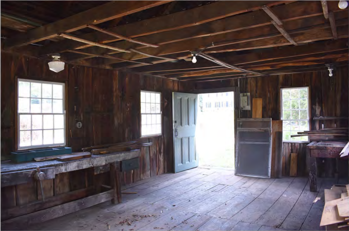
5. Interior view of the first floor of the Olney Cook Artisan Shop showing glazing workspace, looking north from south corner.
