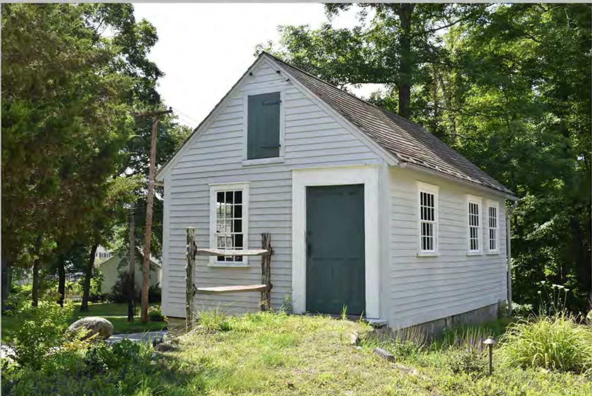
2. General view of Olney Cook Artisan Shop showing northeast and northwest elevations, looking south from property parking area.
