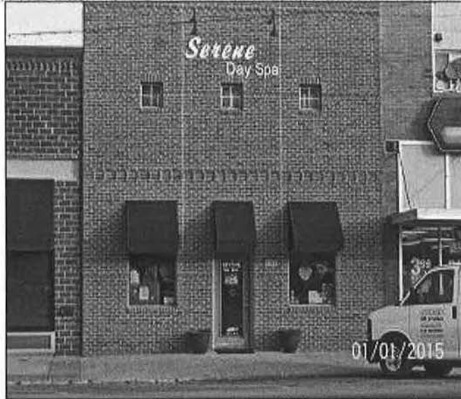
Figure 78: 131 West Washington Street (Clarke County Assessor, 2015)
