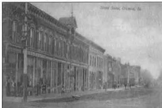
Figure 100: Looking southwest, ca.1916 (Osceola Main Street)
