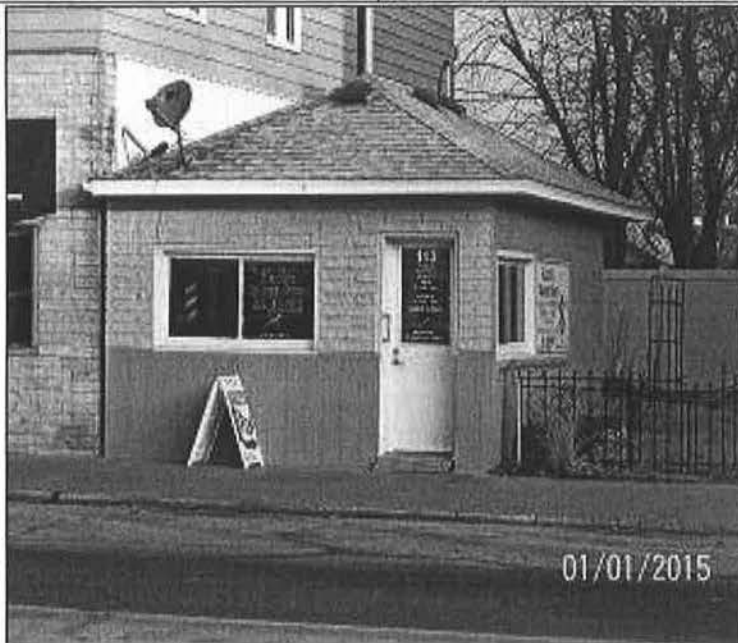
Figure 69: 113 West Washington Street (Clarke County Assessor, 2015)
