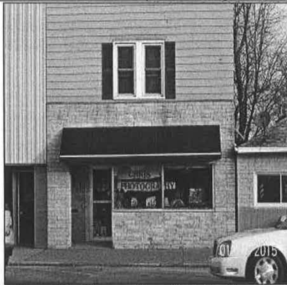
Figure 70: 115 West Washington Street (Clarke County Assessor, 2015)
