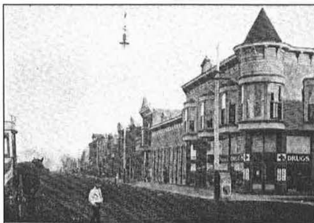
Figure 101: Looking southeast, ca.1916
