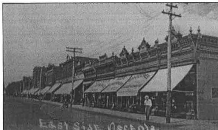
Figure 110: Looking northeast, ca.1910, the row of metal-clad stores is right of center (Naumann)
