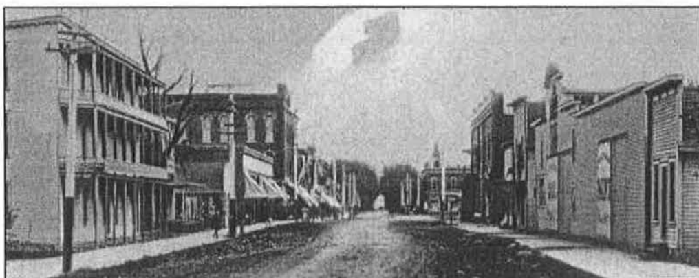
Figure 102: North Main Street, looking south, ca.1910 (Osceola Main Street)
