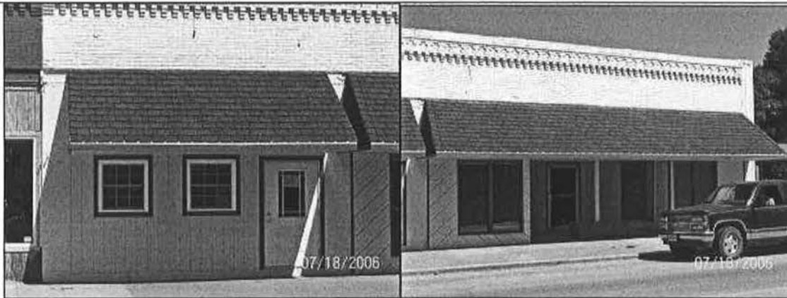
Figures 37-38: 113-15-17 North Main Street (north end of frontage is at the left) (Clarke County Assessor)
