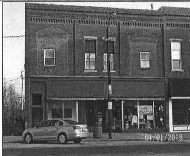
Figure 68: 103-05 West Washington Street (Clarke County Assessor, 2015)
