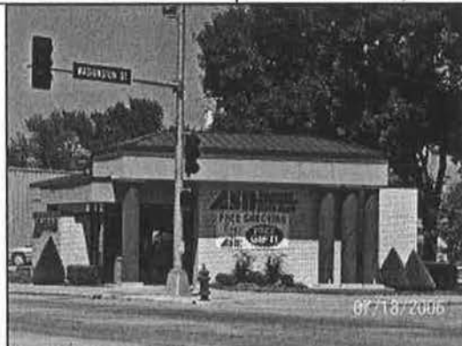
Figure 35: 101 North Main Street (Clarke County Assessor)
