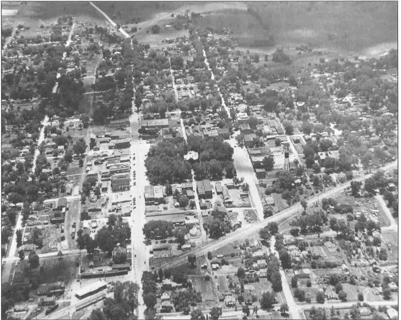
Figure 91: Aerial view looking south, 1931 (State Historical Society of Iowa, State Archives, Cities and Towns, Des Moines Register photo, 1931)
