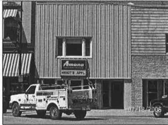
Figure 71: 117 West Washington Street (Clarke County Assessor, 2006)
