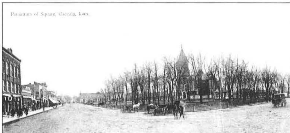
Figure 104: Pre-1912 panoramic view, east portion, looking south and southwest ( https://digital.grinnell.edu/islandora/object/grinnell:16430 )
