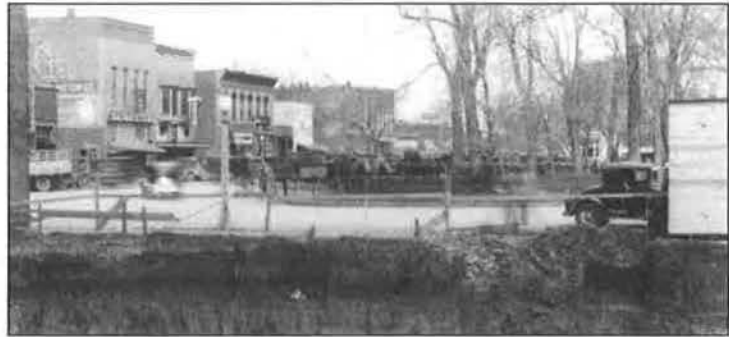
Figure 112: Looking northwest from post office construction site, 1935, note the movie house marquee on 127-129 West Washington (Courtesy of the local postmaster)
