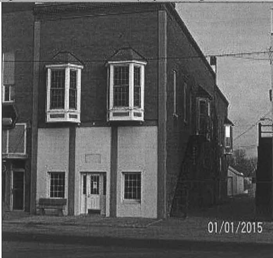
Figure 75: 127 West Washington Street (Clarke County Assessor, 2015)
