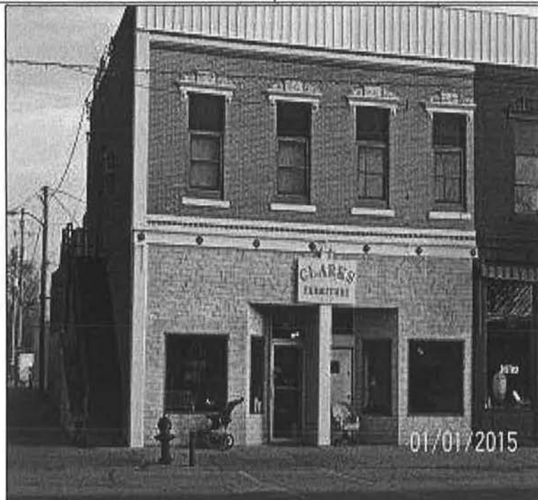
Figure 74: 121-23 West Washington Street (Clarke County Assessor, 2015)
