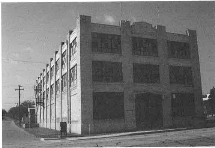
Figure 5: The Parker-Browne Company Building, 1212 E. Lancaster Ave., constructed in 1924. It is an example of an industrial/warehouse building on Fort Worth's Near Southside built using a reinforced concrete grid pattern but was constructed in a more refined style and nine years after the Fort Worth Warehouse & Transfer Company Building.
