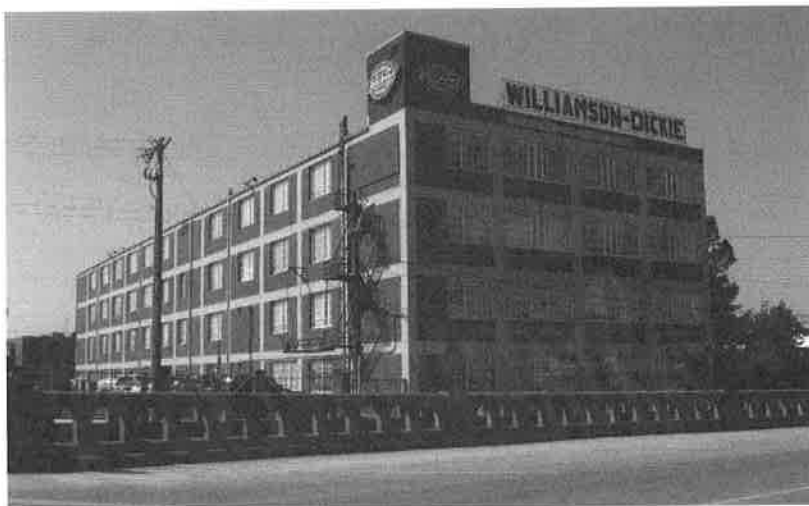
Figure 6: Williamson-Dickie Company Building, 509 W. Vickery Blvd., located approximately seven blocks west of the Fort Worth Warehouse & Transfer Co. Building. It was constructed in 1924 and is an example of a warehouse/industrial building that uses a reinforced concrete grid pattern as structural support. All original windows have been replaced. Its larger window openings were beneficial to its function as a garment factory. Such windows were not necessary for the Fort Worth Warehouse & Transfer Company Building's function as a storage facility.
