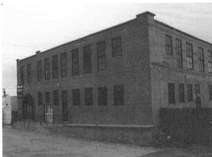
Figure 4: Miller Manufacturing Company Building, 311 Bryan Avenue, was constructed in 1911 and is an example of an early reinforced concrete industrial building constructed in the Near Southside of Fort Worth (and one block from the Fort Worth Warehouse & Transfer Company Building). It was listed in the National Register of Historic Places in 2010 for its architectural and historic significance.
