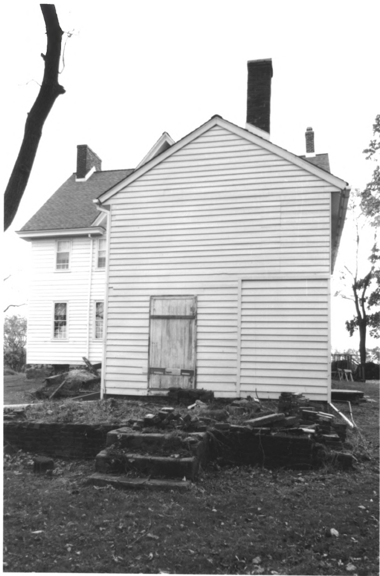
INSKEEP HOUSE, BURLINGTON CO., N.J., PHOTO # 4
