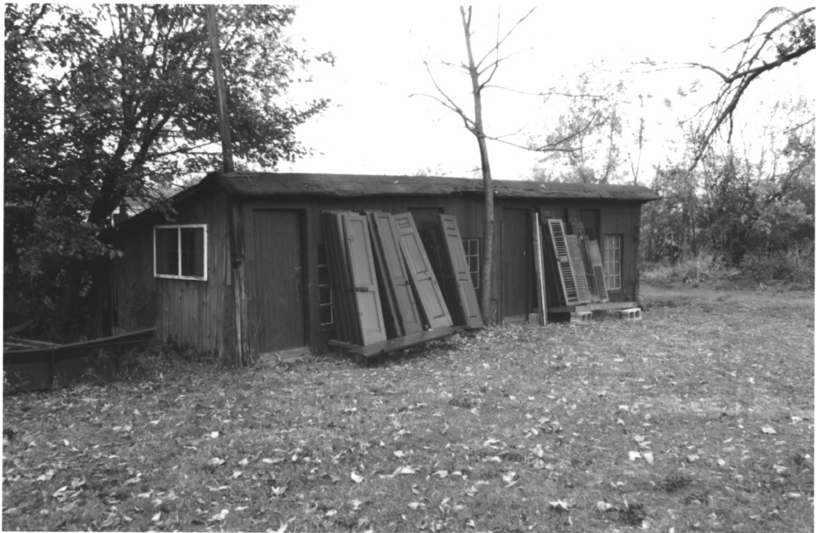
INSKEEP HOUSE, BURLINGTON CO. N.J., PHOTO # 10
