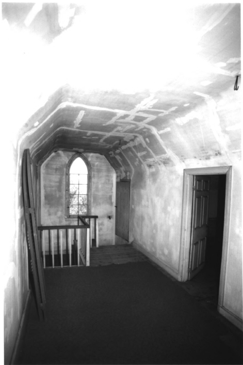
INSKEEP HOUSE, BURLINGTON CO. N.J., PHOTO # 8
