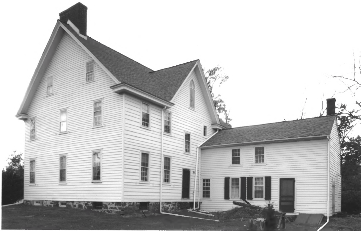
INSKEEP HOUSE, BURLINGTON CO. N.J., PHOTO # 3
