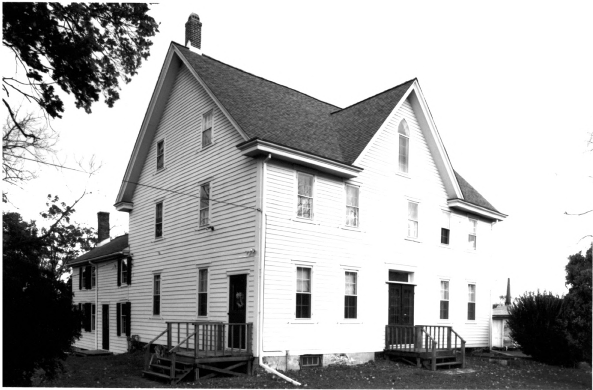
INSKEEP HOUSE, BURLINGTON CO. N.J., PHOTO # 2
