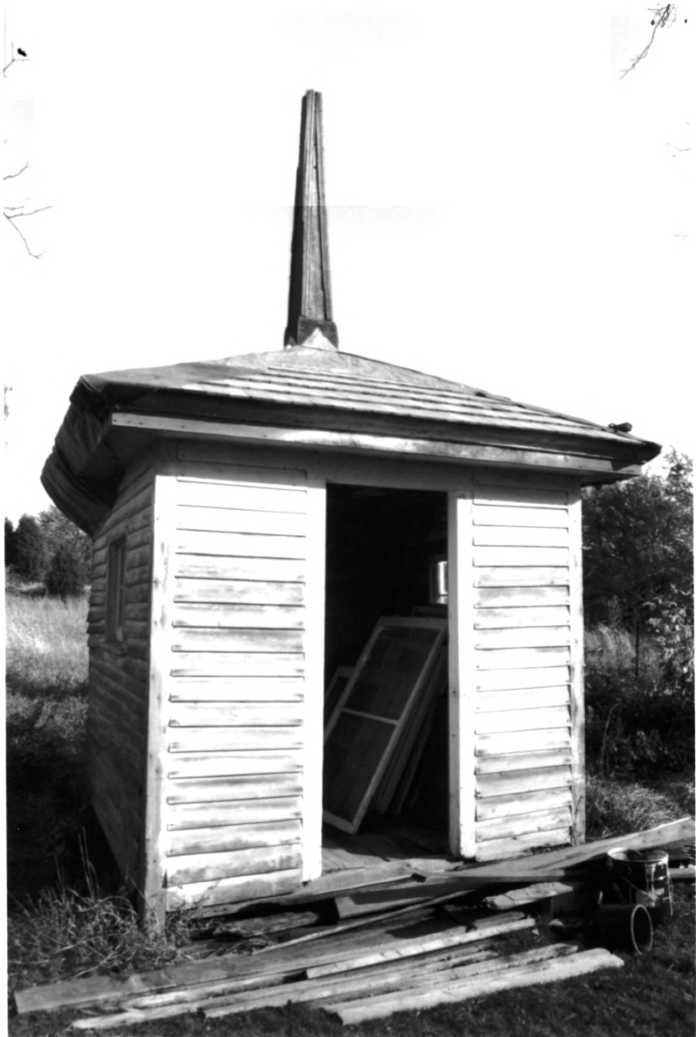
INSKEEP HOUSE, BURLINGTON CO. N.J., PHOTO # 9
