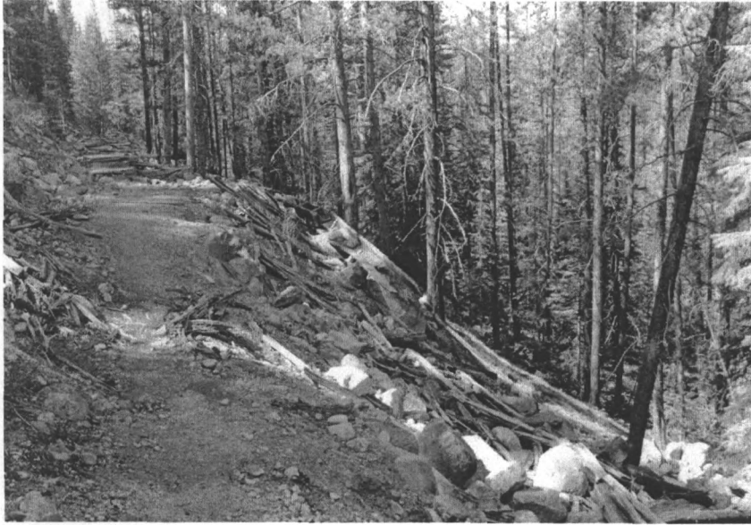
Photo #33 Structure #140, road, and Site #97, flume View to N
