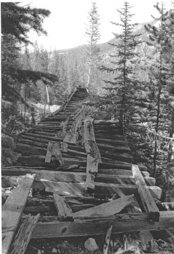
Photo #34 Structure #100, trestle View to N
