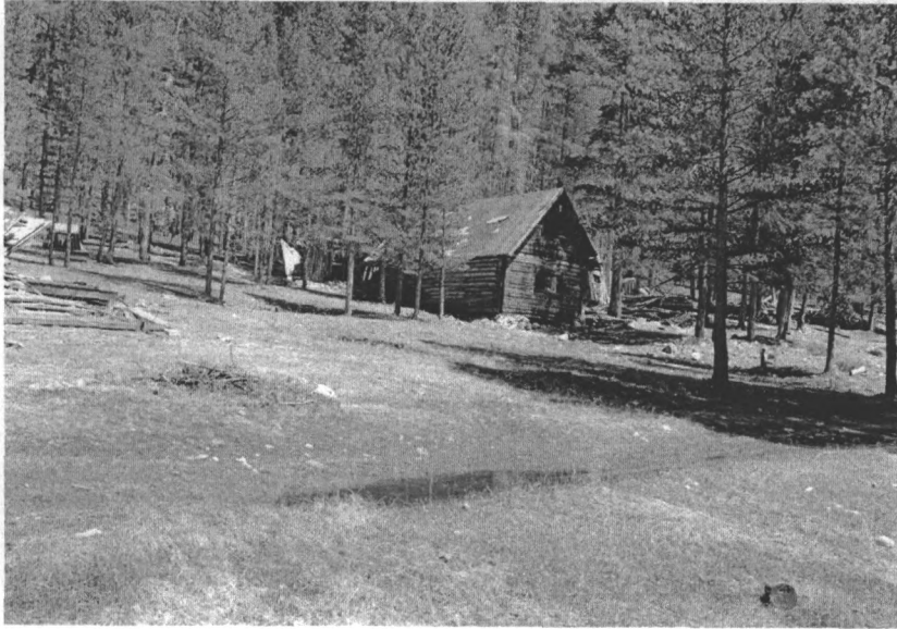
Photo #19 Building #44 View to SE
