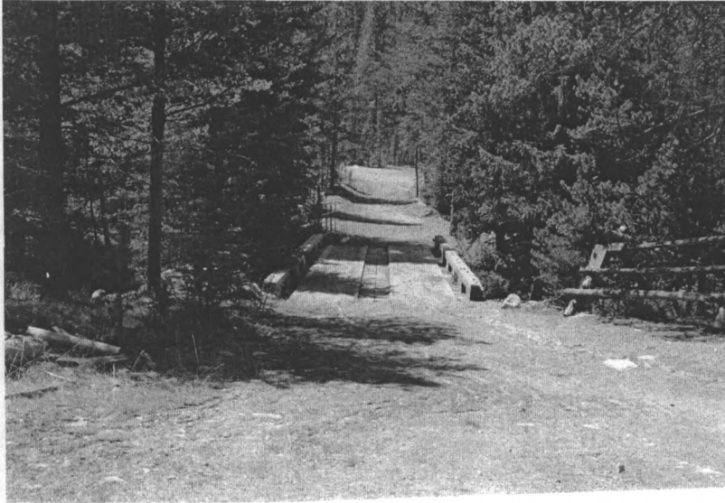
Photo #9 Structure #125, stringer bridge View to W
