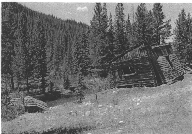
Photo #8 Building #9, shiplap building View to NW
