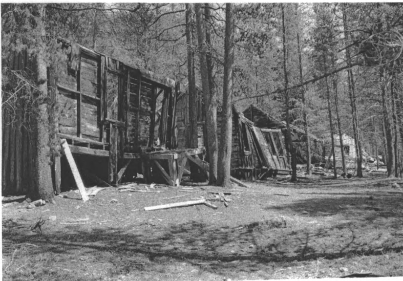
Photo #22 Site #s 60, 63, and 64 View to SE
