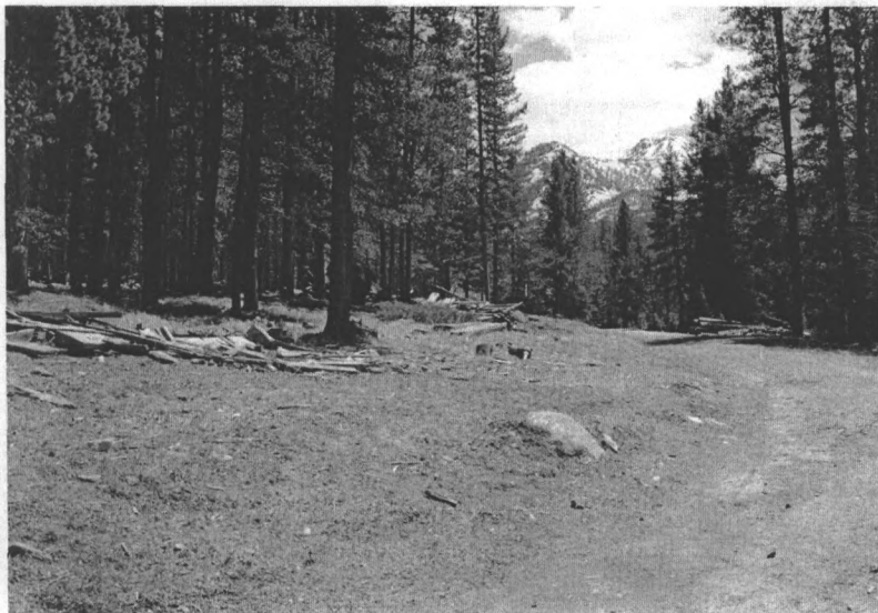
Photo #7 Site #7, collapsed wood-frame building View to S
