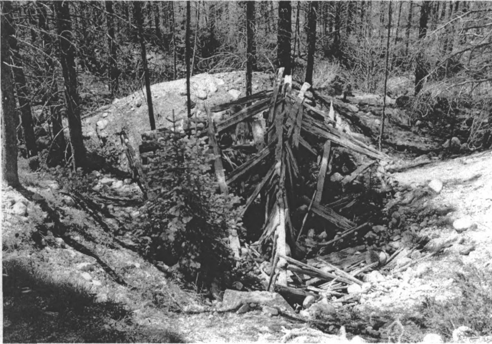
Photo #1 Site #1 partially collapsed dugout View to W
