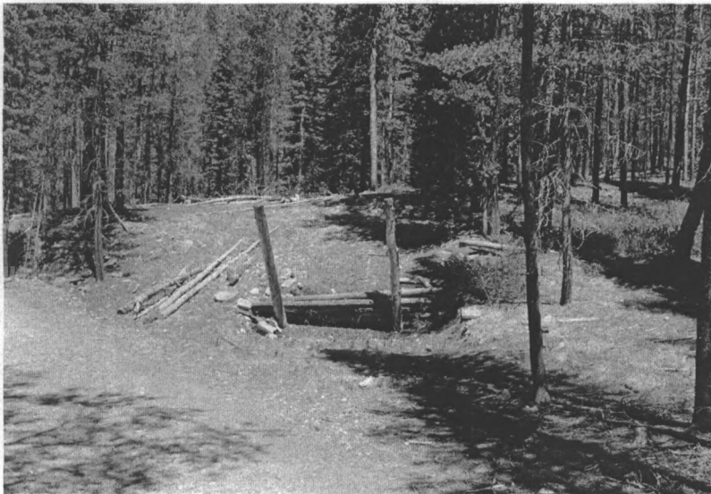
Photo #6 Structure #123, loading dock View to NE
