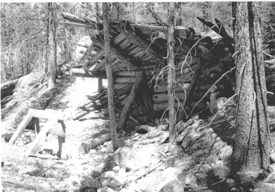
Photo #2 Site #2 collapsed log cabin View to N
