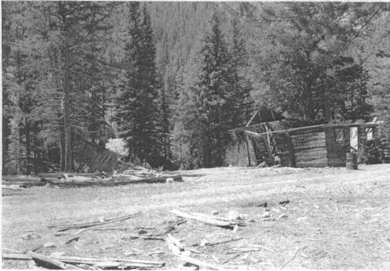
Photo #13 Site #s 19, wood-frame cabin, and 20, pumphouse, View to NW
