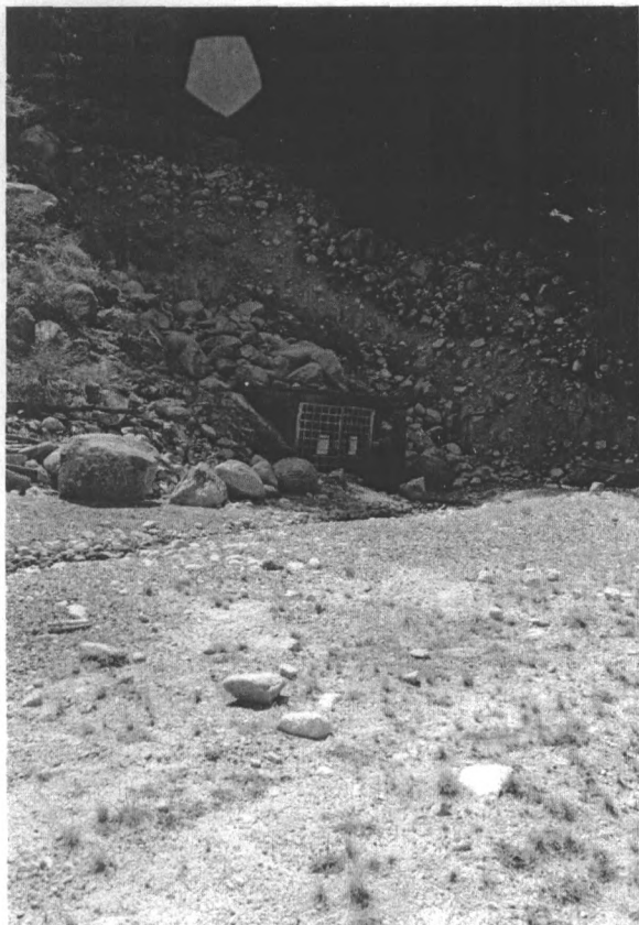
Photo #28 Structure #91, c. 1950s lower portal mine adit View to W
