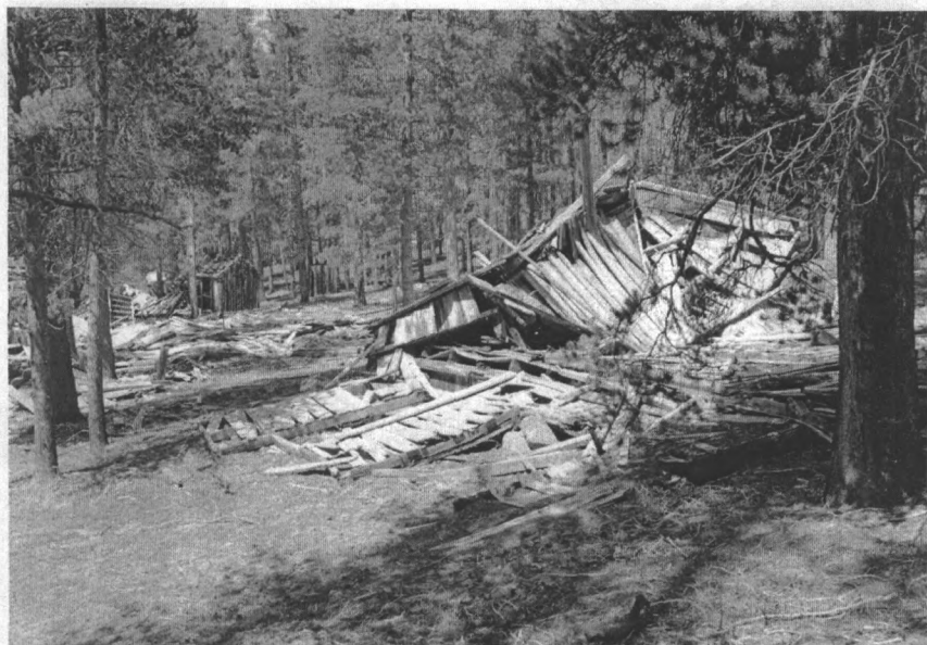
Photo #23 Site #s 64, 66, 67, and 72 View to NE
