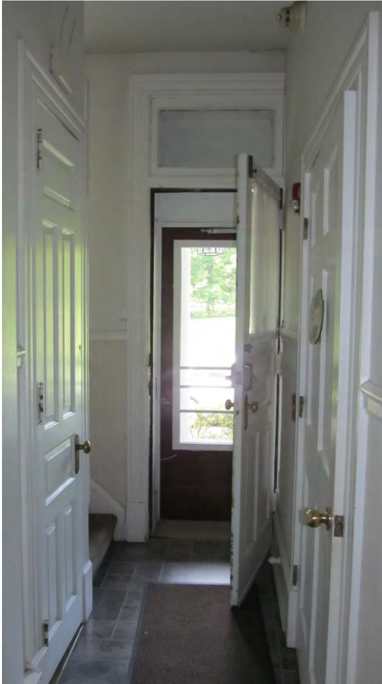
Photo 18. First floor, rear corridor
