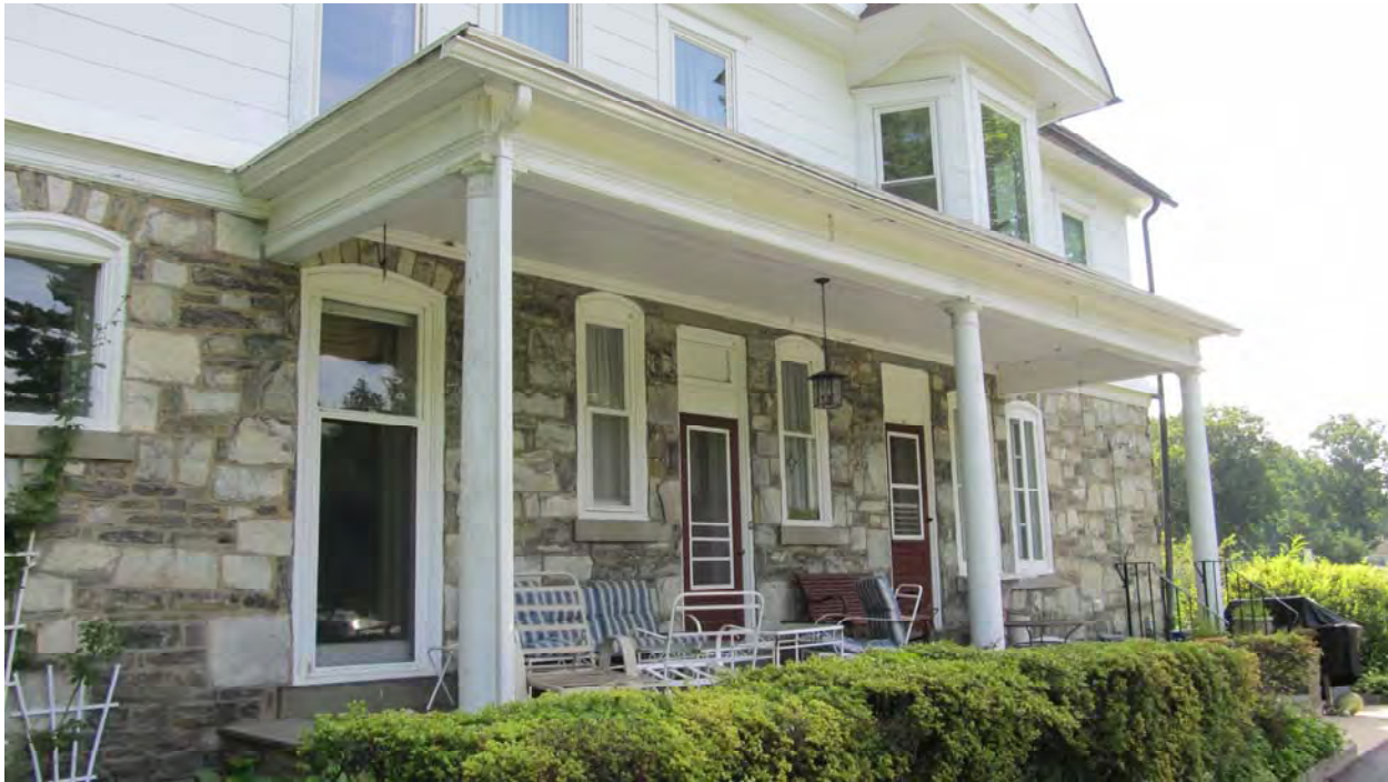
Photo 5. Detail of porch on south elevation, looking northeast
