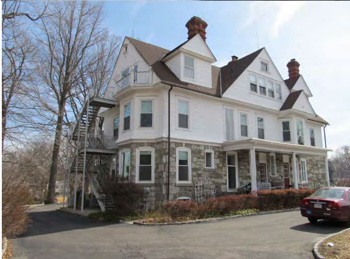
Figure 1. Mill-Rae, west and south elevations, c. 1908 (above) and in 2015 (below). Top photo from Trainer family papers; bottom photo taken in 2015 by nomination author.
