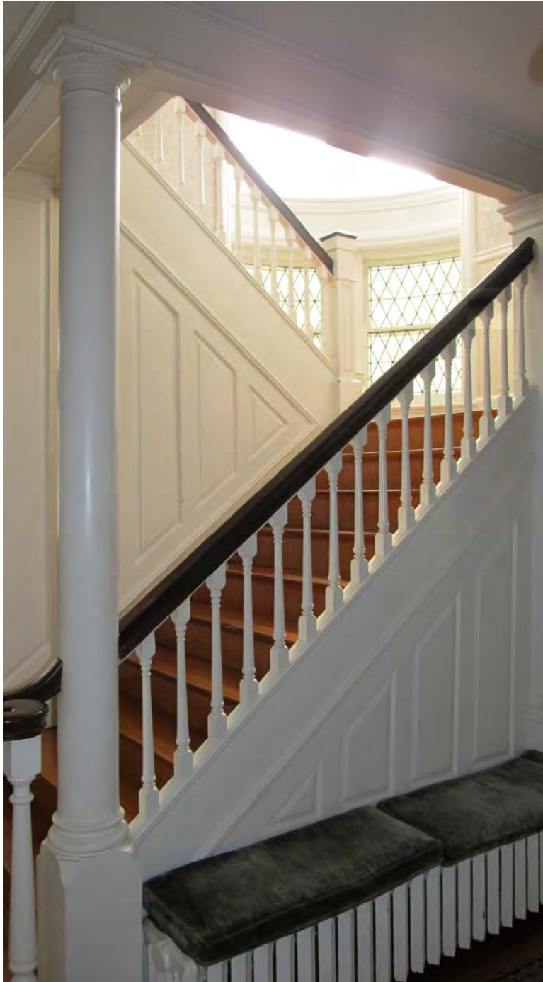
Photo 15. First floor, stair
