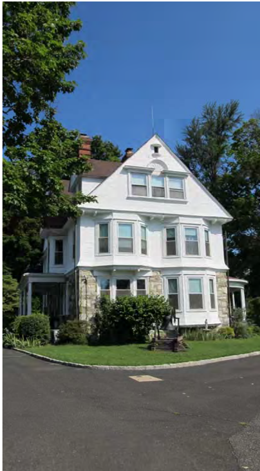
Photo 8. East elevation, looking northwest
