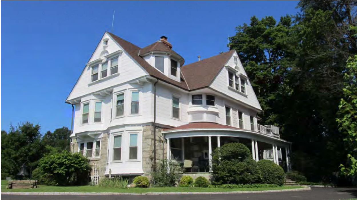
Photo 9. East and north elevations and north porch, looking southwest.
