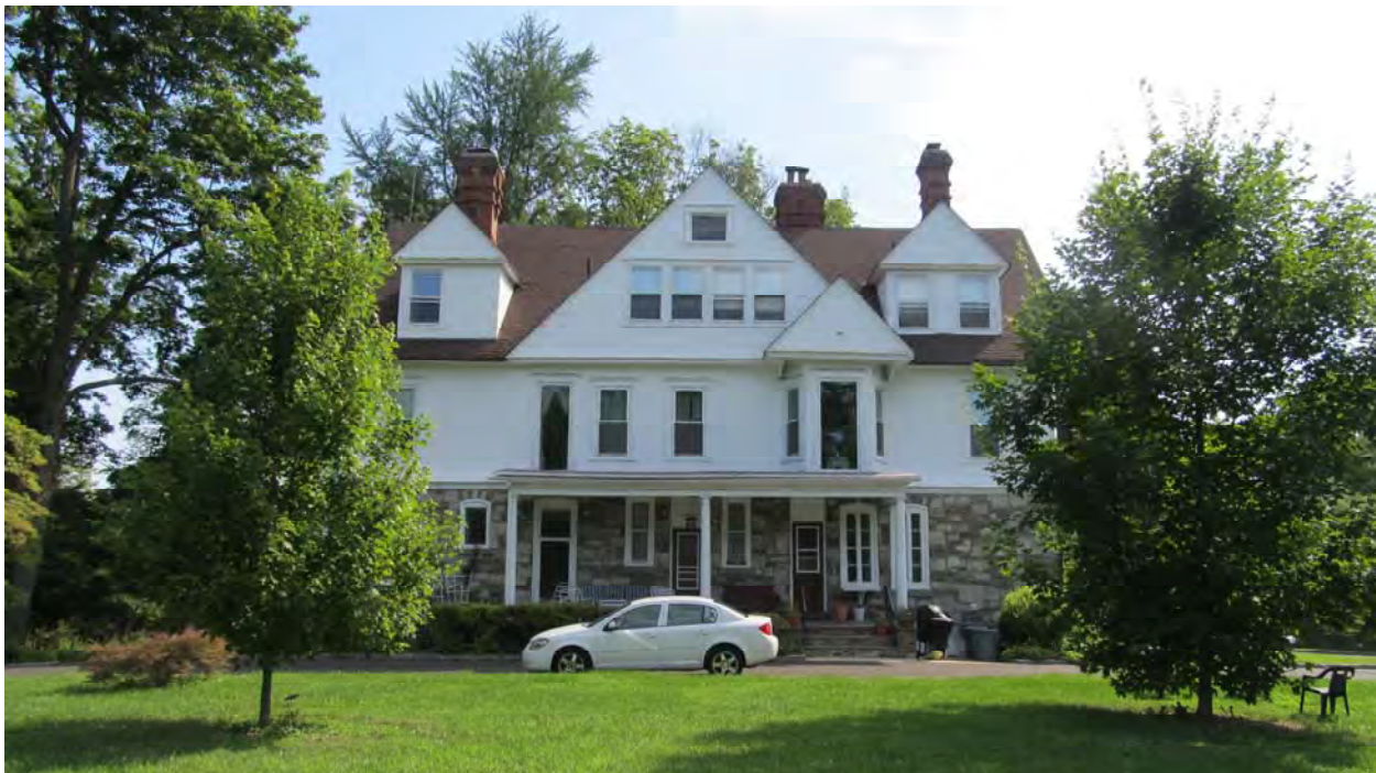
Photo 4. South elevation, looking northeast
