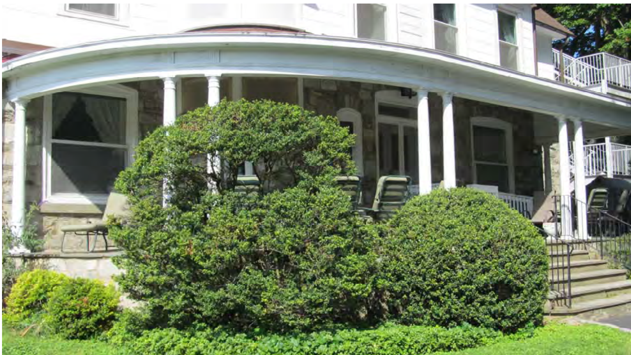
Photo 6. Detail of porch on north elevation, looking southwest
