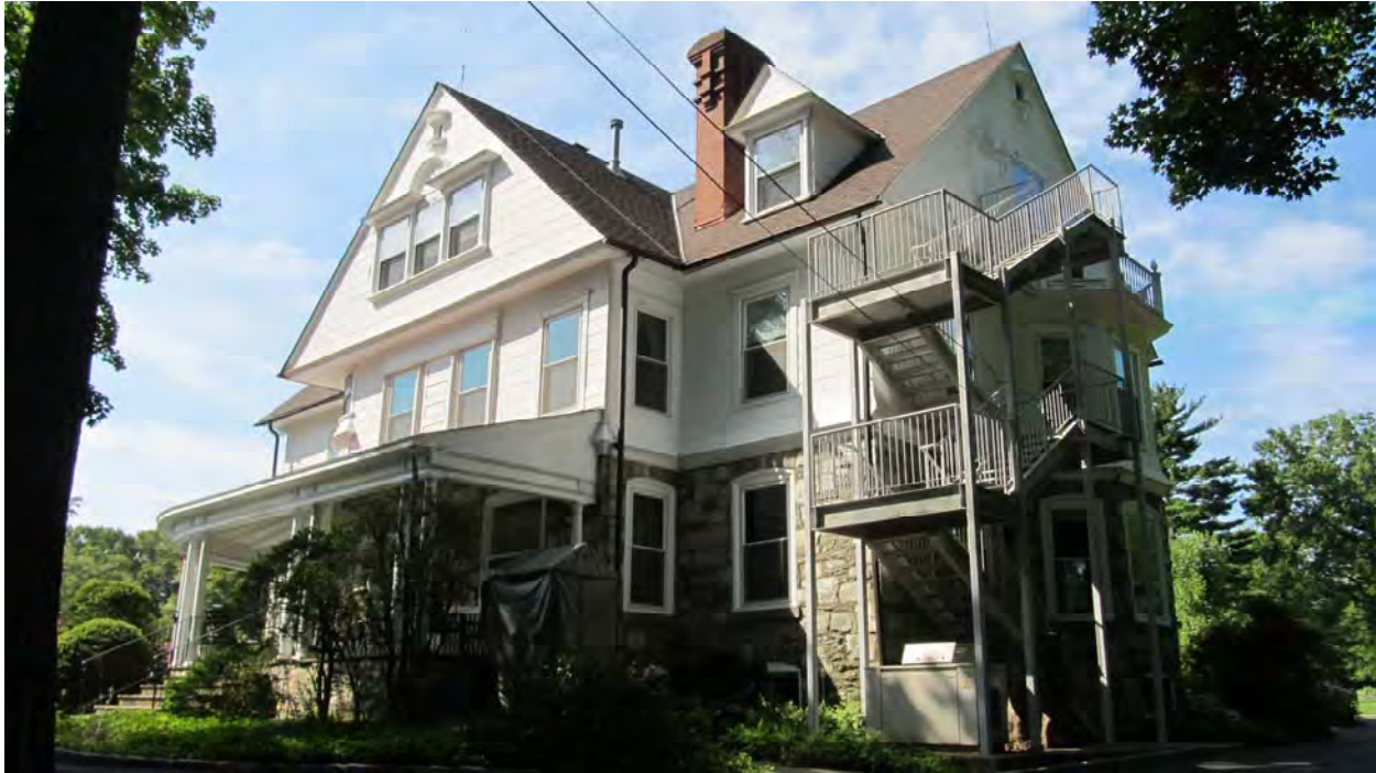
Photo 7. North elevation, looking southwest
