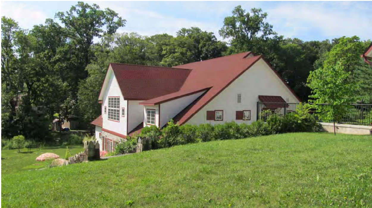
Photo 11. Education and Conference Center building, looking south
