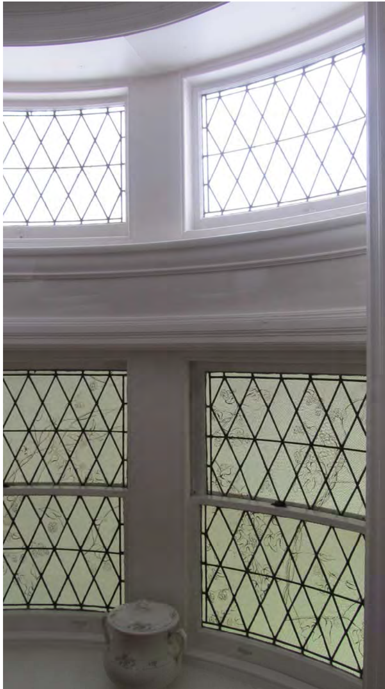
Photo 16. First floor, detail of stair window
