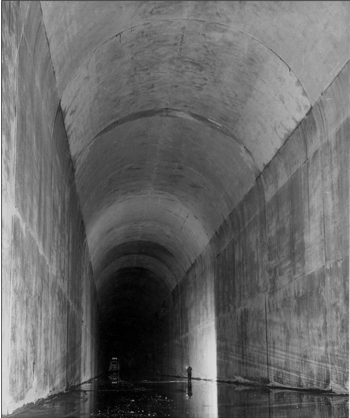
PA7-11192 NIAGARA POWER PROJECT. WATERWAYS-SECTION #1. A WORKMAN IS DWARFED BY 66-FOOT HIGH COMPLETED AND BACKFILLED SECTION OF CONDUIT #2 NEAR PINE AVENUE IN NIAGARA FALLS. CONDUIT IS FORTY-SIX FEET WIDE. POWER AUTHORITY-STATE OF NEW YORK UHL, HALL & RICH-ENGINEERS JANUARY 13, 1960
