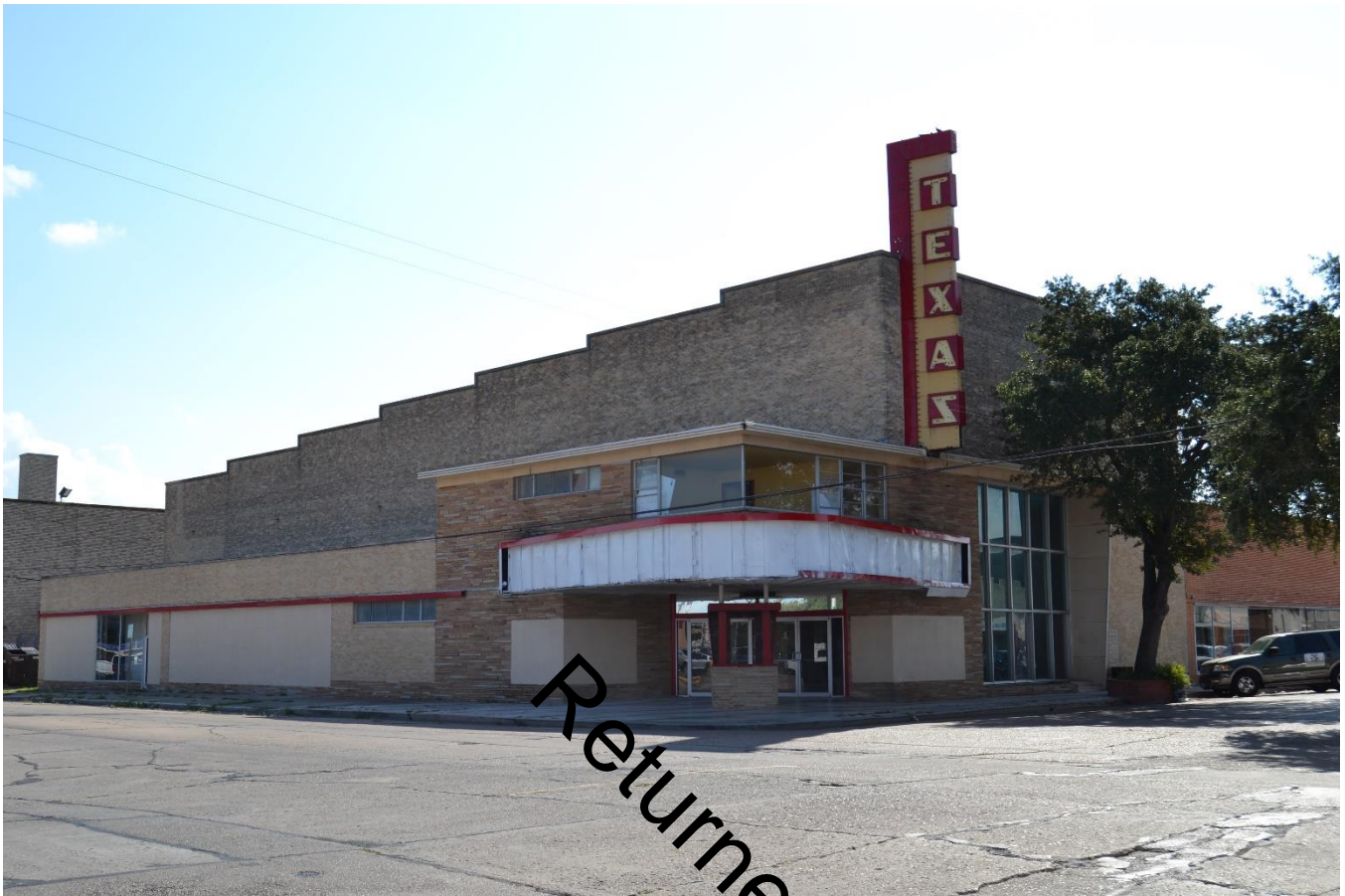
Photo No. 18 (TX_KlebergCounty_KingsvilleDowntownHistoricDistrict_0018) Resource No. 47, 327 East Kleberg Avenue, oblique view of the Texas Theater, view facing southwest.
