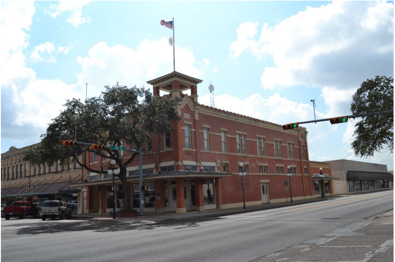
Photo No. 12 (TX_KlebergCounty_KingsvilleDowntownHistoricDistrict_0012) Resource No. 21, 201 East Kleberg Avenue, oblique view of John B. Ragland Mercantile Company Building, view facing southeast.
