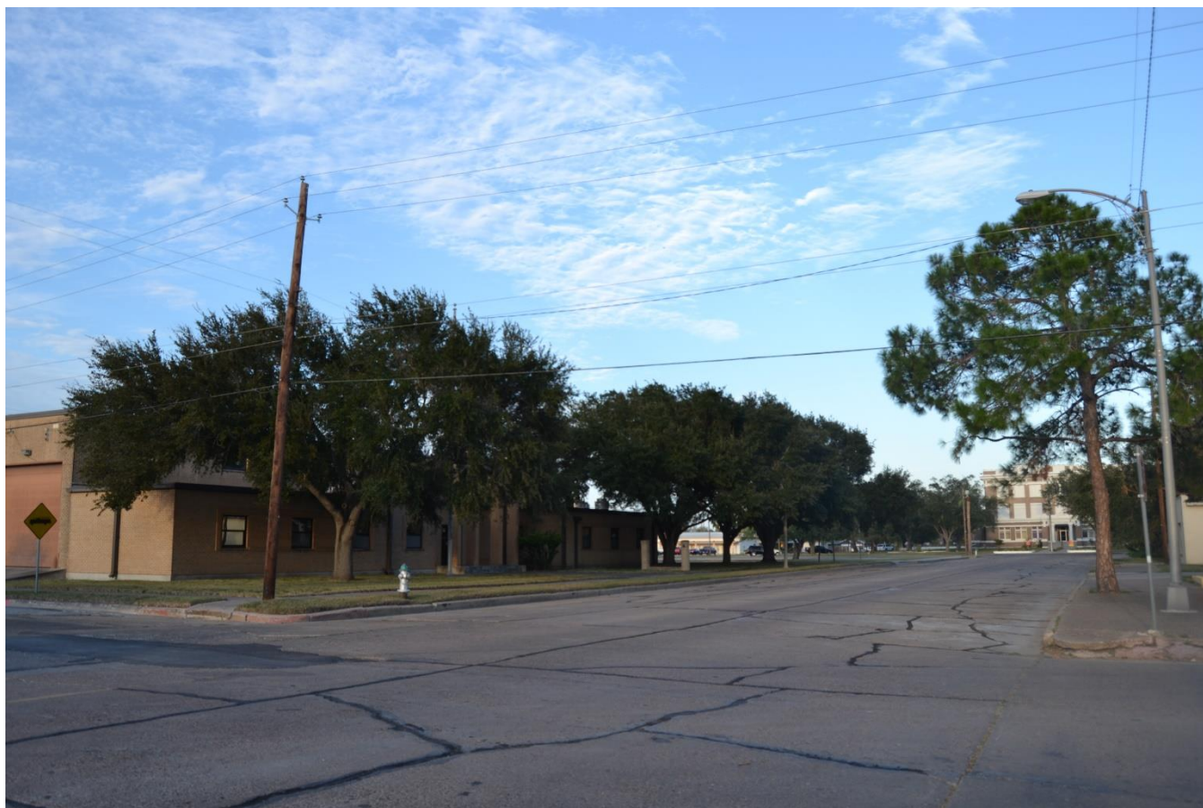
Photo No. 24 (TX_KlebergCounty_KingsvilleDowntownHistoricDistrict_0024) Resource No. 57, 604 East Kleberg Avenue, oblique view of the National Guard Armory Building, view facing northeast.
