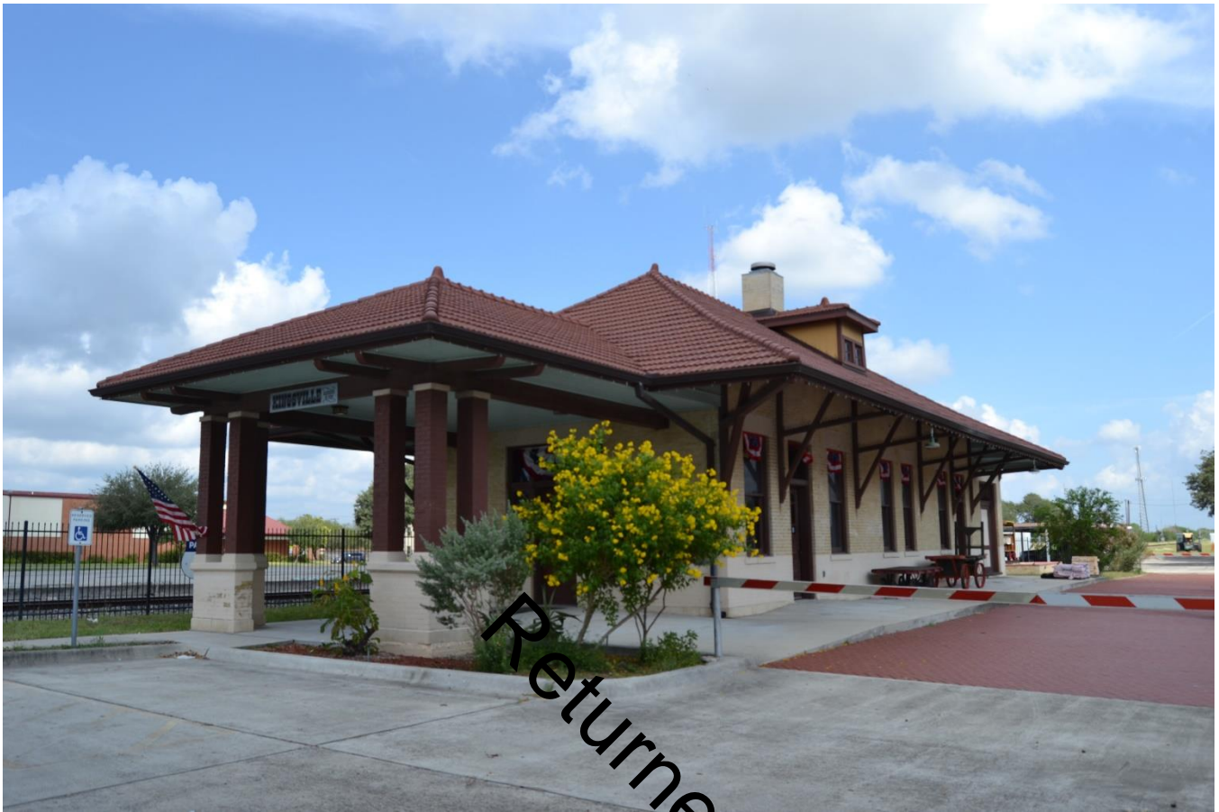
Photo No. 11 (TX_KlebergCounty_KingsvilleDowntownHistoricDistrict_0011) Resource No. 2, 100 West Kleberg Avenue, oblique view of St. Louis, Brownsville & Mexico Railroad Depot, view facing northwest.
