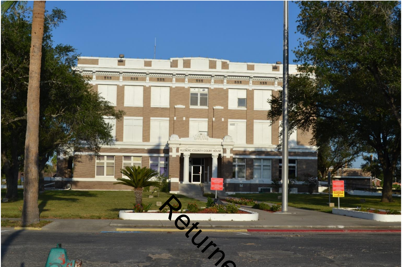
Photo No. 22 (TX_KlebergCounty_KingsvilleDowntownHistoricDistrict_0022) Resource No. 62, 700 East Kleberg Avenue, façade of Kleberg County Courthouse, view facing east.
