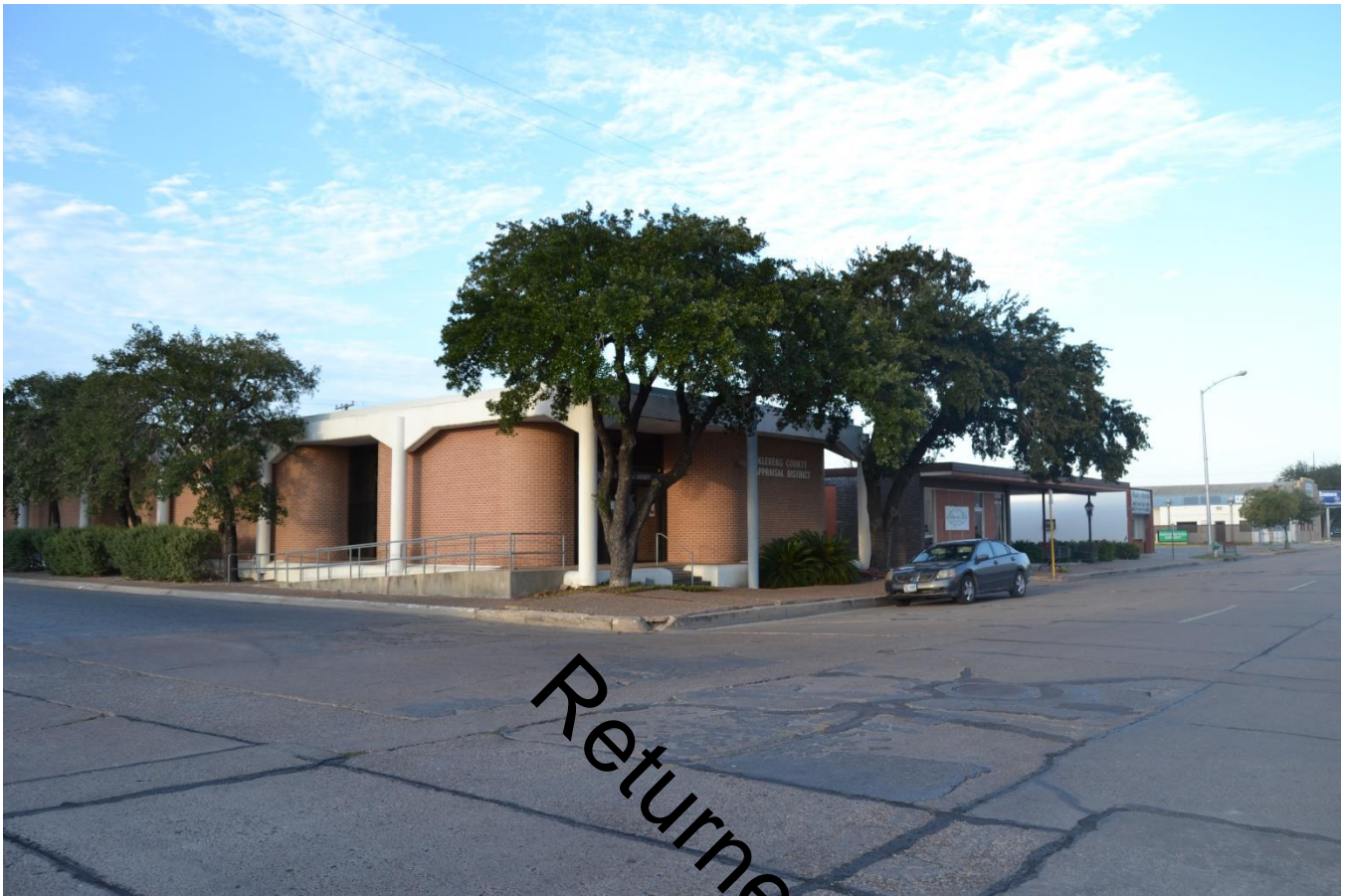
Photo No. 25 (TX_KlebergCounty_KingsvilleDowntownHistoricDistrict_0025) Resource No. 51, 502 East Kleberg Avenue, oblique view of the Kleberg County Abstract Company Building, view facing northeast.
