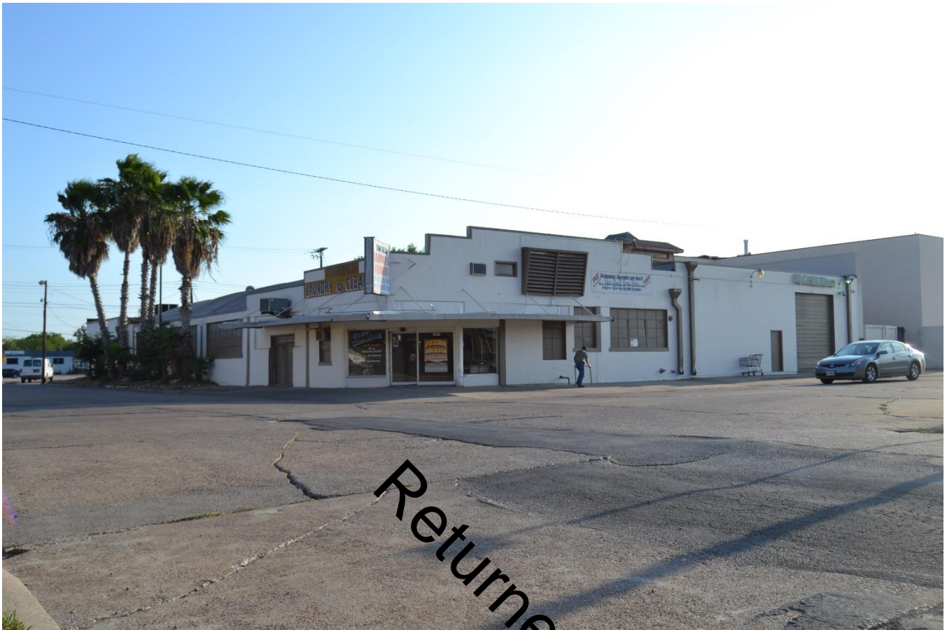
Photo No. 21 (TX_KlebergCounty_KingsvilleDowntownHistoricDistrict_0021) Resource No. 56, 529 East Kleberg Avenue, oblique view of the Kingsville Laundry and Cleaners Building, view facing southwest.
