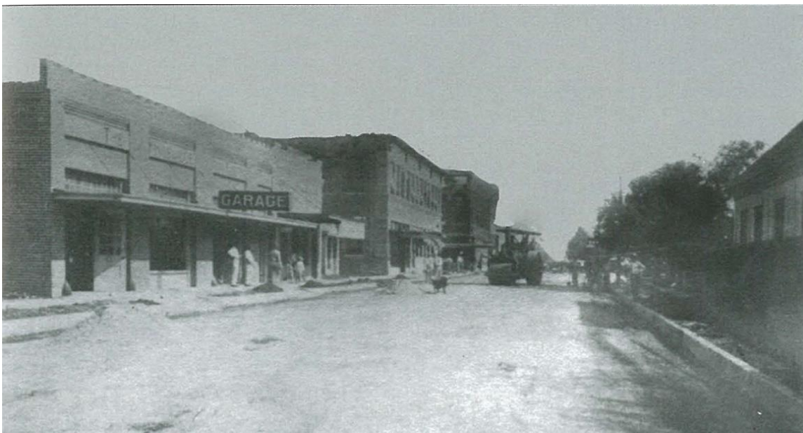
View of North 6th Street (north of East Kleberg Avenue) during paving in 1919. Depicted from left to right are an auto garage (demolished before 1962), Robert J. Kleberg and Company bank buildings, and Ragland's Mercantile. Source: Kingsville, crediting South Texas Archives, Texas A&M University-Kingsville.
