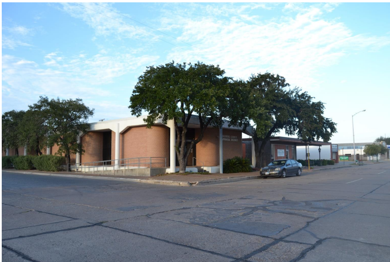
Photo No. 25 (TX_KlebergCounty_KingsvilleDowntownHistoricDistrict_0025) Resource No. 51, 502 East Kleberg Avenue, oblique view of the Kleberg County Abstract Company Building, view facing northeast.
