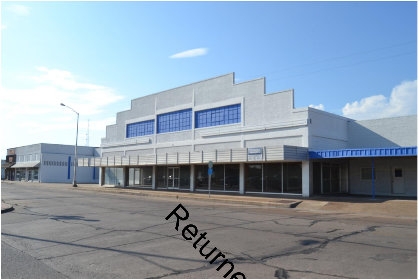
Photo No. 19 (TX_KlebergCounty_KingsvilleDowntownHistoricDistrict_0019) Resource No. 50, 410–428 East Kleberg Avenue, oblique view of the Gulf Coast Motor Company/K.A. Childs Motors – Ford Dealership, view facing northwest.
