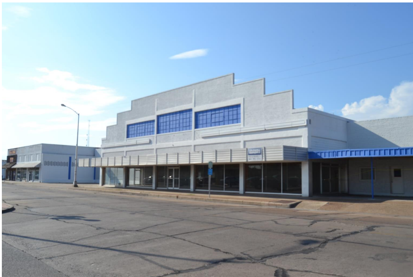
Photo No. 19 (TX_KlebergCounty_KingsvilleDowntownHistoricDistrict_0019) Resource No. 50, 410–428 East Kleberg Avenue, oblique view of the Gulf Coast Motor Company/K.A. Childs Motors – Ford Dealership, view facing northwest.
