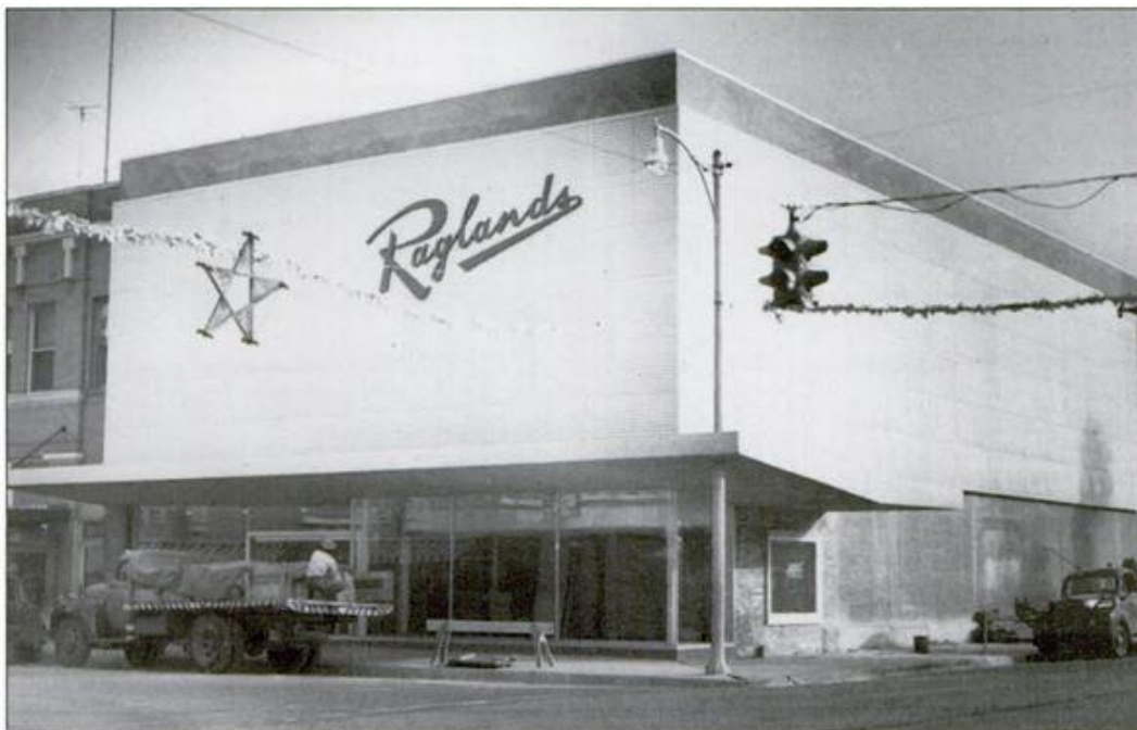
View of Ragland's Department store after the store's remodeling. July 1950. Source: Kingsville, crediting King Ranch, Inc., Kingsville, Texas
