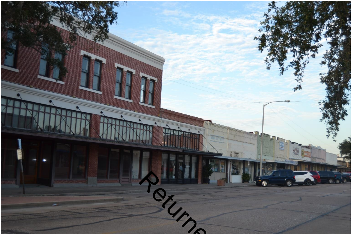
Photo No. 8 (TX_KlebergCounty_KingsvilleDowntownHistoricDistrict_0008) Contextual view of district from 300 block of Kleberg Avenue, view facing northeast.
