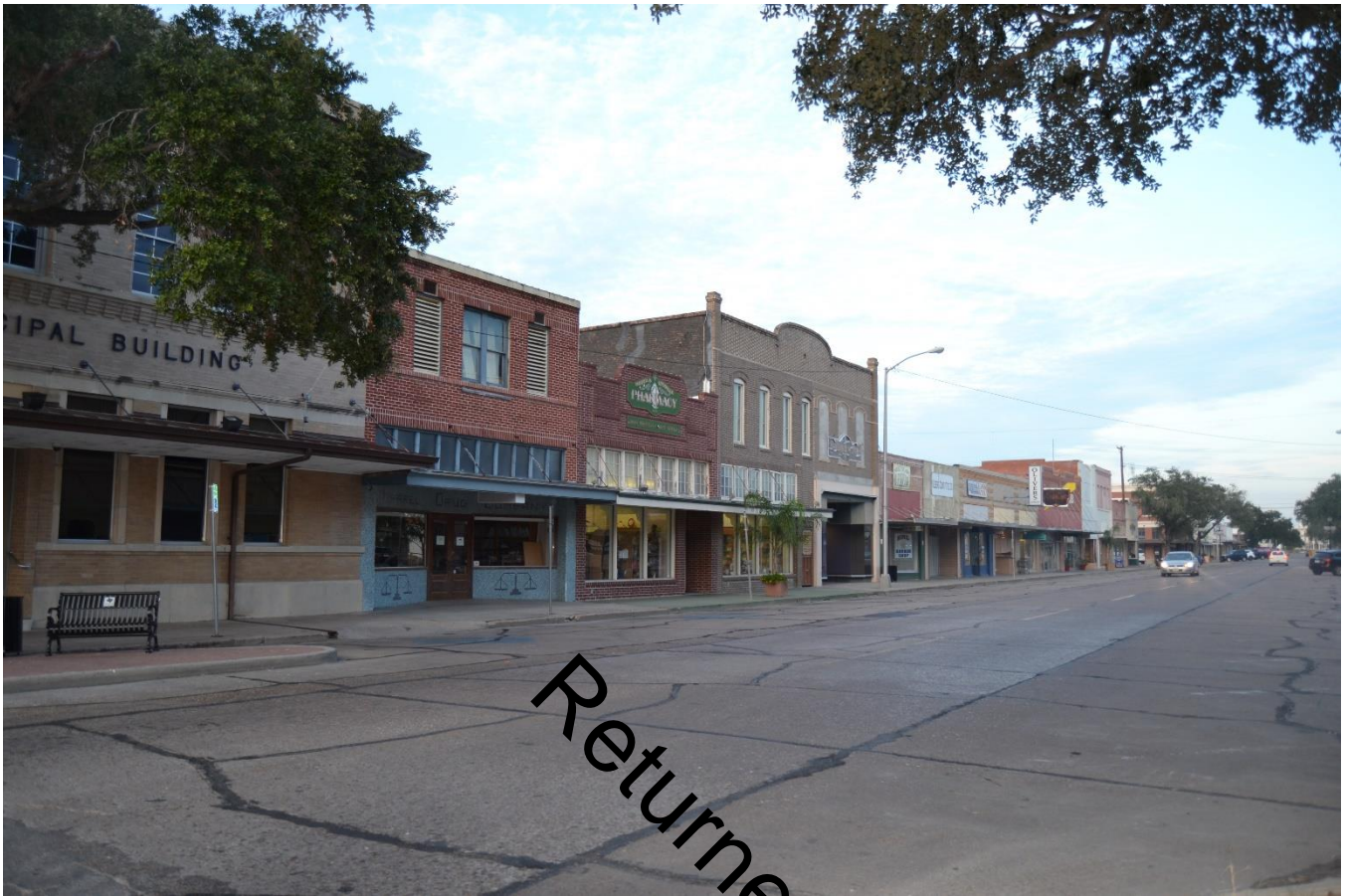
Photo No. 3 (TX_KlebergCounty_KingsvilleDowntownHistoricDistrict_0003) Contextual view of district from 200 block of Kleberg Avenue, view facing northeast.
