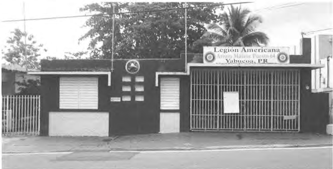
FIG. 3: Yabucoa Fire Station northwest elevations, looking southeast, in Yabucoa, Puerto Rico. The piece of land occupied by the fire station is located on #22 Muñoz Rivera Street. The Municipality of Yabucoa owns the former firehouse, but in the late 1990's it was granted custody of it to the American Legion Department of Puerto Rico – Arturo Malave Post 64 , which holds meetings and events on the premises. Photo: Guillermo Marrero, September 10, 2011.
