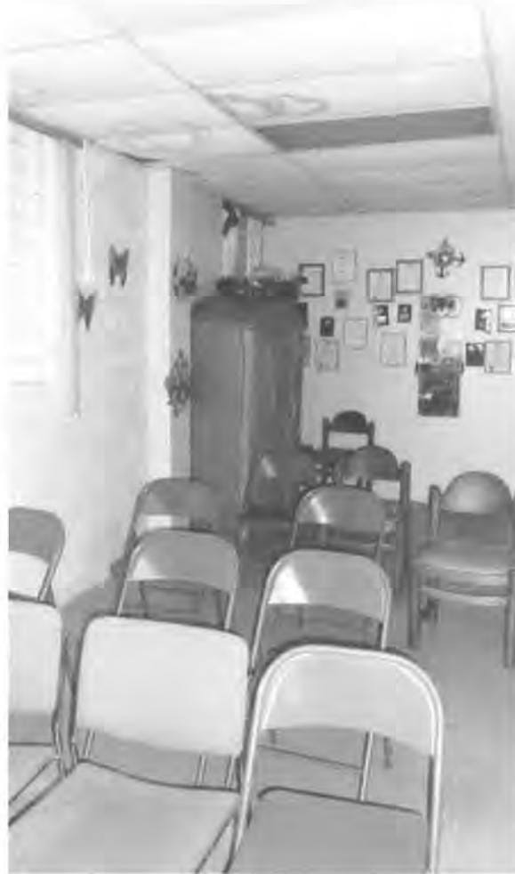
FIG. 7: Yabucoa Fire Station south elevations, looking north, in Yabucoa, Puerto Rico. The original fire truck garage is utilized for meetings, portions of the walls are painted and not covered; a door has been added to provide an additional means of egress from the room. Photo: Guillermo Marrero, June 10, 2012.
