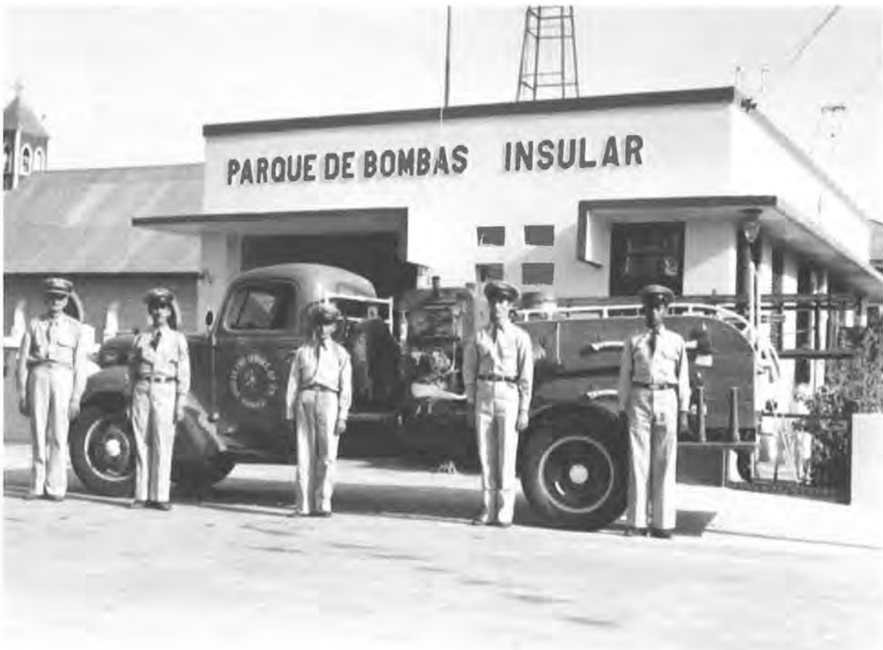
FIG. 1: Guanica Fire Station in Guanica, Puerto Rico. Similar to the Yabucoa Fire Station. Prototype B was the one chosen for Yabucoa; the original, basic plans consisted of a single story, asymmetrical model with a flat roof, yet open space for one truck, measuring 34'-6" x 22'-0". An entrance door to its right completed the main façade. Six small, square-shaped openings in this main elevation provided light for its interior spaces through glass panes or glass block, as well as an articulation of the otherwise plain concrete wall. Horizontal eaves (sometimes curving down) and roof parapets with rounded edges reverberate traces of the Art Deco style. Some of these structures include a flagpole in iron piping. The name " Parque de Bombas " is often featured in bas-relief concrete at the parapet over the truck opening. Source: Gobierno de Puerto Rico Servicio Insular de Bomberos de Puerto Rico, Informe Annual 1945-1946. Publicacion del Servicio Insular de Bomberos.
