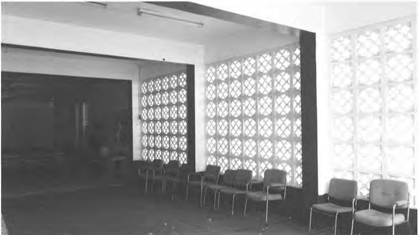
FIG. 5: Yabucoa Fire Station interior east elevation, looking east, in Yabucoa, Puerto Rico. The southwest elevation is composed by a three bay ornamental cement blocks walls that encloses the 1970's expansion. Built over an eighteen inch (18") low parapet, the fourteen inch (14") squared decorative blocks are laid out in a six high by a seven wide grid. Photo: Guillermo Marrero, June 10, 2012.
