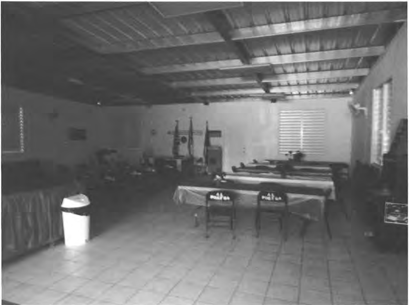
FIG. 8: Yabucoa Fire Station interior view looking southeast, in Yabucoa, Puerto Rico. Towards the back of the lot, a second addition was made after 2006 to provide for a larger enclosed meeting area. Surpassing 1,000 ft 2 , the room provides enough space for all types of protocolary activities, social and commemorative events. Photo: Guillermo Marrero, June 10, 2012.
