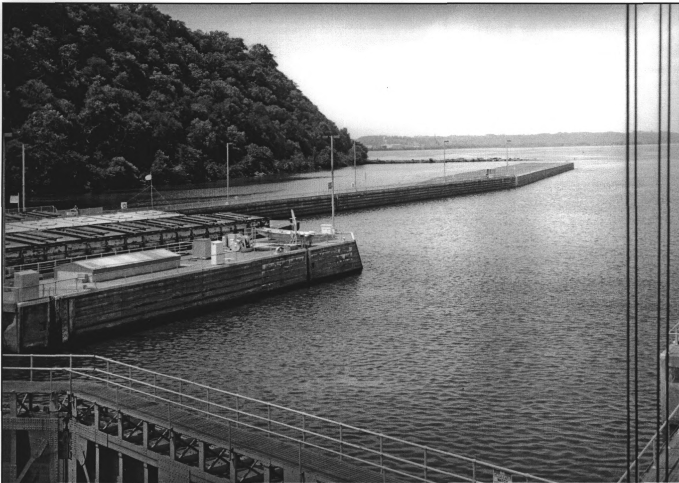
PHOTO 4. Upstream Guide Wall Extensions, Deflecting Dike, and Slough Impoundment.
