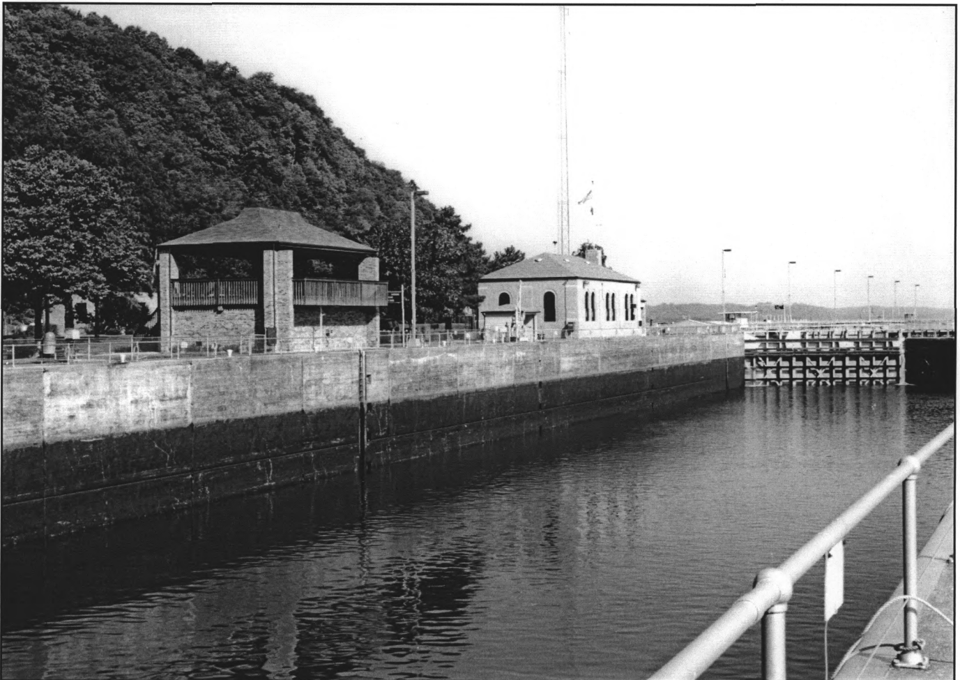
PHOTO 6. Lock Chamber in Foreground, Visitor Center at Left, Scooter Shed, Central Control Station, Upstream Face of Downstream Lock Gates at Right.
