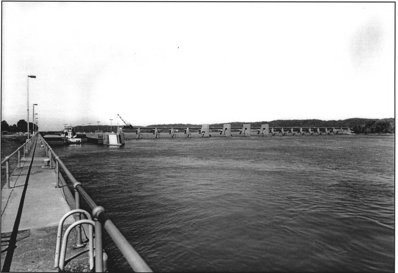
PHOTO 3. General View of Dam, Downstream Side.
