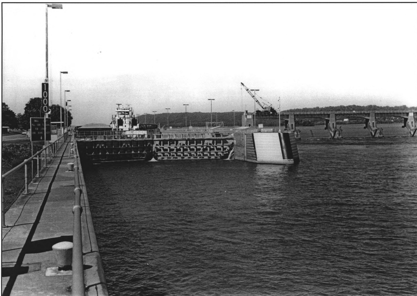
PHOTO 2. General View of Lock, Downstream Side.
