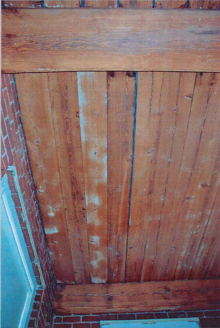
21. View east, unit ceiling detail revealing exposed wood decking (Feb. 2018).
