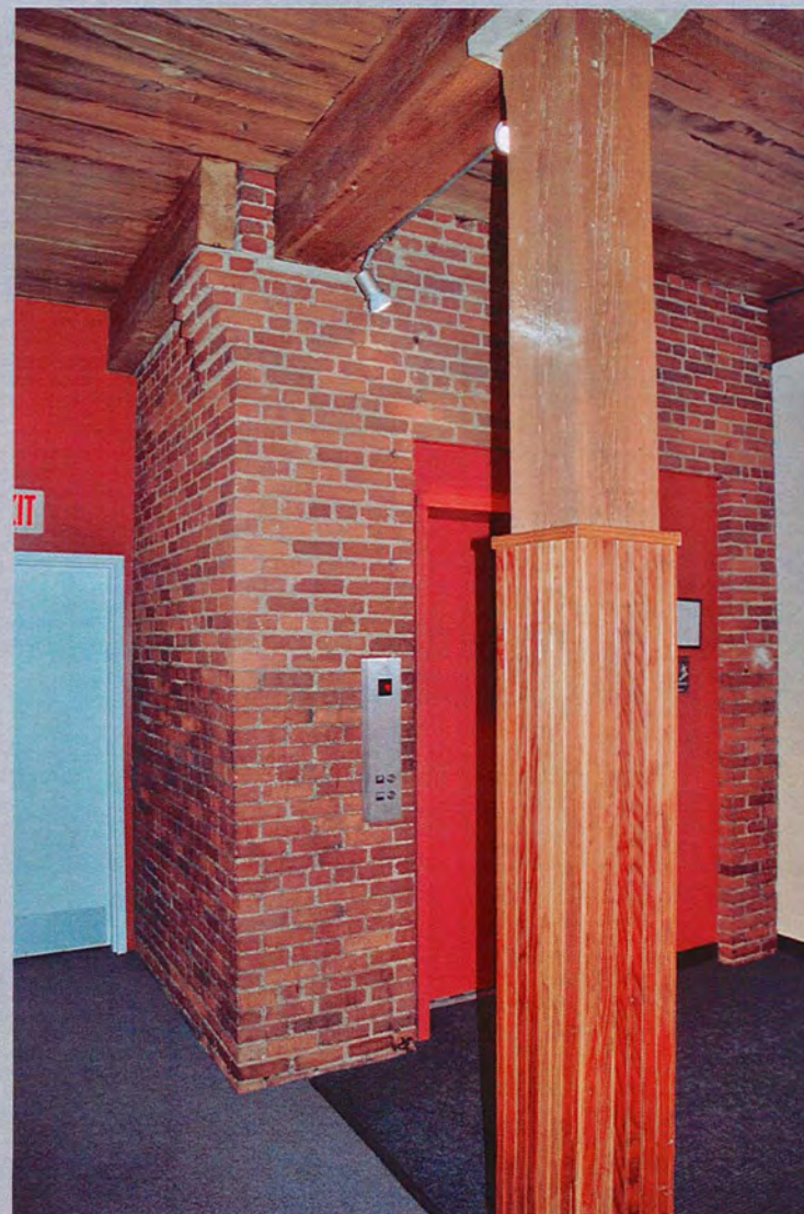
14. View northeast, fourth floor, original brick-enclosed freight elevator that was repurposed in 1976 as pedestrian elevator; brick shaft features corbelled upper corners and load-bearing beams set into the walls (Feb. 2018).
