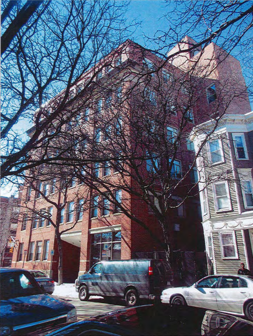
7. View southwest towards the George Close Company Building (Feb. 2017).
