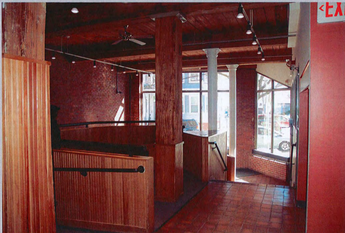
10. View east of lobby showing exposed brick walls, square wood and circular concrete columns and decking (Feb. 2018).
