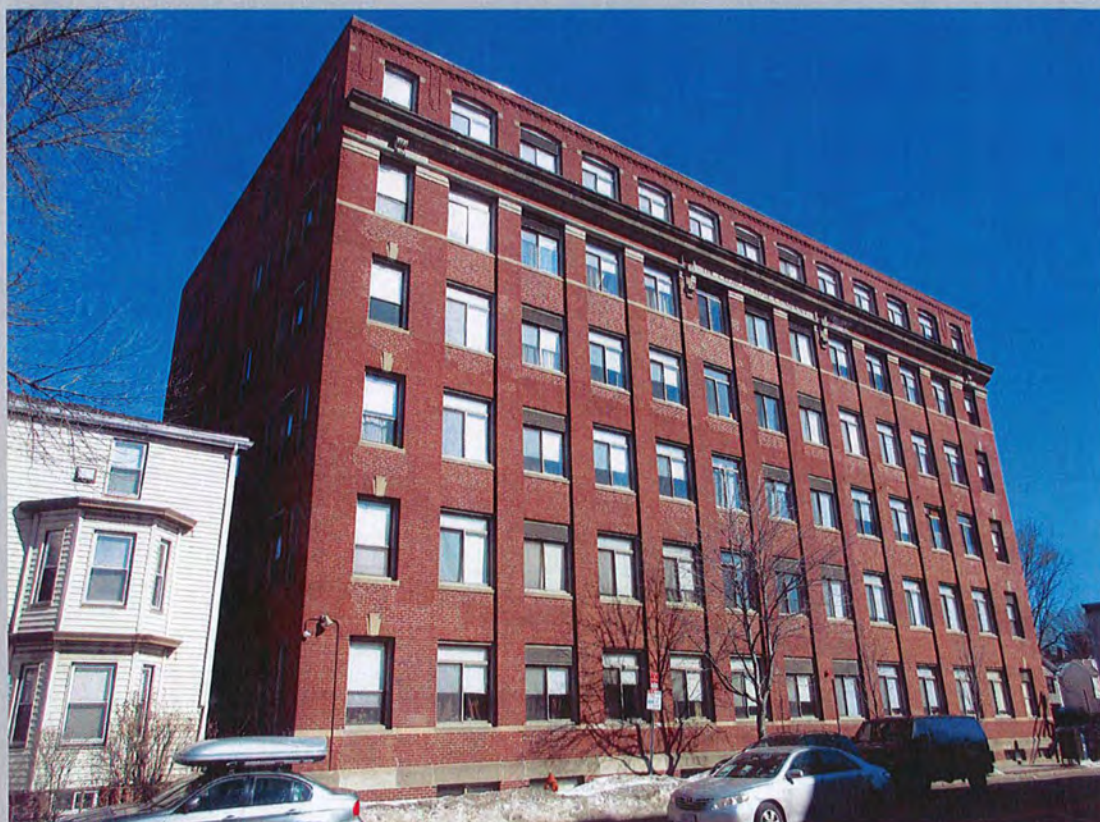
2. View northeast towards the George Close Company Building (Feb. 2017)
