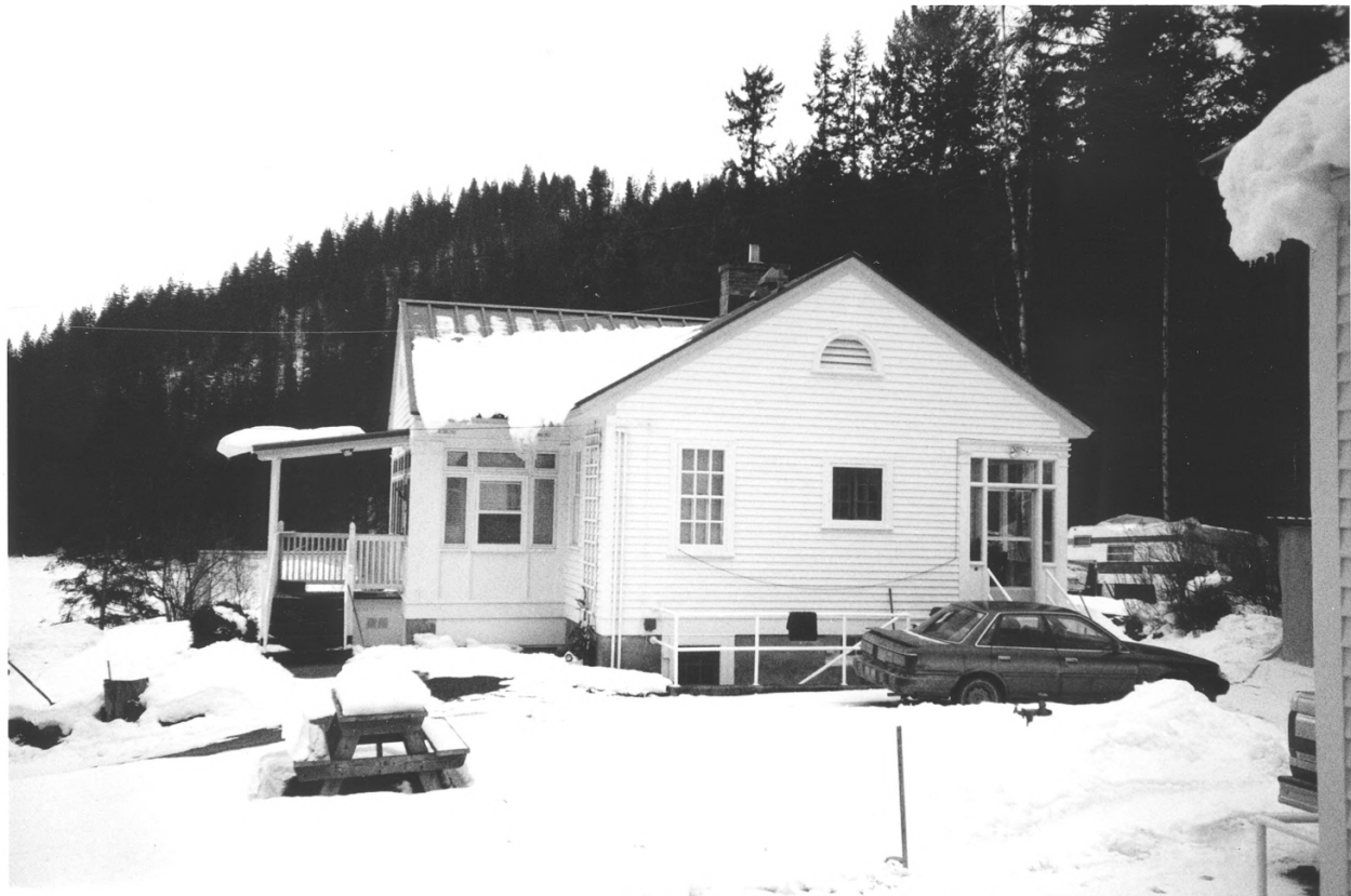
METALINE FALL BORDER STATION, METALINE FALLS, PEND OREILLE COUNTY, WA. PHOTO NO 8.
