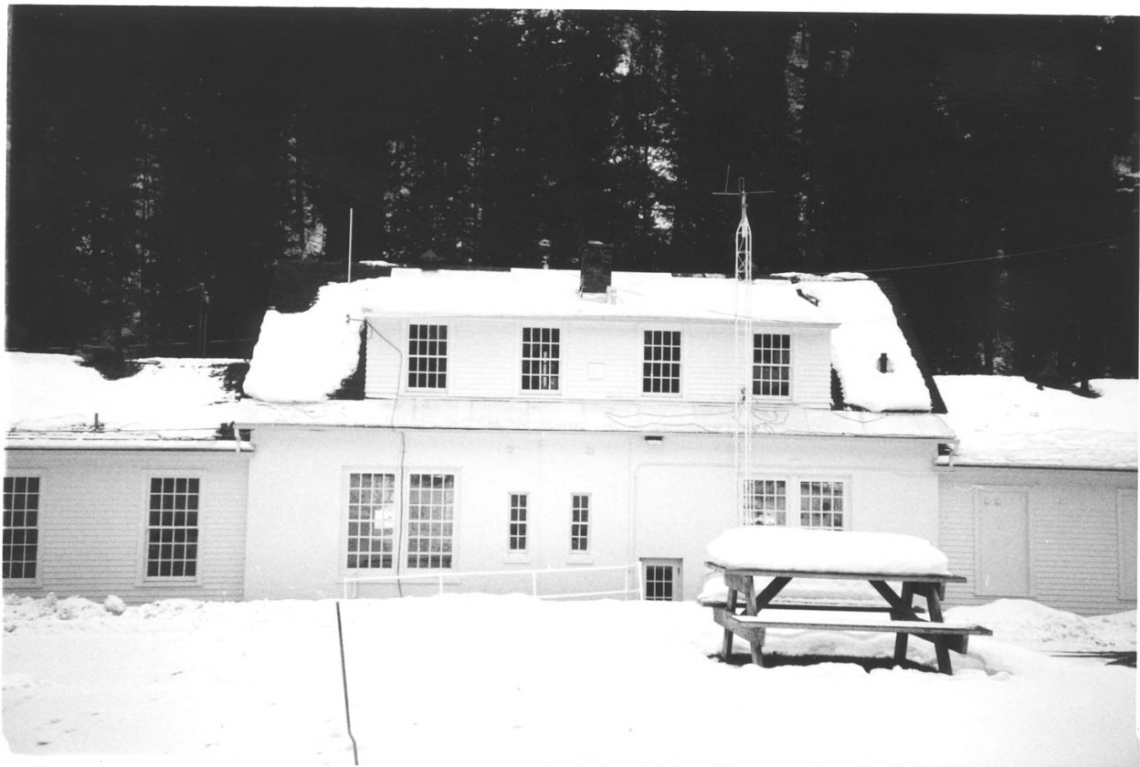
METALINE FALLS BORDER STATION, METALINE FALLS, PEND OREILLE COUNTY, WA. PHOTO 5
