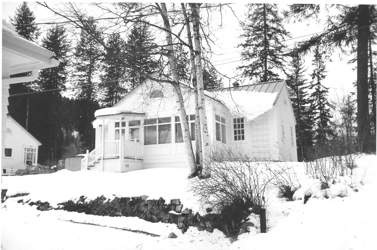
METALINE FALLS BORDER STATION, METALINE FALLS, PEND OREILLE, WA. PHOTO NO 6.
