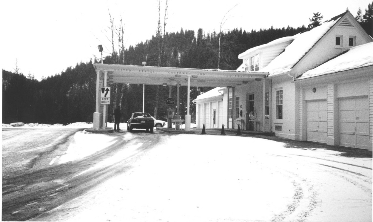
METALINE FALLS BORDER STATION, METALINE FALLS, PEND OREILLE COUNTY, WA. PHOTO NO. 2.
