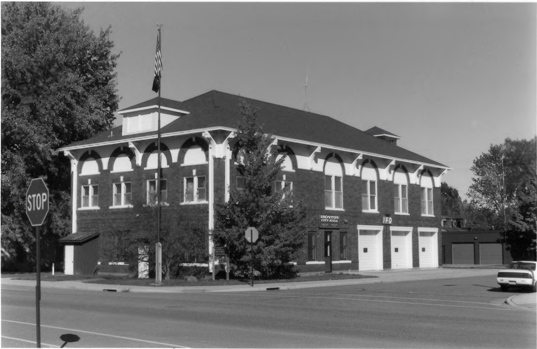
Ironton City Hall Crow Wing Co., Mn 014235 - 20A/21
