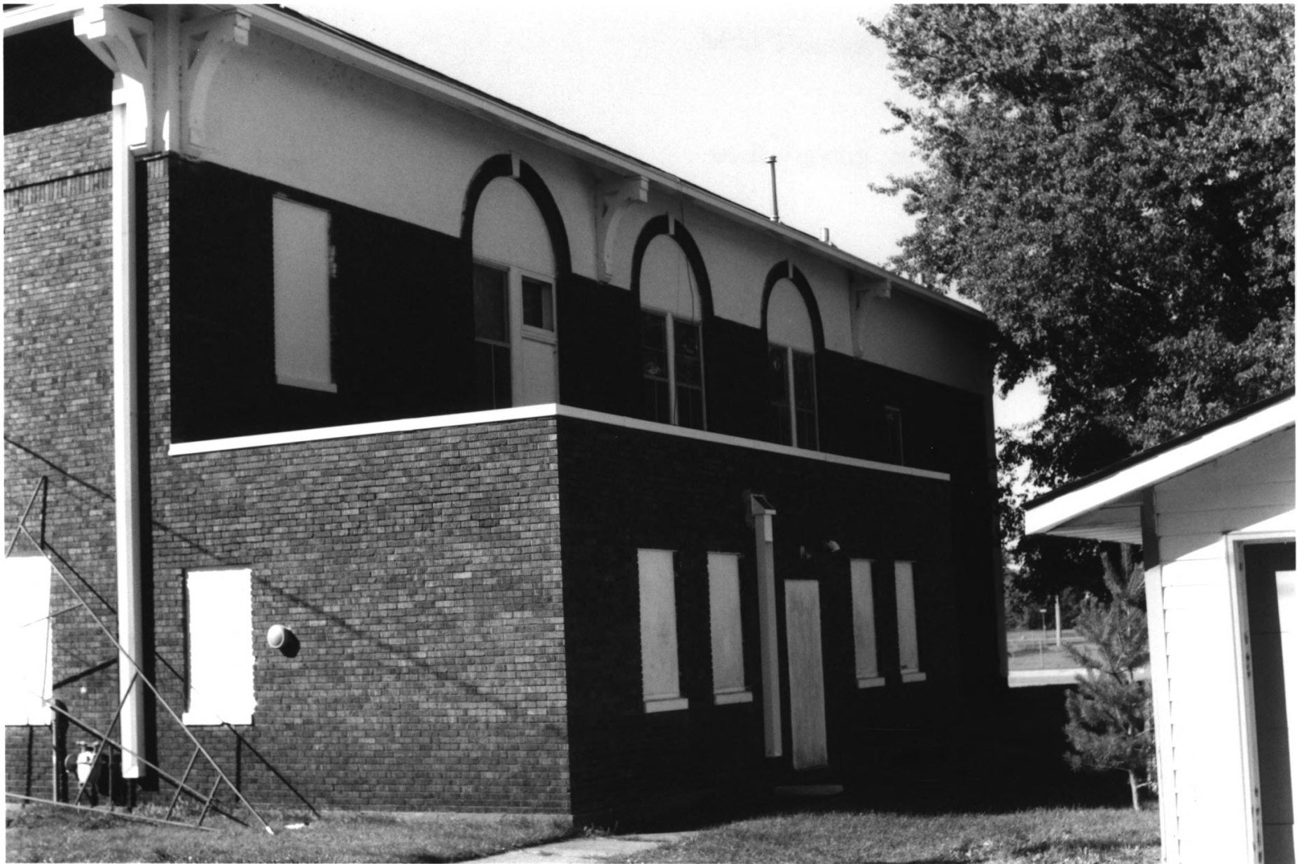
IRONTON CITY HALL CROW WING CO., MN 014235-6
